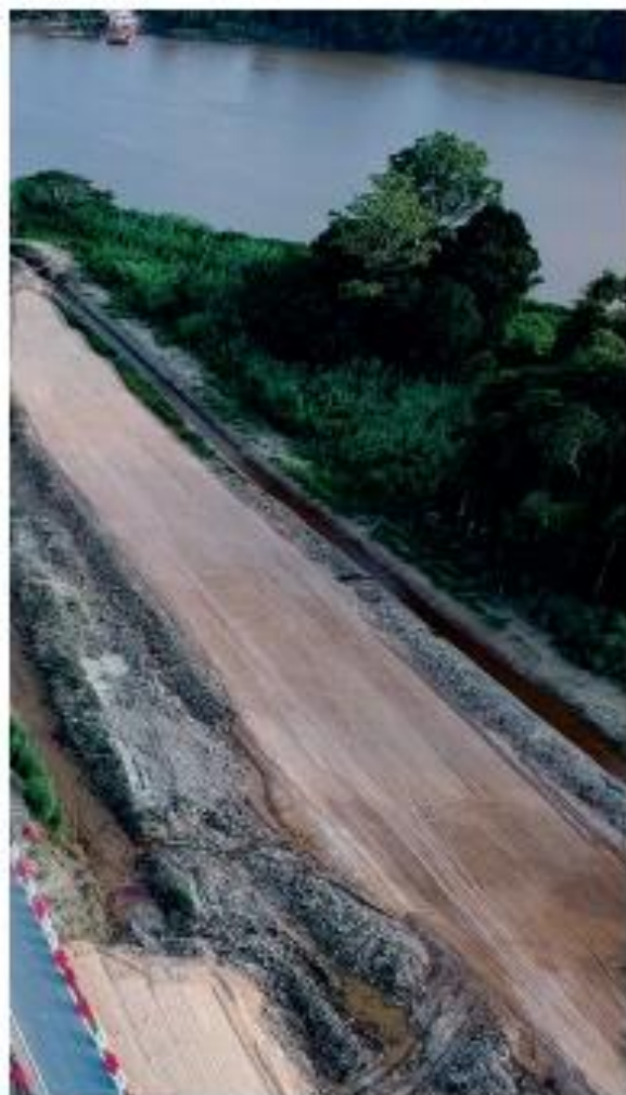
Construction of Marudi Bridge, costing over RM75 million is progressing well and is expected to be completed in early 2023.
