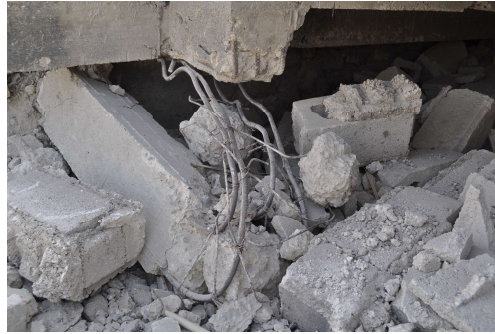
Fig. 1.1. Steel bar in the collapsed structures at the UNIH University in Haiti earthquake (Eberhard et al., 2010).
