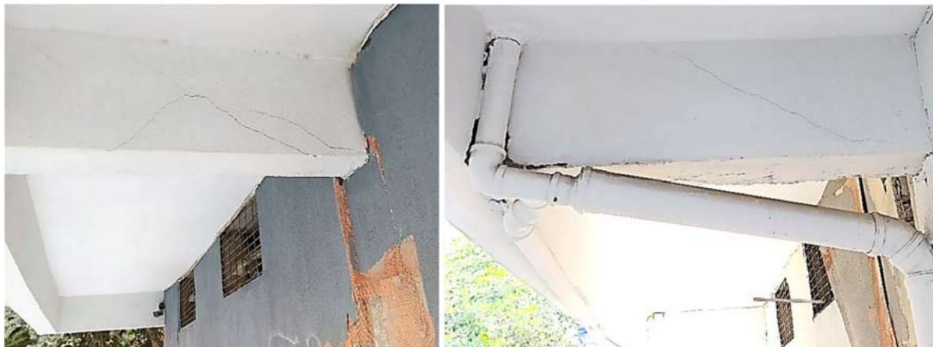
Fig. 1.2. Overhang damages in Samos Island Earthquake (Çetin et al., 2020).
