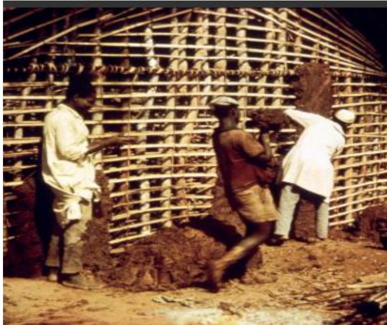
Figure 2-6: Wattle and daub building construction
