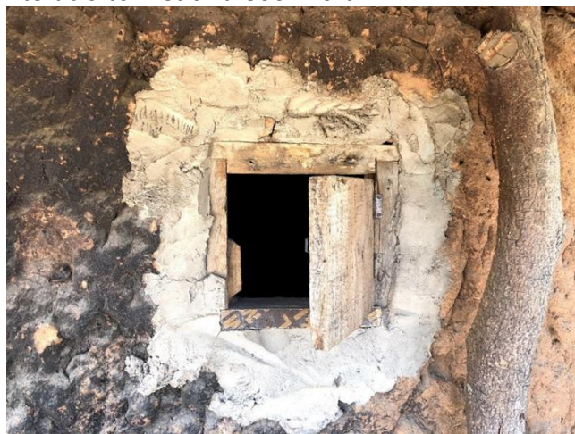
Figure 5-20: Picture illustrating the tiny window (600mm by 600mm) on a typical Ilorin adobe traditional building.
