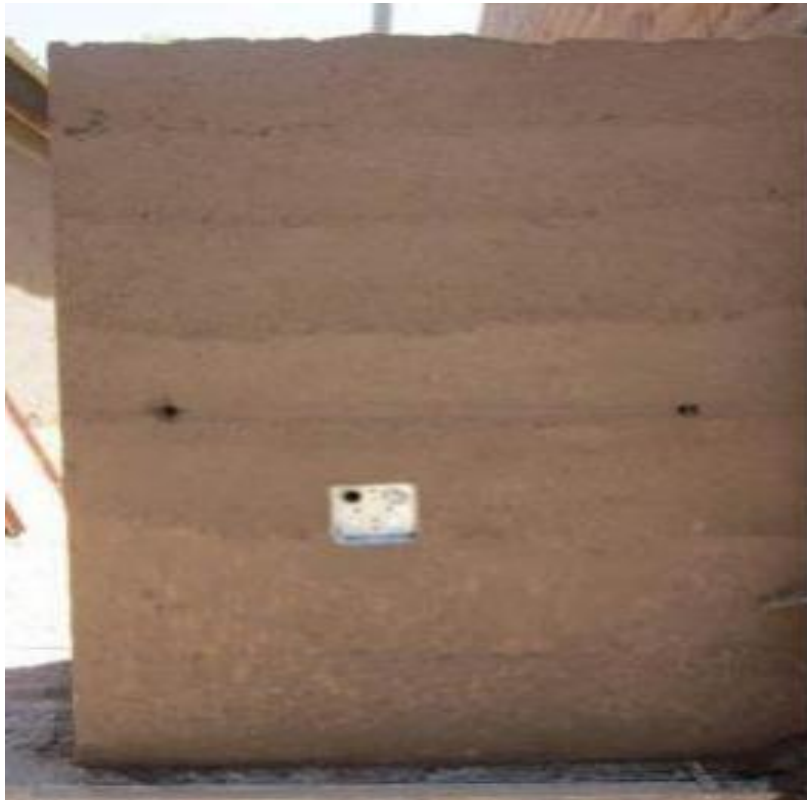
Figure 2-4: Wall made from rammed earth.
