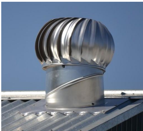
Figure 2.15. Exhaust rotating wind cowl installed on the roof of a building
