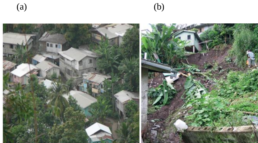
Figure 2-21 (a) Archetypal unplanned housing on unstable slopes in Castries, Saint Lucia, Eastern Caribbean; (b) Landslide on unplanned development (Holcombe et al. 2016)
