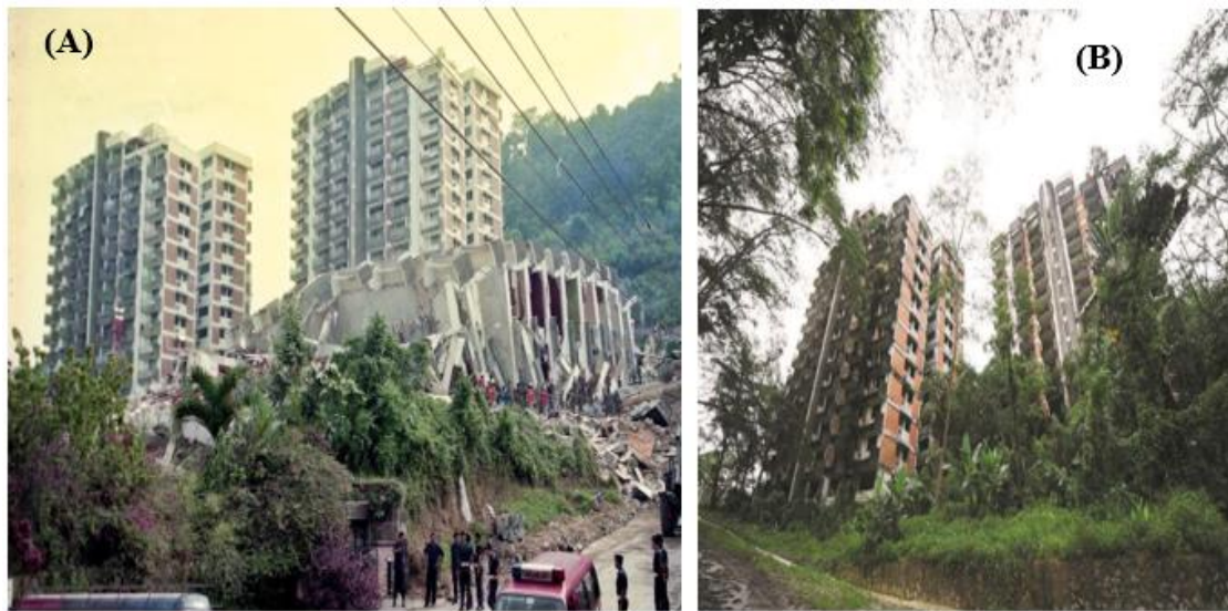
Figure 2-5 (A) Collapse of Block 1 of Highland Towers in 1993 due to catastrophic landslide (Krishnan 2023); (B) Remains of Block 2 and 3 of Highland Towers (Gul et al. 2017)
