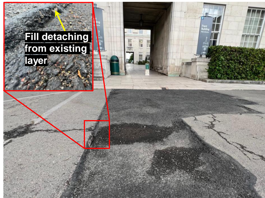
Figure 2-32: Illustration of a settled trench fill (Location: Trent Building, University Park; Date: June 27, 2022).
