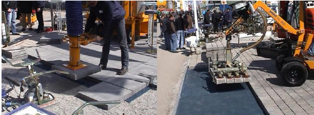
Figure 2-35: Robotic arm installing slab on site [238].
