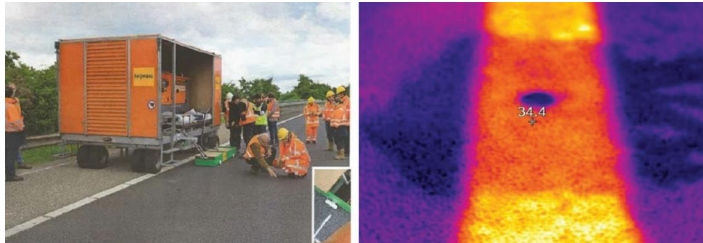
Figure 2-21: Induction heating on Dutch Highway A58 [203]
