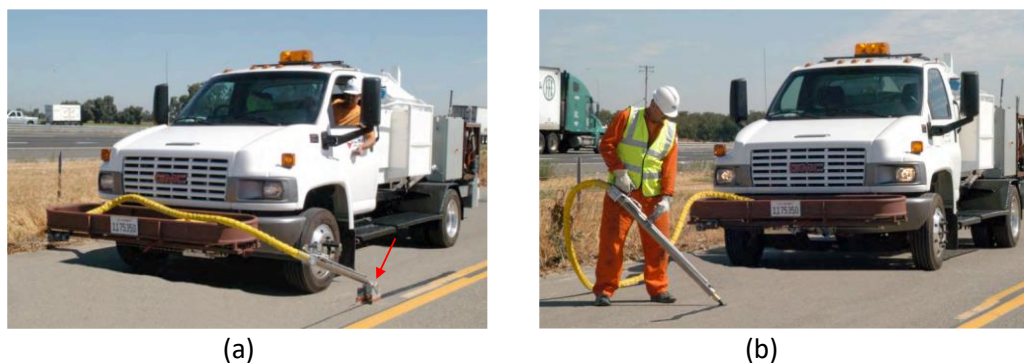
Figure 2-24: Sealzall machine: (a) during longitudinal crack sealing (b) In-lane crack sealing [17].
