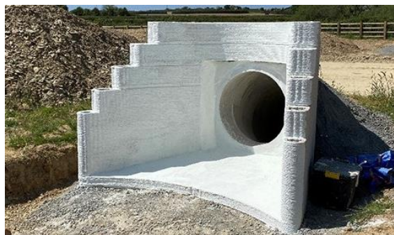
Figure 2-44: 3D printed headwall by Cambridge researchers installed on a section of the A30 road in Cornwall 19 .
