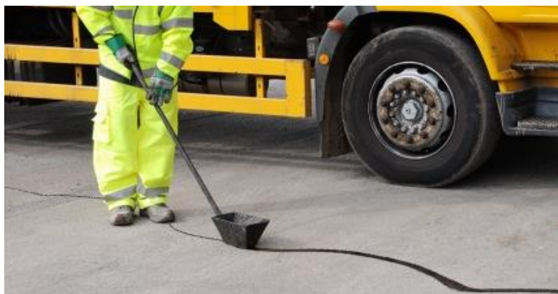
Figure 2-23: Crack filling by hand using a pour pot 10 .
