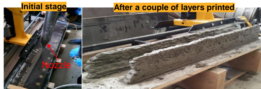
Figure 2-38: Extrusion of concrete from a 3D printing nozzle [241].
