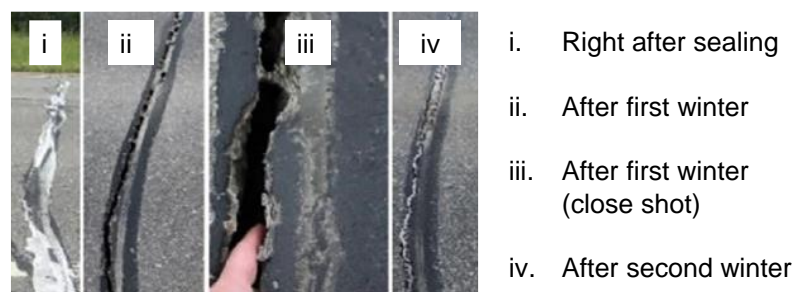
Figure 2-27: Illustration of adhesion loss in sealed cracks on site.
