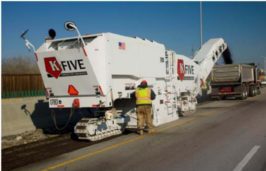
Figure 11. Milling machine removing asphalt pavement layers as part of road rehabilitation (West, 2010).
