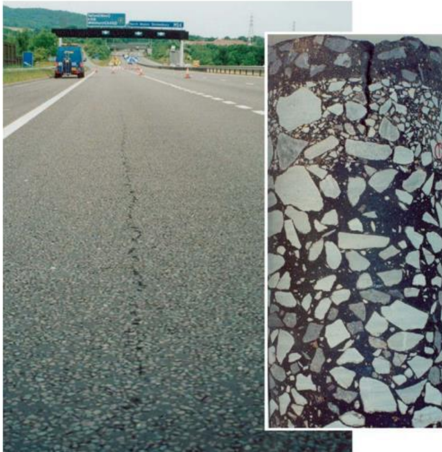
Figure 5. Longitudinal crack in a major UK motorway (Xu et al., 2015).
