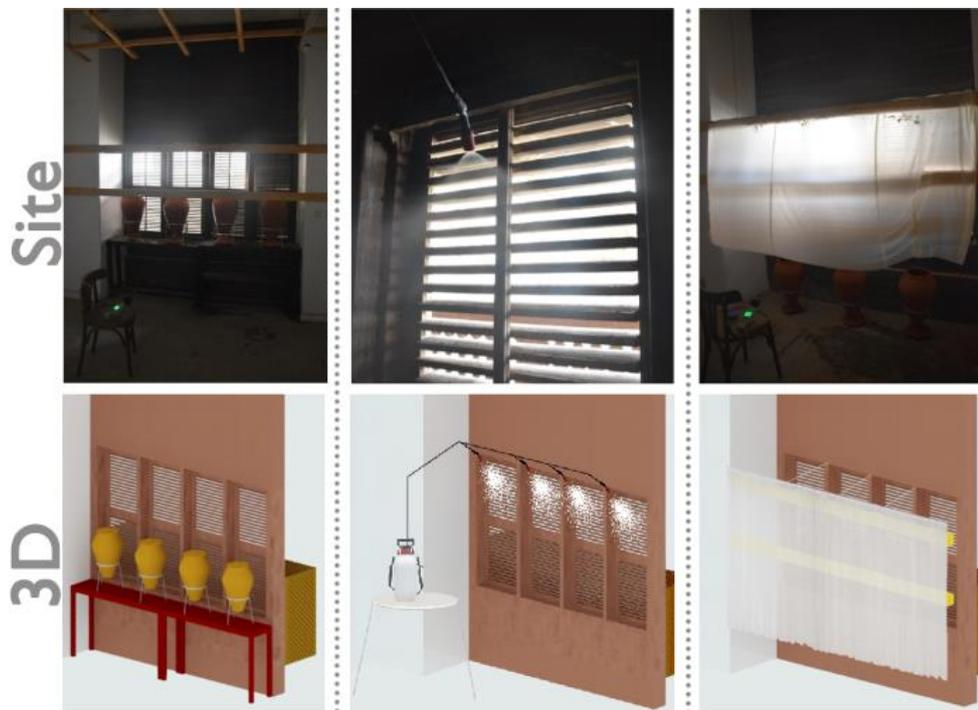
Figure 5-33 Passive evaporative cooling techniques used with the mashrabiya in R1 on the site: Pots (left), Water spray (middle) and, Cloth (right), and (below) the techniques in and 3D views
