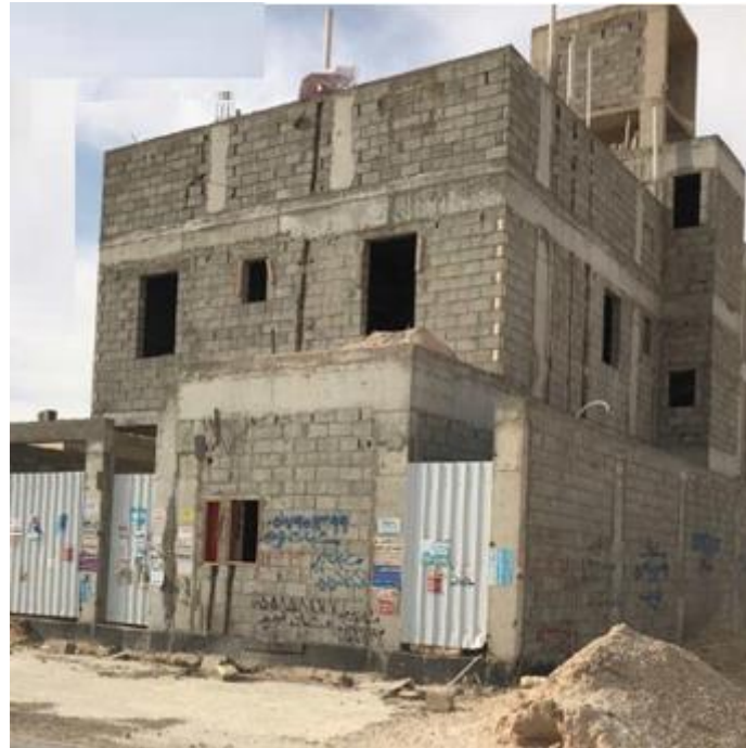
Figure 6-2: Typical envelope of a villa building under construction in KSA (Source: Khabaz, 2018)
