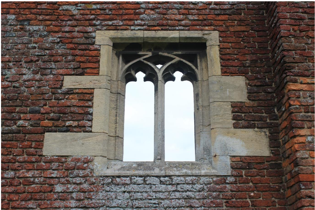
Figure 26 Window of the "Stables" with anachronistic Y-tracery
