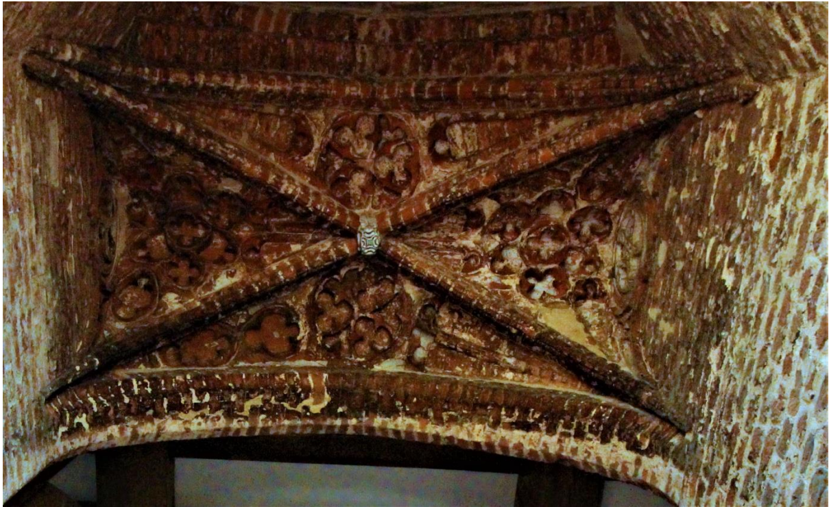
Figure 130 Vaulting of third floor chamber south-west window
