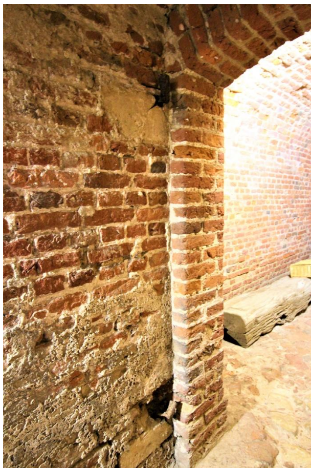
Figure 97 Pintles of the basement south-western turret doorway
