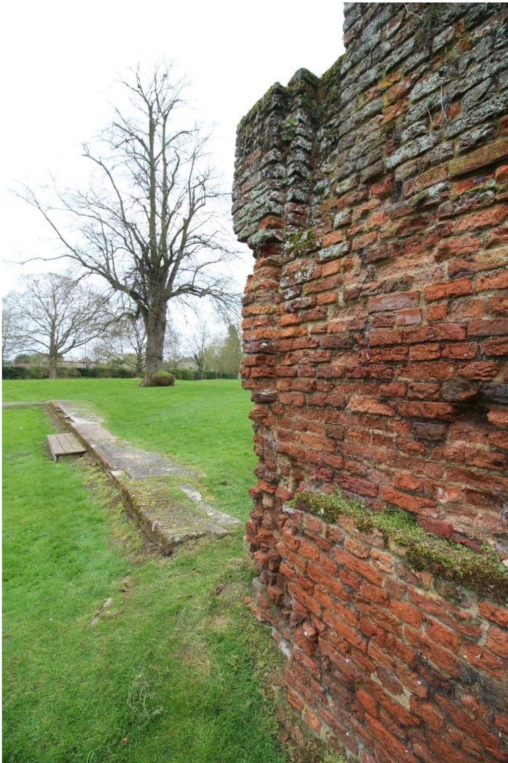
Figure 29 Stub of transverse screen wall in the east wall of the “Stables”
