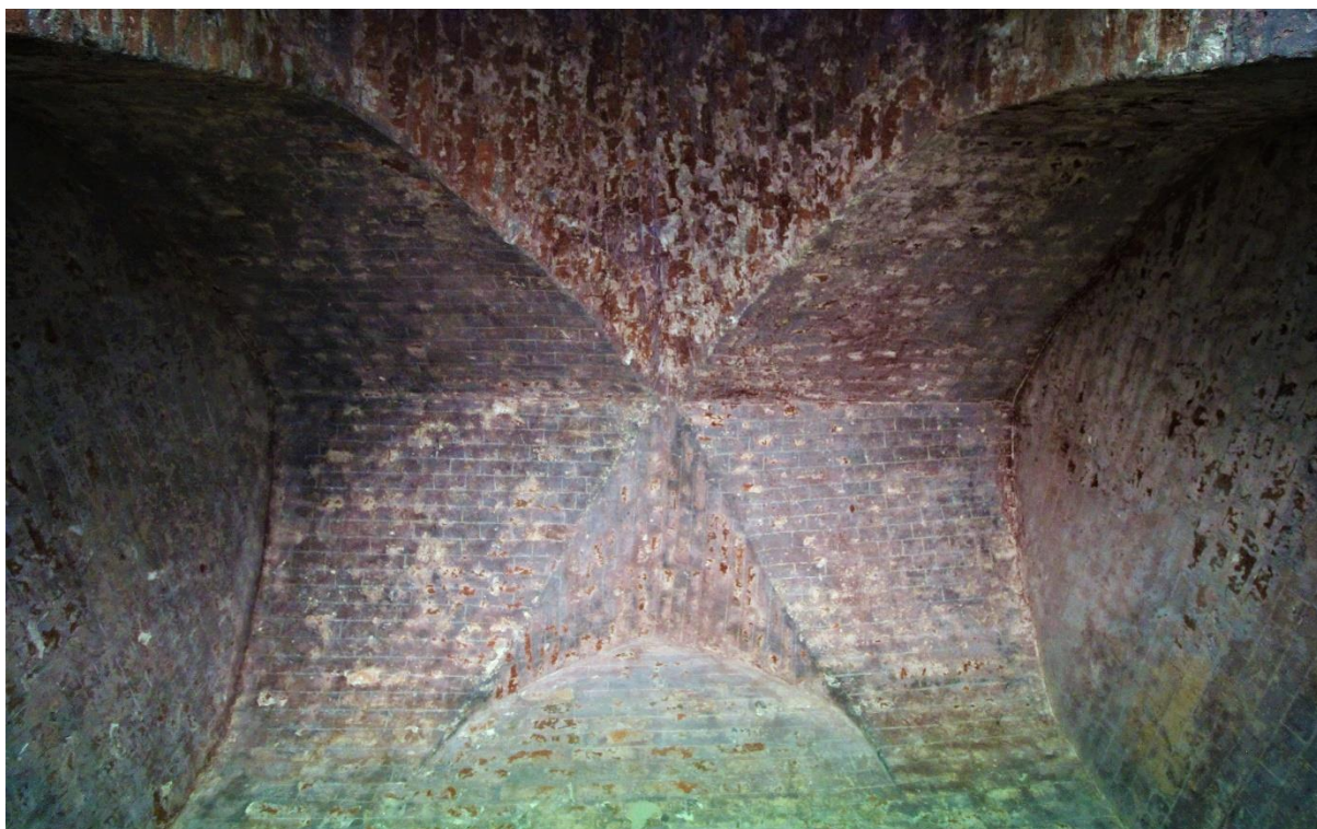
Figure 109 First floor lobby vaulting
