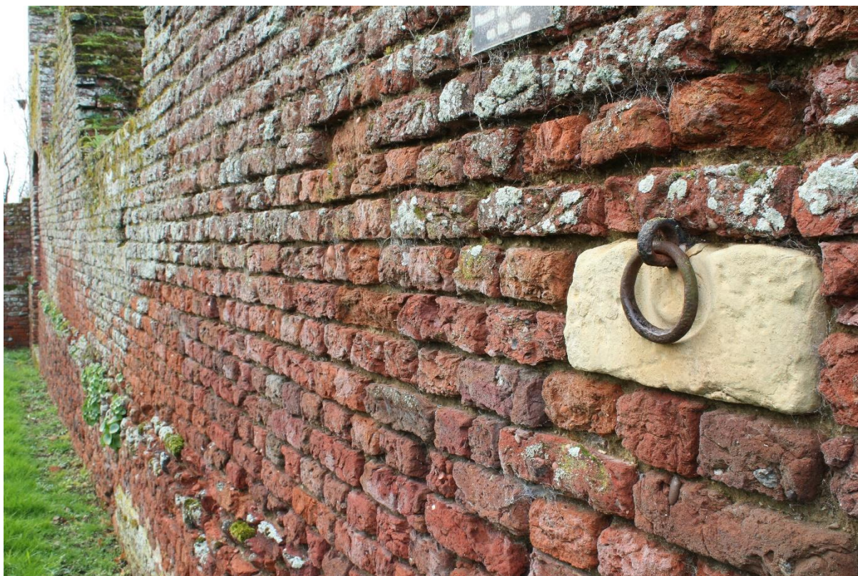
Figure 33 Possible tether ring set into the west elevation of the “Stables”
