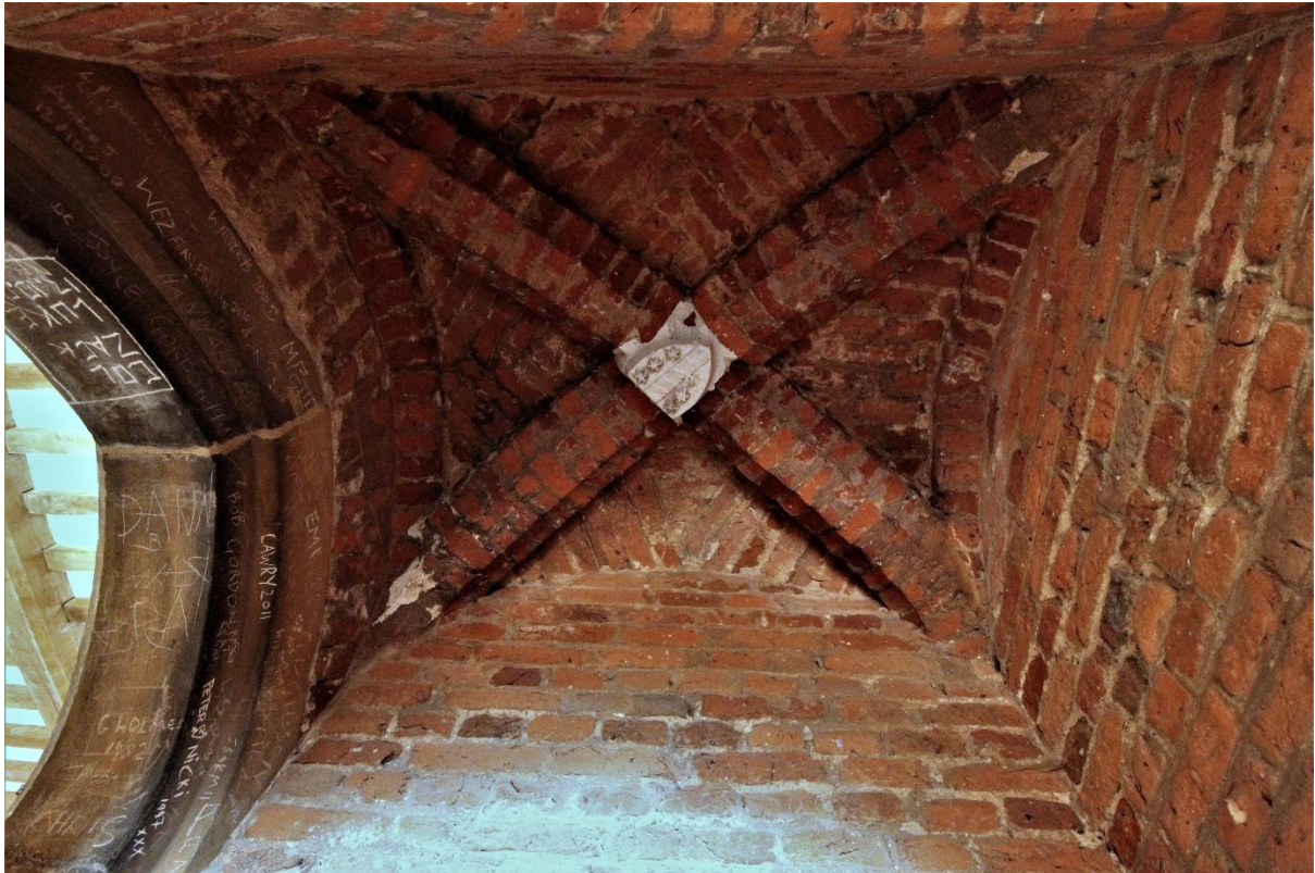
Figure 132 Vaulting to lobby of third floor south-western turret
