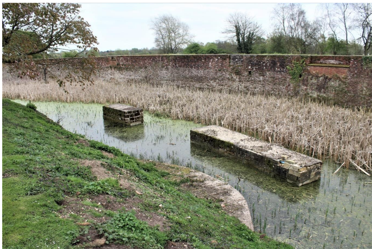
Figure 14 Thirteenth century tower foundations along the southern bank of the Inner Ward and location of the south bridge
