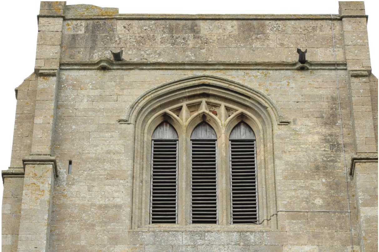
Figure 71 Uncusped window tracery of the tower of Holy Trinity Tattershall
