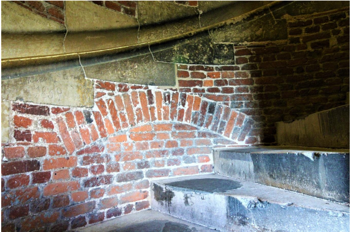
Figure 90 Staircase relieving arch
