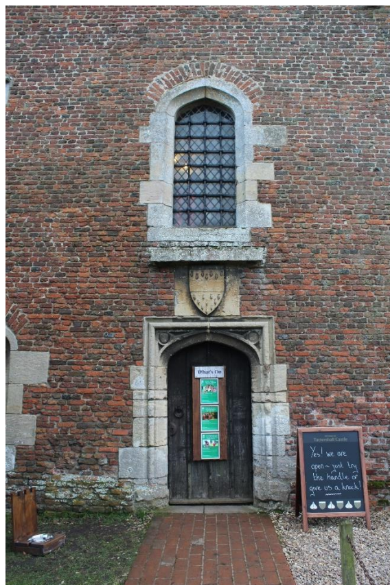
Figure 37 Inserted door (bottom), inserted Bernack armorial and carved string course (middle), former doorway (top) in the north elevation of the “Guardhouse”
