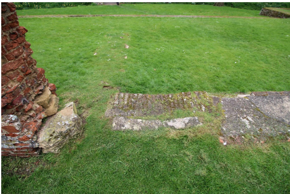
Figure 32 Moulded stone door jamb and brick threshold of the “Stables”
