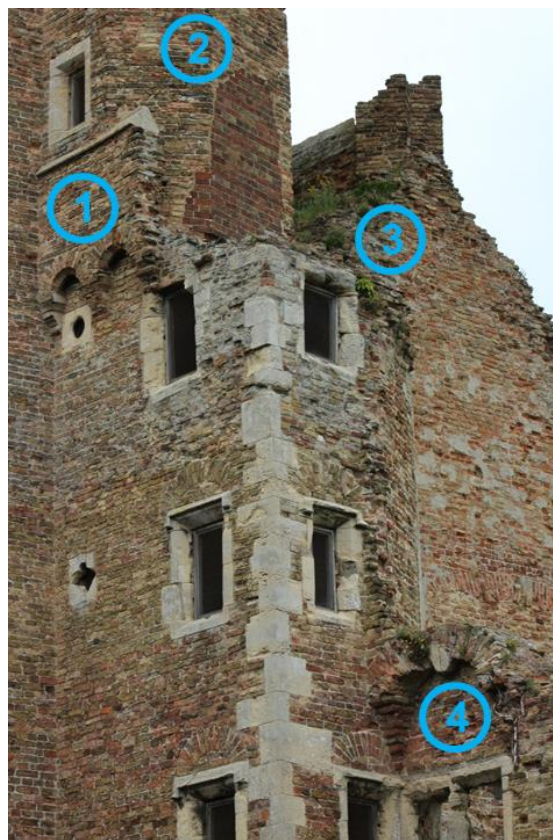
Figure 187 Detail of great hall range at Caister. Showing: 1) Crenellations and blind machicolations, 2) blocked door to parapet, 3) wall scar, 4) arcaded corbels for lower machicolations
