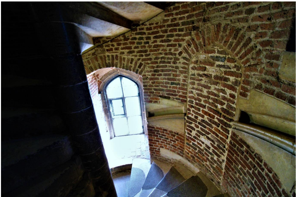
Figure 89 Former doorways between ground and first floor in the stair turret
