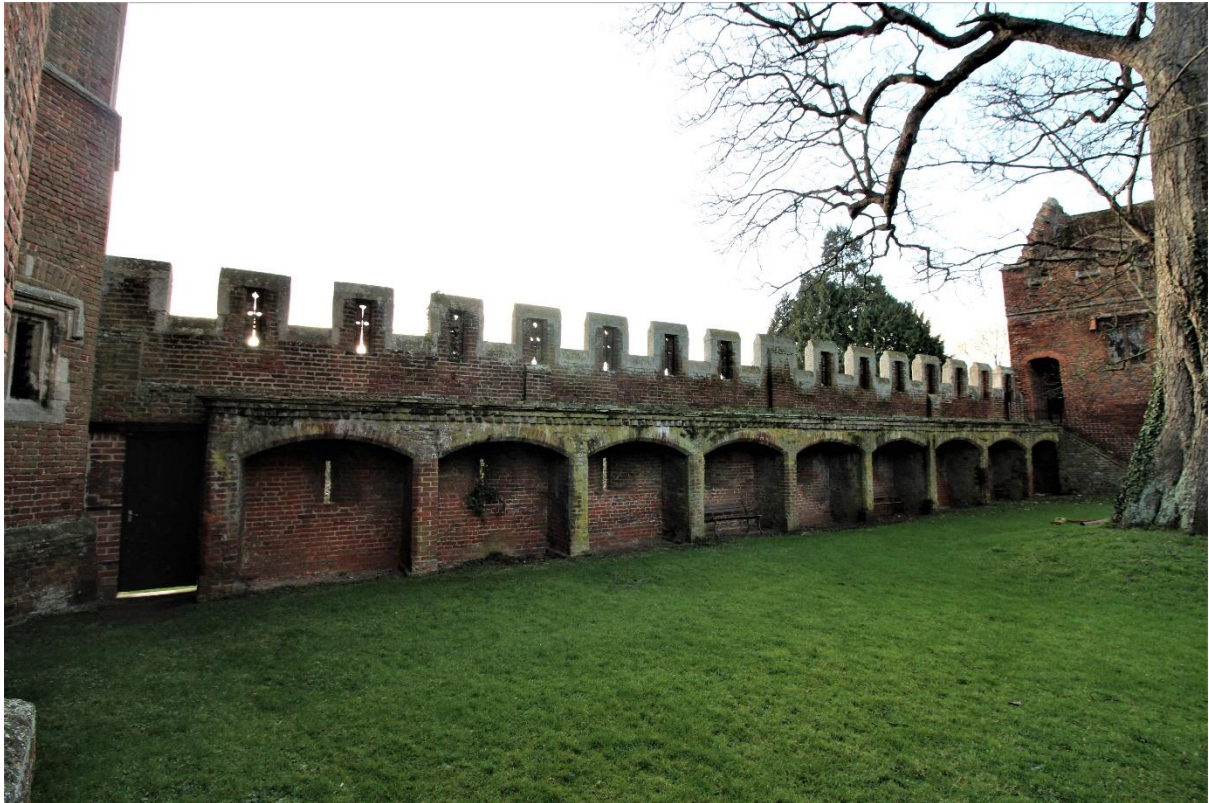
Figure 40 Arcaded inner curtain wall at Buckden Palace
