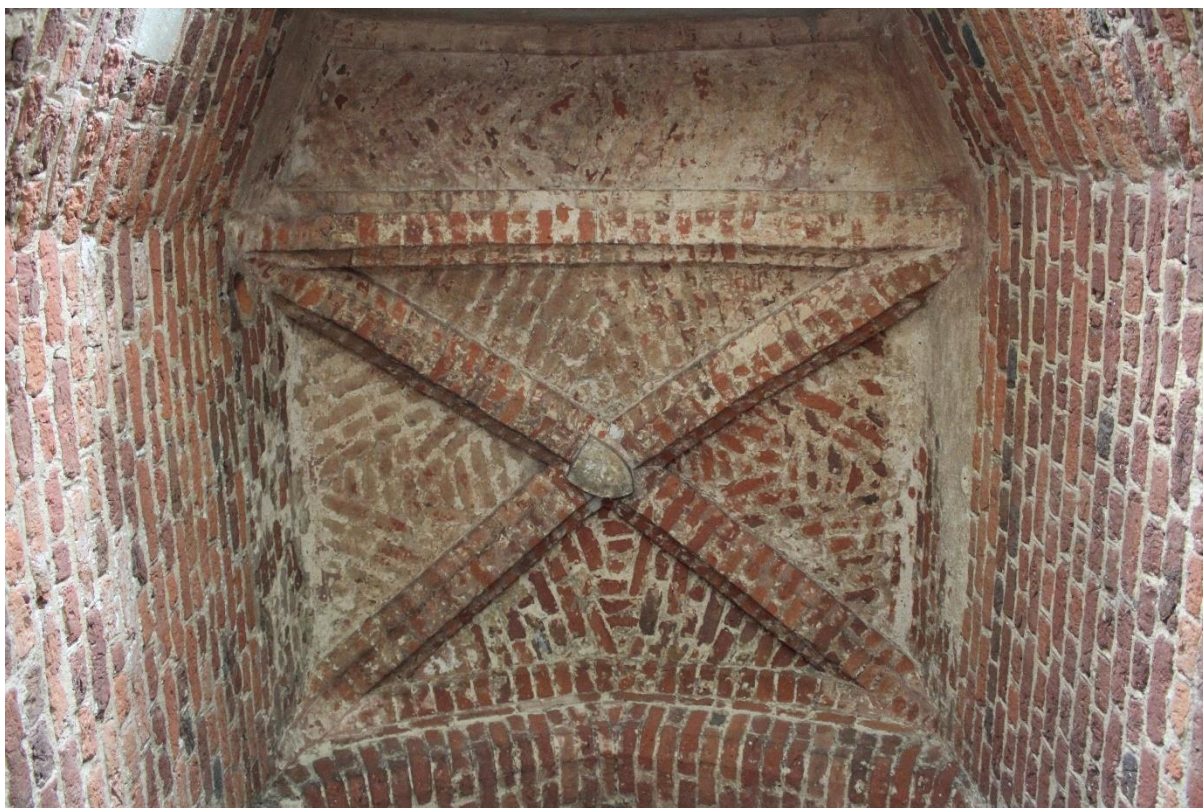
Figure 115 Vaulting of first floor south-western window
