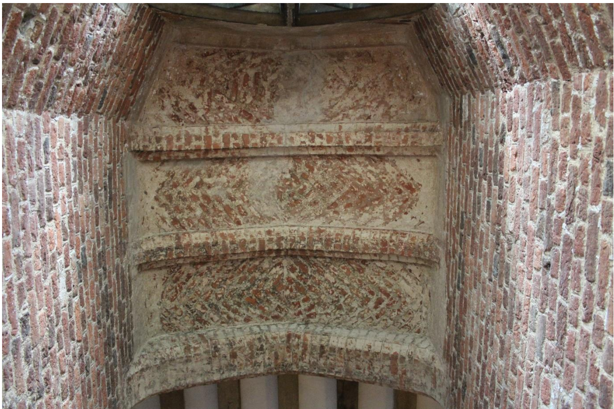
Figure 113 Vaulting of first floor south window
