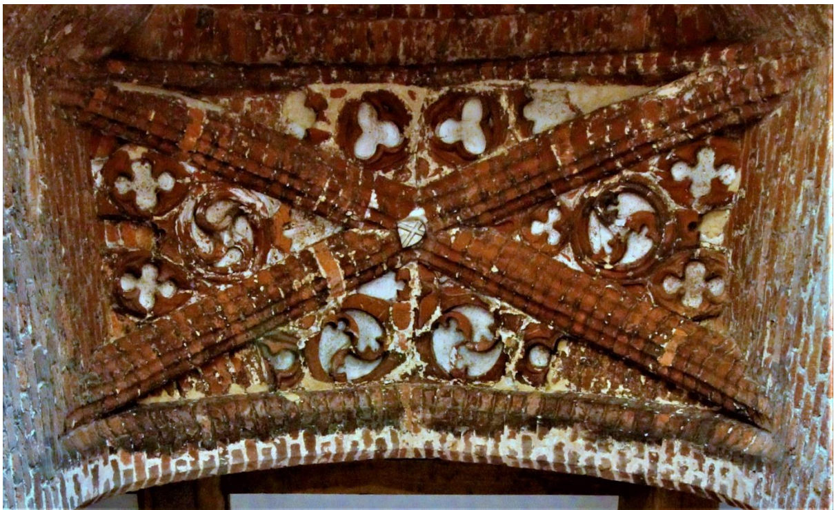
Figure 129 Vaulting of third floor chamber north-west window
