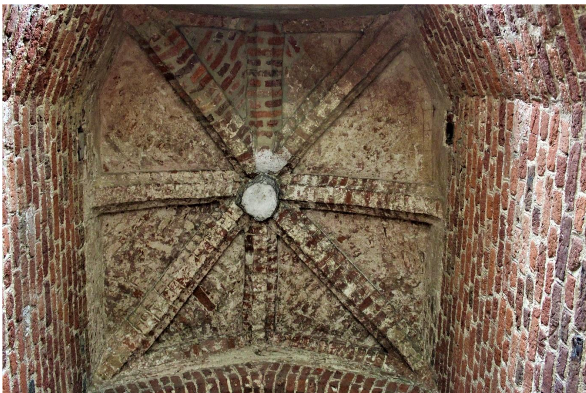
Figure 114 Vaulting of first floor north-western window
