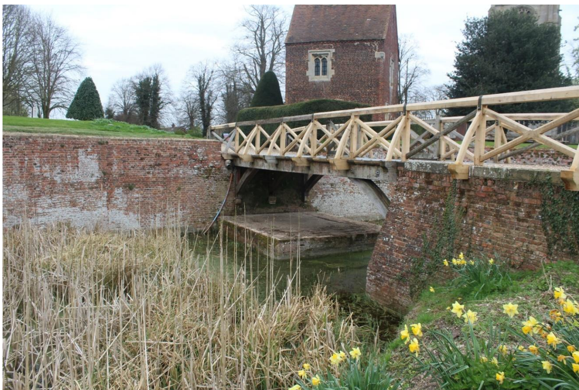
Figure 15 Thirteenth century bridge abutment encased in mid-fifteenth century brickwork
