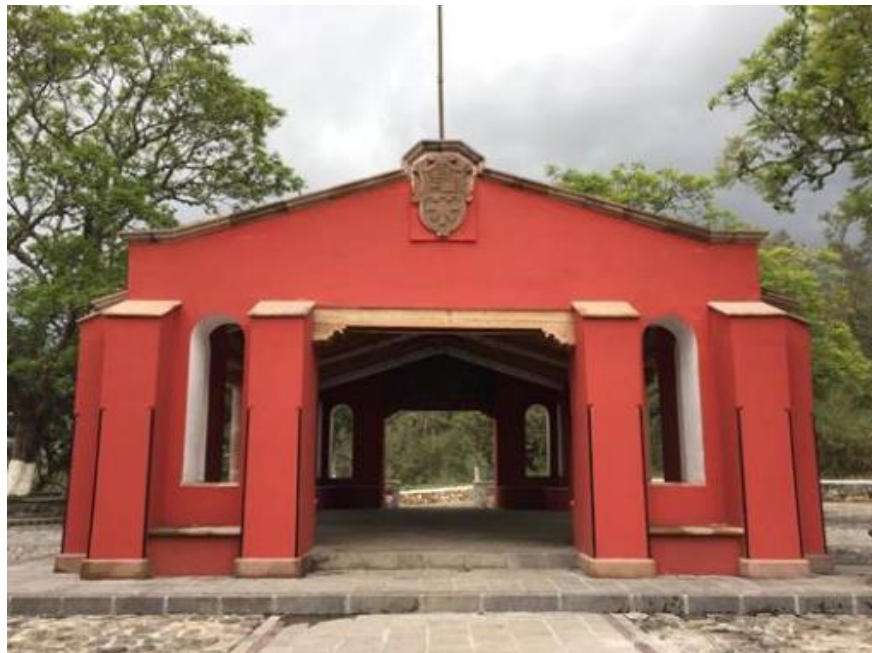
Figure 6.45. Gazebo in the Estribo Chico Viewpoint built in a neocolonial style. Photograph by the author.
