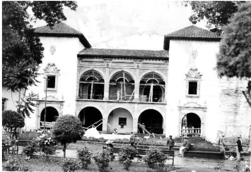
Figure 6.14. Construction of the Emperador Caltzontz'in theatre, ca. 1936. Source: IIE-UMSNH Photograph Archive.
