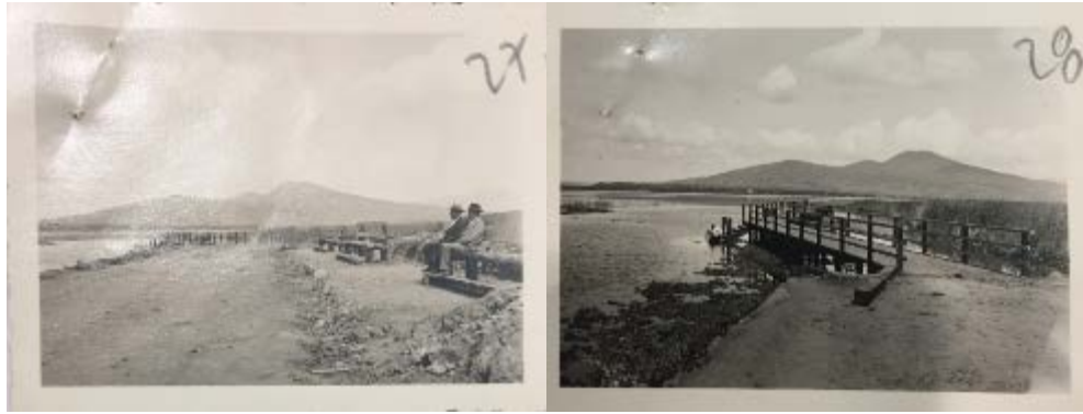
Figure 6.29. Photographs of the works carried out in the proximities of the lake by Ferrocarriles Nacionales de México. Source: Letter from Engineer Antonio Madrazo to the Private Secretary of President Lázaro Cárdenas, January 1936. AGN-AP, Box 625, Folder 514. 63/19
