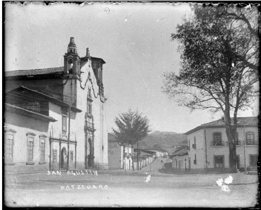
Figure 6.13. San Agustín Complex Convent, ca.1920s. The convent is the low building next to the church. Source: Colección Manuel González Galvan, IIE-UNAM Photographic Archive.
