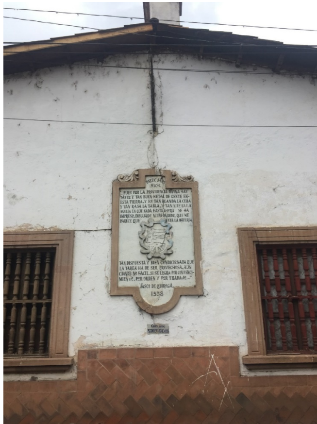
Figure 6.39. The sidewall of Pátzcuaro Service Station. Photograph by the author.
