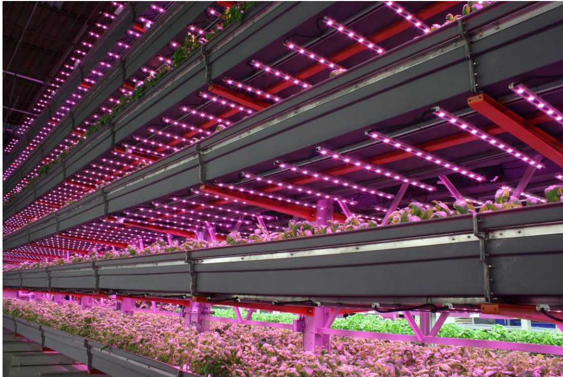
Figure 2. 2 Typical vertical farming facility, Association For Vertical Farming, launched in 2013, USA.
