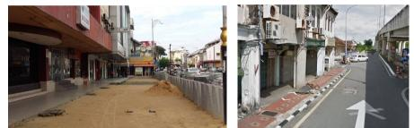
Figure 2 Pedestrian walkway widening project along Jalan Langgar and narrow sidewalk with broken pavers
