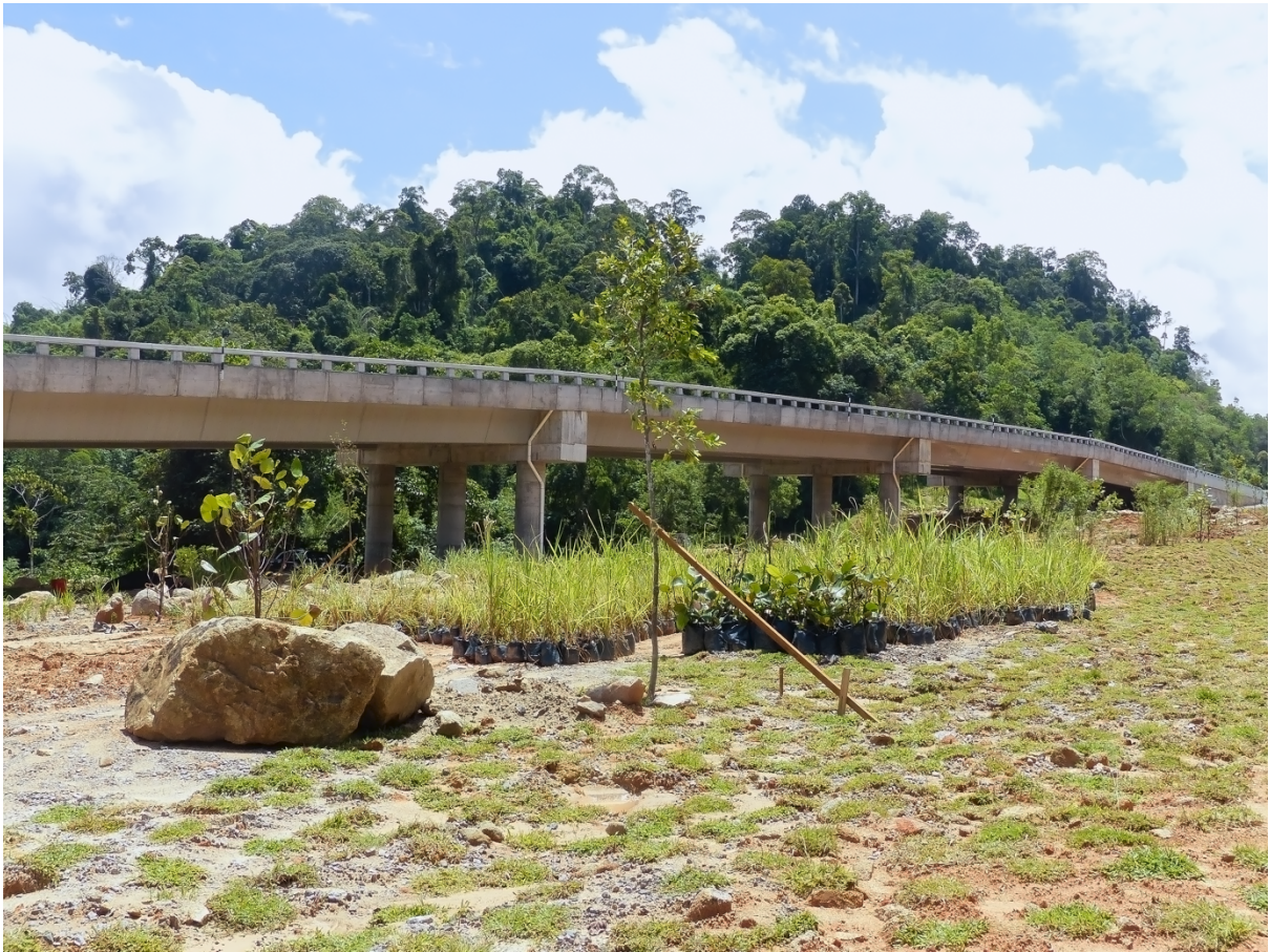
Figure A3-1. Wildlife viaduct in the East-West Highway. The viaduct was completed in September 2015 and its dimensions are 17.4 m width, 8.1 to 11 m height, and 200 m length.
