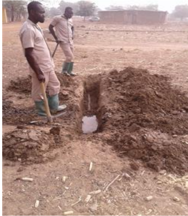
Figure 7.6: Staff of GWCL, repairing leak pipe in Navrongo
