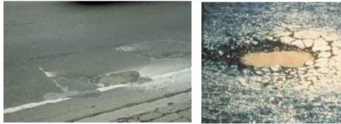
Figure 2.7: High severity patch and pothole (Miller and Bellinger, 2003)
