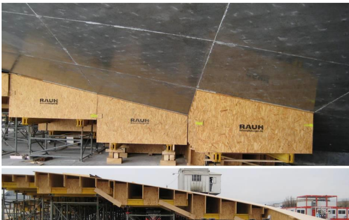
Figure 4-12 Formwork tables on site; after and before concreting (Source: Agnes WEILANDT, Manfred GROHMANN, Klaus BOLLINGER, Michael WAGNER, ROLEX LEARNING CENTER in Lausanne: From conceptual design to execution , 2009)
