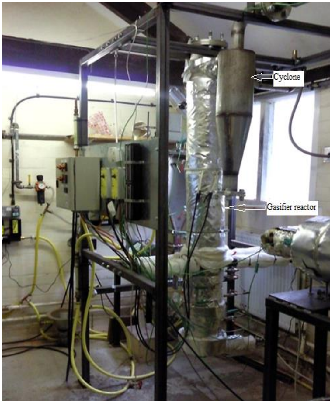
Figure 3-6: Bubbling fluidized bed gasifier reactor and cyclone.
