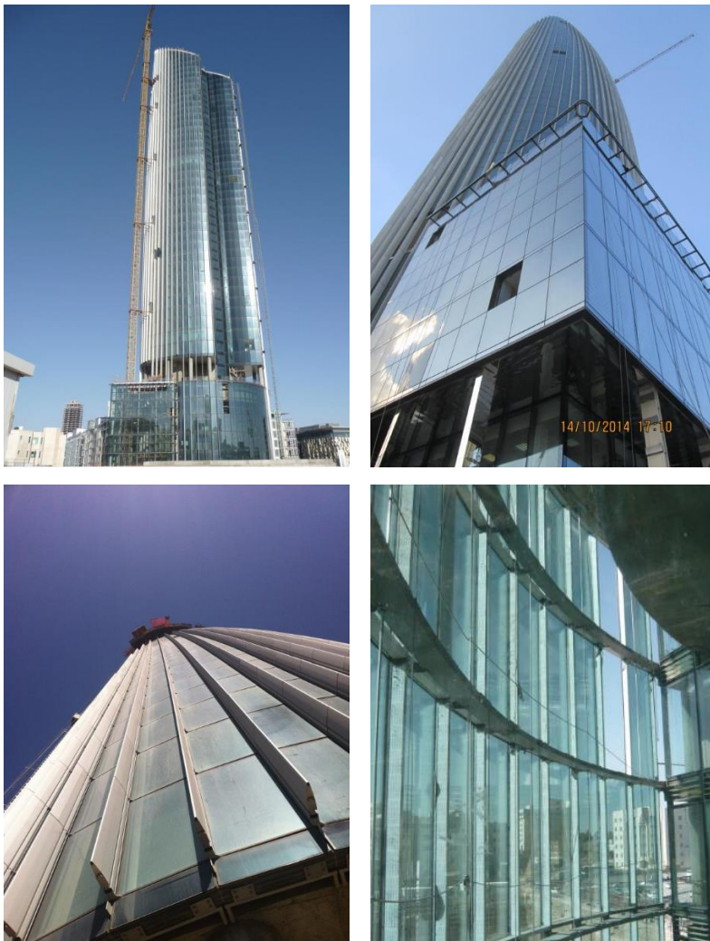
Figure 2.14: Shots of Rotana Amman Hotel in Amman. Full glazed facades with shading elements are shown. Source: (D'ingénierie, 2014).
