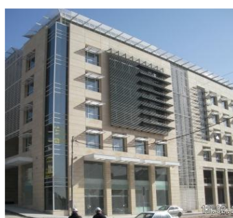
Figure 2.8: Several passive techniques for Building Facades in Abdali Project / Amman, as sample of passive solution for modern buildings in the city. Source: (Abdali, 2013a).
