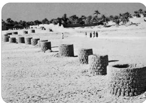
Figure 4.1: Weels of the Fougara. Amara, Nordell and Benyoucef, 2011
