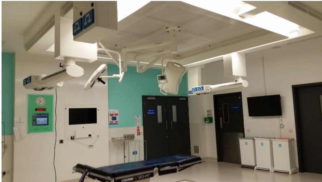
Figure 6.15 Laminar flow ventilation unit in the theatre
