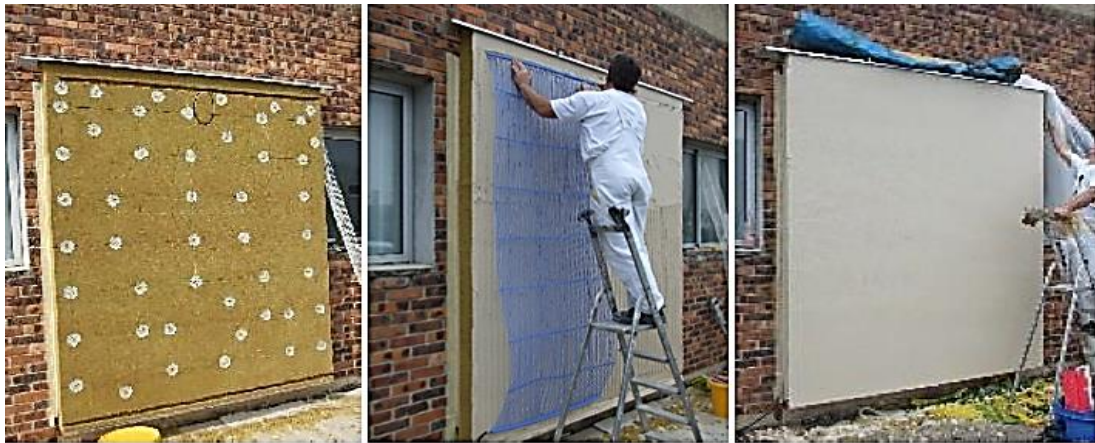
Figure 3-8 Collector installation for Long-term laboratory tests of the integrated concept (ESTTP, 2009)
