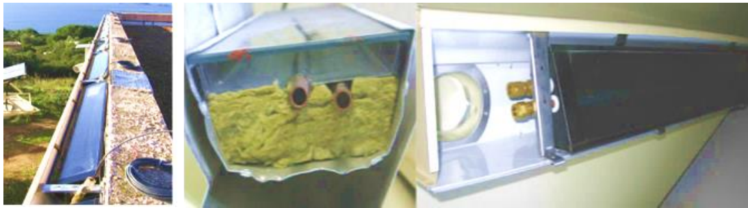
Figure 3-4 Structure of solar water collector of H2OSS (Motte et al., 2013b)
