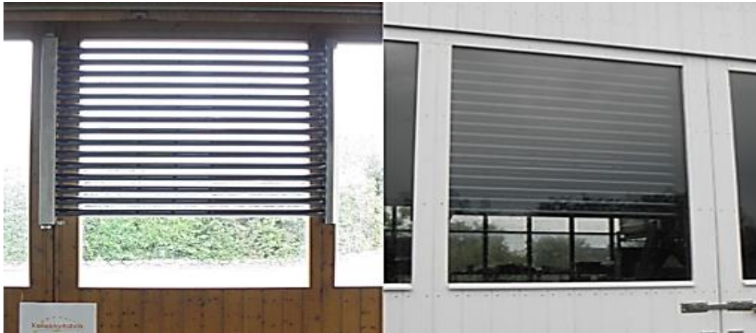
Figure 3-7 Prototype of air collector mounted at the windows of Kollektorfabrik storehouse (Kollektorfabrik, 2011)
