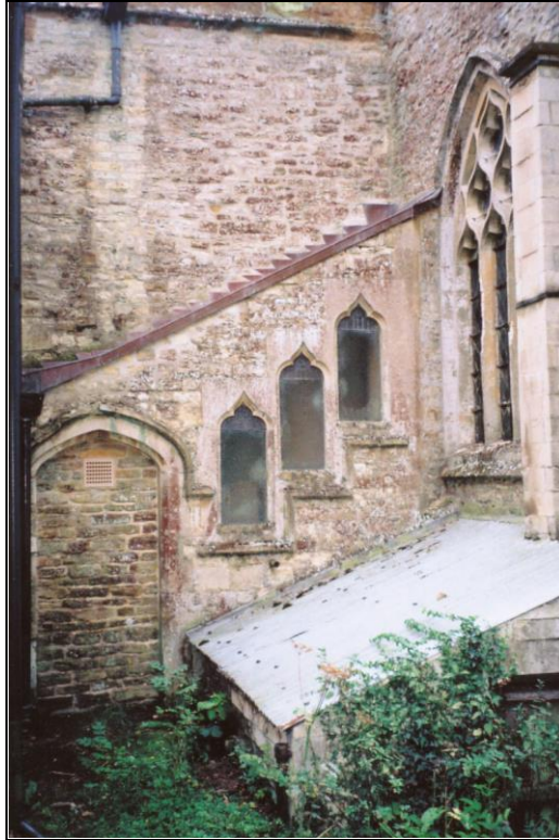
Fig. 2.2 : Stoke Bruerne: the blocked exterior doorway to an unusual straight staircase to the rood-loft. Stairs generally spiralled inside the internal structure.
