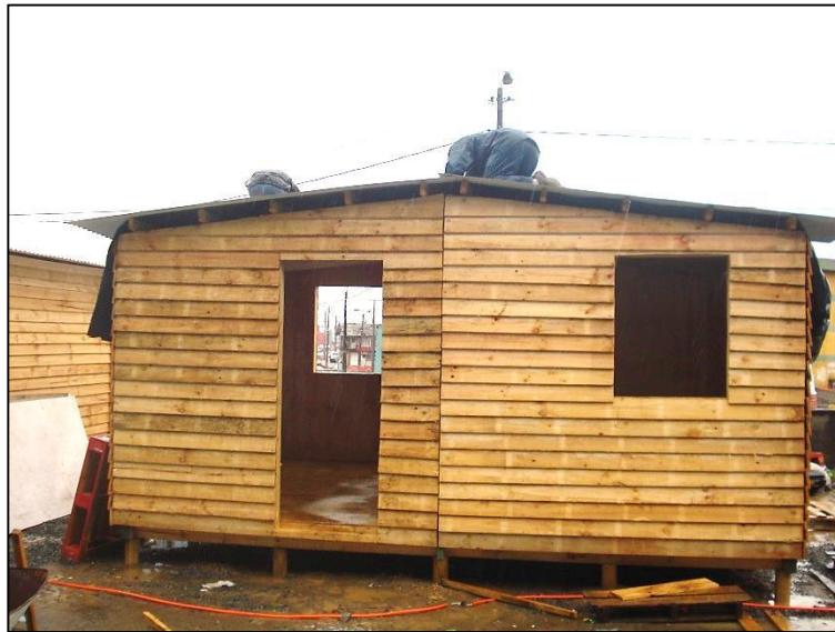
Figure 8.1. Temporary house or 'mediagua' in El Morro (Source: Talcahuano City Council, 2010)
