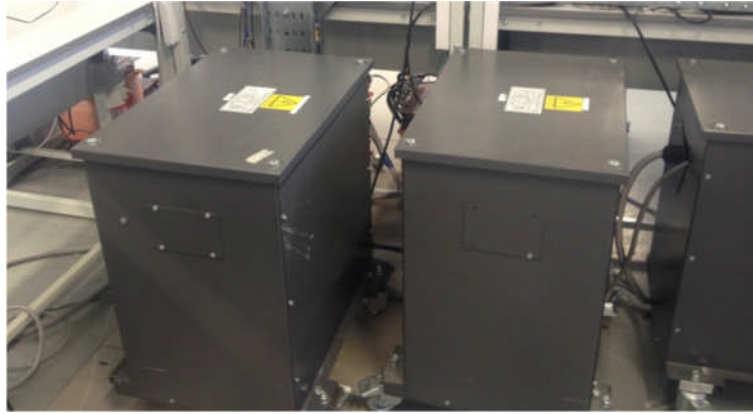
Figure 8.7. Isolation transformers.
