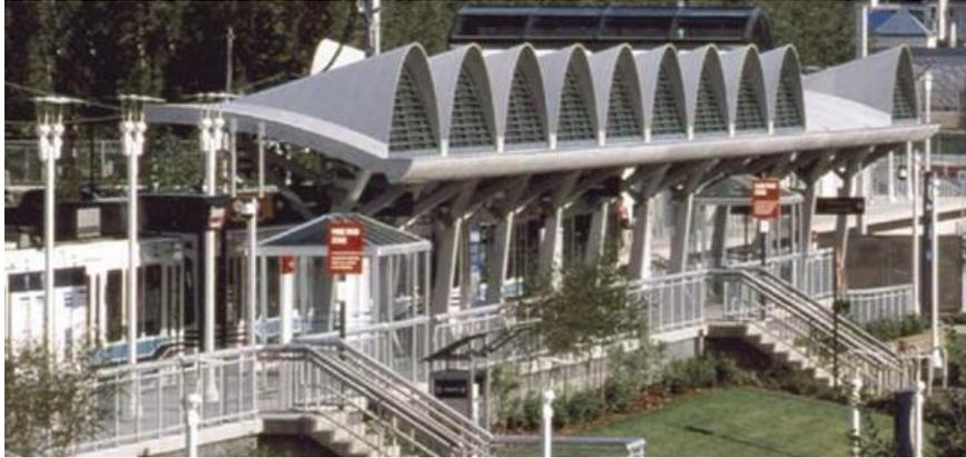
Figure 2.15 Train station roof supported by a single line of columns (Vicenzino *et al.*, 2005)
