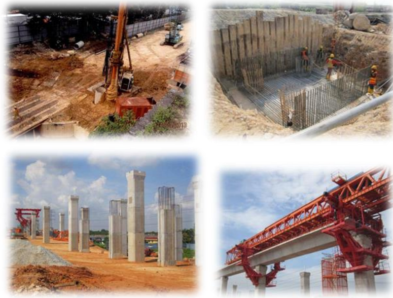
Figure 3.1: Main Construction Scope of Elevated Guideway in Kelana Jaya Extension Project
