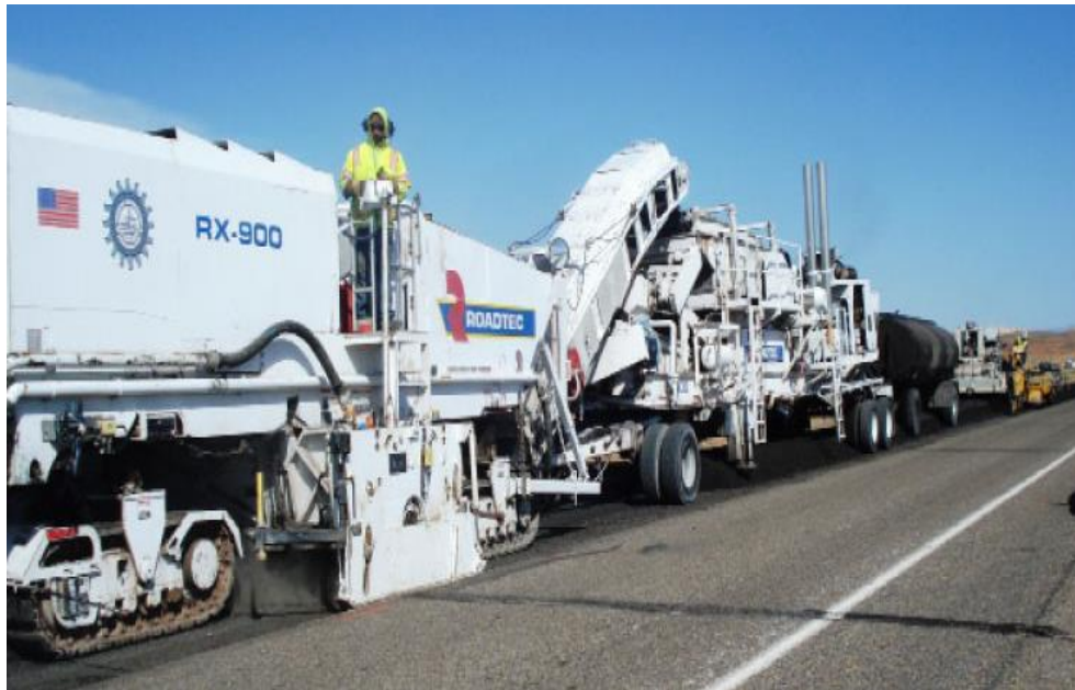
Figure 2-5: Cold in-place recycling train (Roadtec, 2015)
