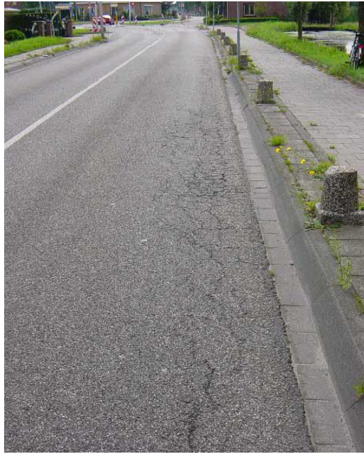
(a) Longitudinal and Alligator Cracking
