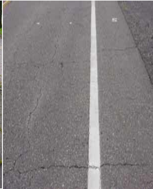
(b) Transverse Cracking
