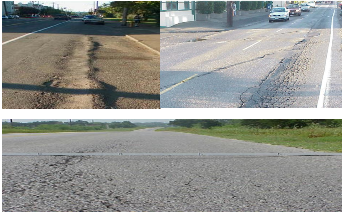
Figure 1.1 Permanent deformation in asphalt pavement (Science, 2014)
