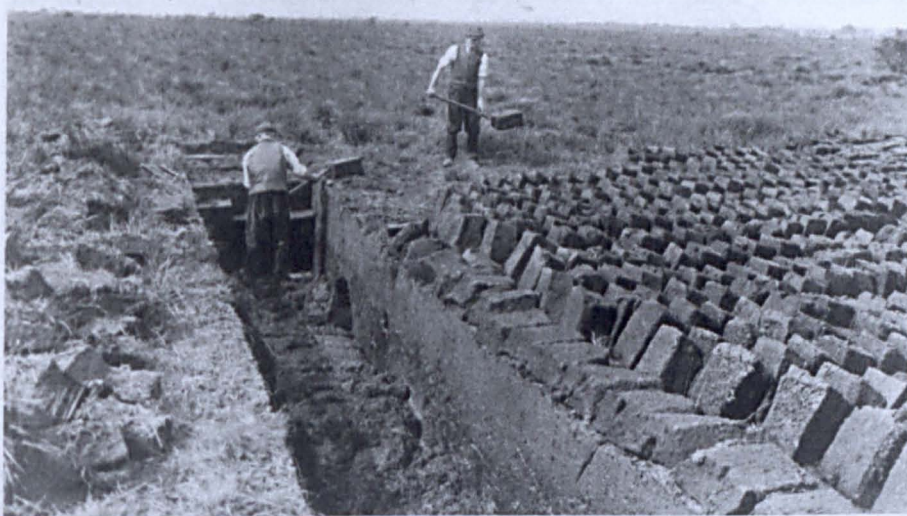
Plate 1.2: Construction of open drains using traditional peat cutting methods circa 1887. (Courtesy of the collection of Dr Phillips).
