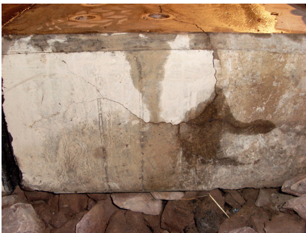
Figure 3.4 Cracked bearer
