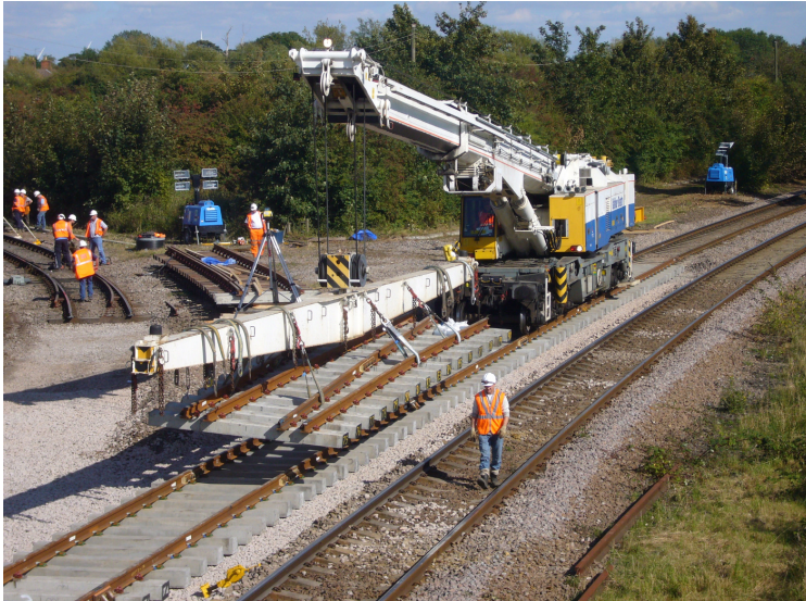
Figure 5.3 March West installation crane
