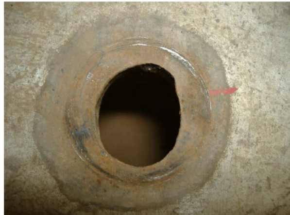
Figure 4.2 Shroud plate not cut to specification
