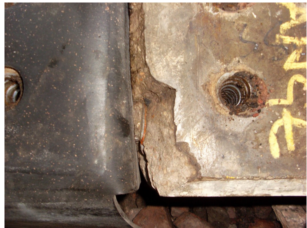
Figure 3.5 Broken bearer
