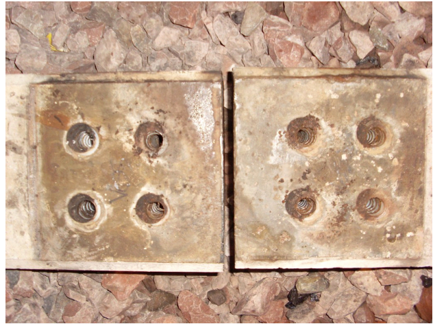
Figure 4.4 Voiding and alignment issues
