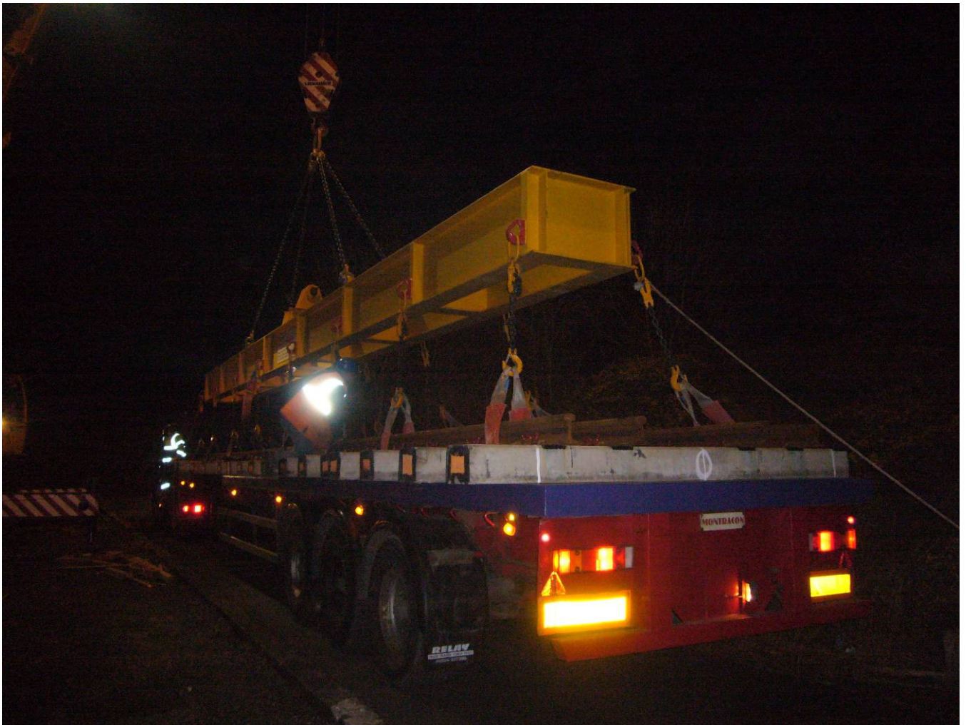
Figure 3.1 Delivery of the first S&C panel
