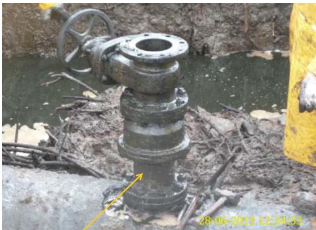
Plate 3-4: Arrow pointing at an illegal valve on a 28" pipe; picture taken on 28 th June 2013 (Shell Nigeria, 2013d).
