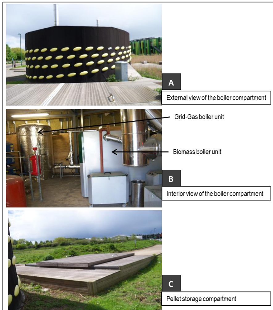
Figure 7.3: The Boiler Plant at No.1 Nottingham Science Park
