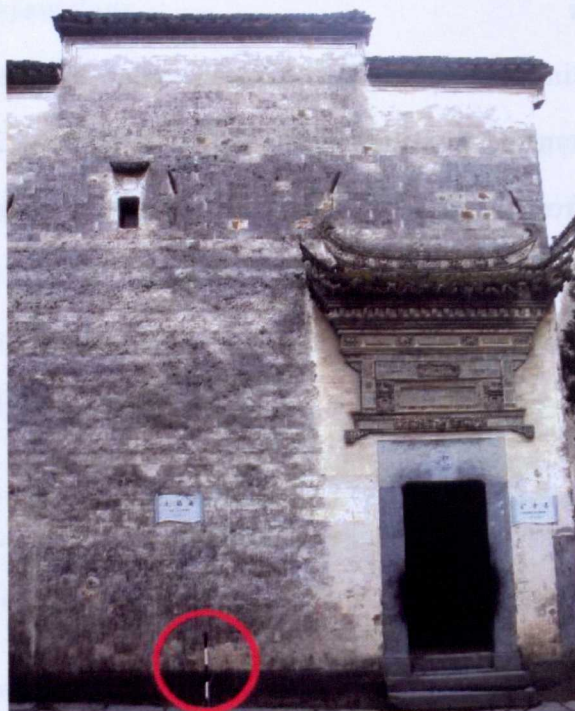
Figure 1. 1 Reference stick attached to the wall that needs to be measured
