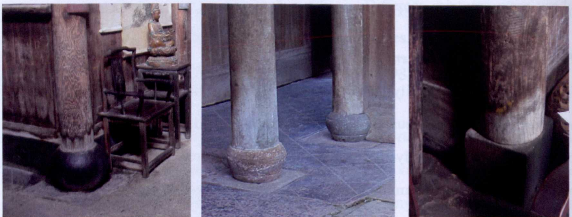
Figure 4. 19 Base type in Xidi village (left), Yuyuan village (middle) and Zhifeng village (right)
