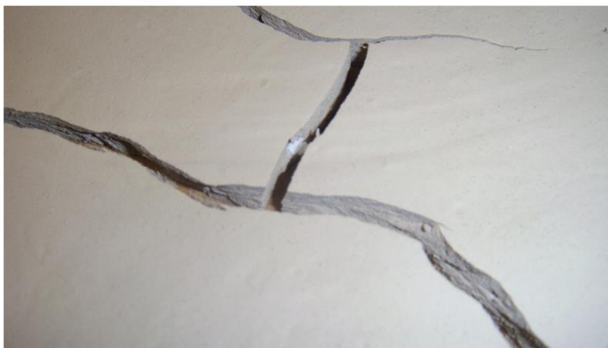
Panel 2 Cracks
