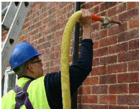
Figure 4-11 Injecting the insulation into the cavity wall (Lgloo insulation, 2011).
