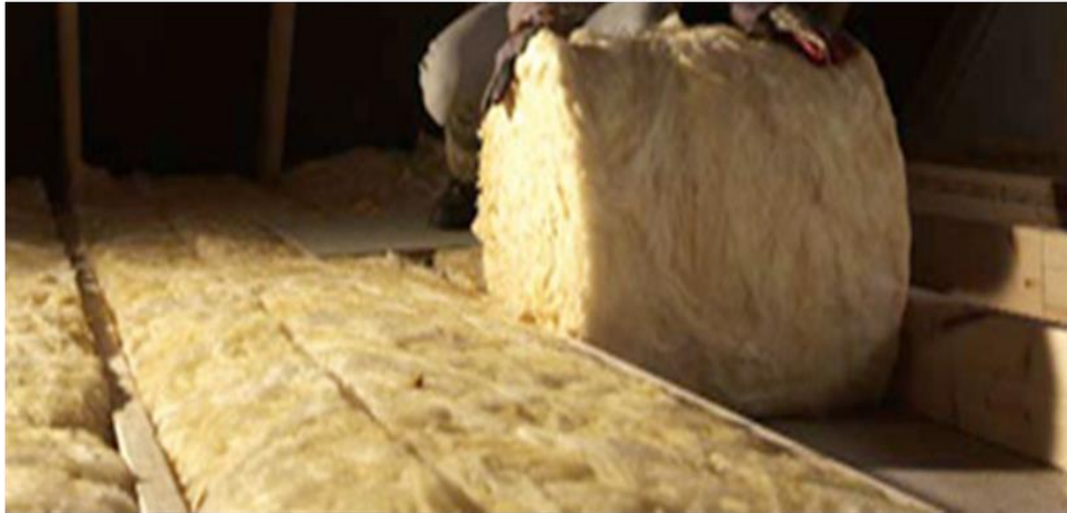
Figure 2-11 Installing Glass wool in a pitched roof.
