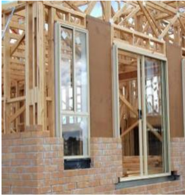
Figure 2-7 Timber frame with brick cladding (Sahota, 2012)
