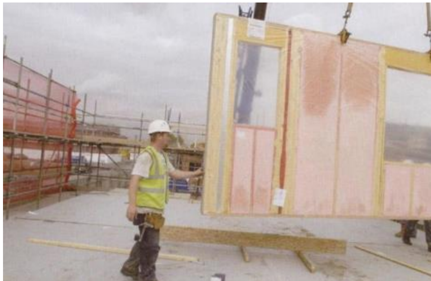
Figure 2-9 Timber frame wall (Patrick, 2007).
