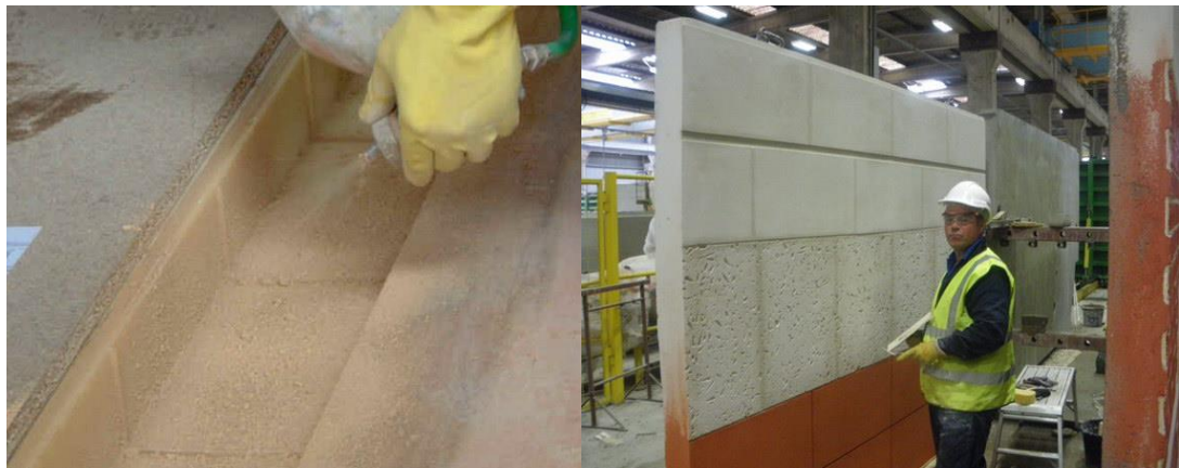
Figure 4-1 Tru-Stone coating applied by spray or trowel (Tru Stone, 2010c).
