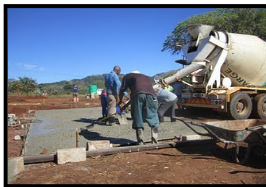
Figure 93: The concrete flat base (Holley, 2011)
