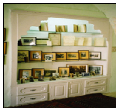
b) The wall thickness has been taken advantage of to install a cupboard. It was originally built as a ' Qaws Elferash ' before converting it later to be used as a cupboard. Located in a bedroom in Bethlehem City.
