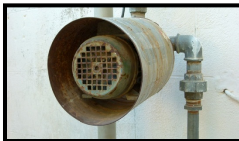
Figure 225: Uncovered water pump in the outdoor play area, that is reachable by children
