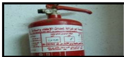
Figure 273: According to the label, this fire extinguisher should have been refilled in May 2008
