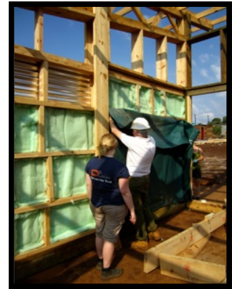
Figure 96: Fitting insulation and a deep proof membrane into the timber stud wall and an internal ply wood cladding (UoN, 2011).
