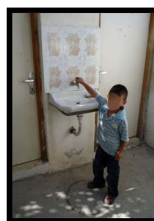
Figure 145: Sinks at inappropriate level for child's use
