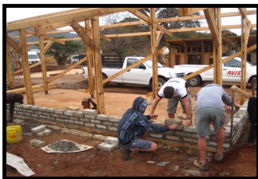
Figure 92: Block walls. Photo by William Holley (Holley, 2011)
