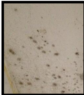
Figure 176: Mould on the KG lavatory ceiling
