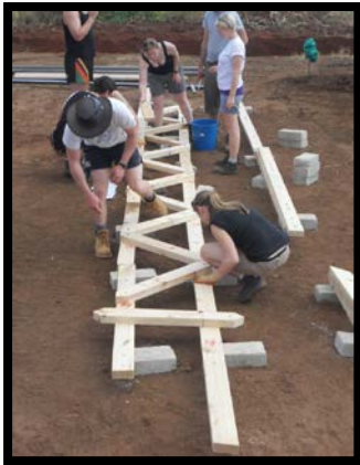
Figure 94: timber roof trusses. Photo by (Edmonds, Letter from Limpopo, 2011).
