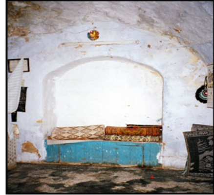
Figure 25: The above photos show the storage spaces in the interior walls ‘Qaws Elferash’. These can be found in all types of traditional houses (type one).
