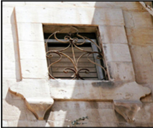
a) A square vent contains horizontal wooden blades, which have the ability to be opened and closed by changing the degree of the blades. It has an iron protection. Mengo's house, Nablus.
