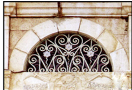
d) An arch vent, which is located above the main door, in Haddad's house has a floral metal decoration in the middle for protection, 1928.
