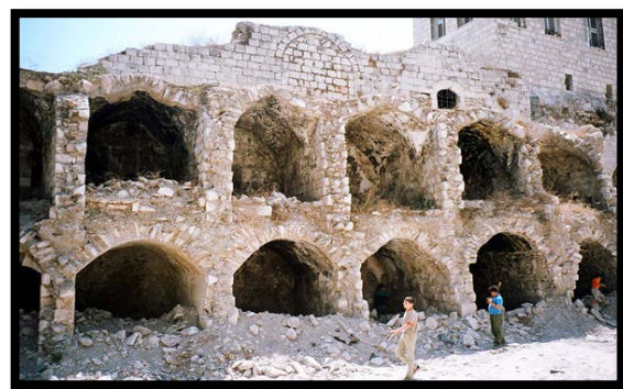
Figure 121: Section shows the building methods in distribute the load in 'multi-storey' the traditional building in PS. Nablus City (2005)
