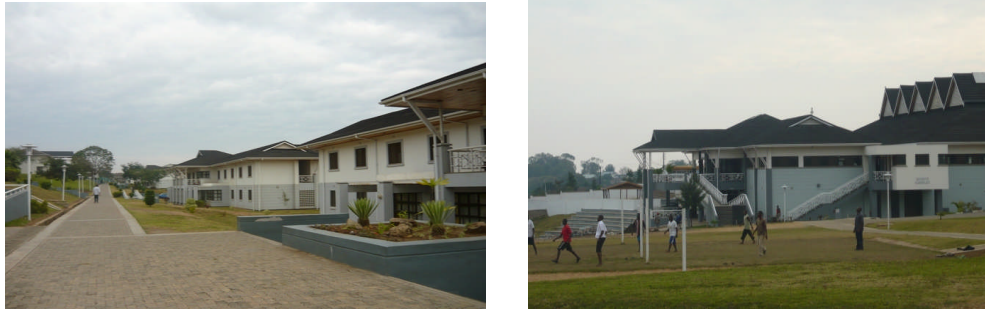
Figure 7-3. The infrastructure built from Norwegian aid.
