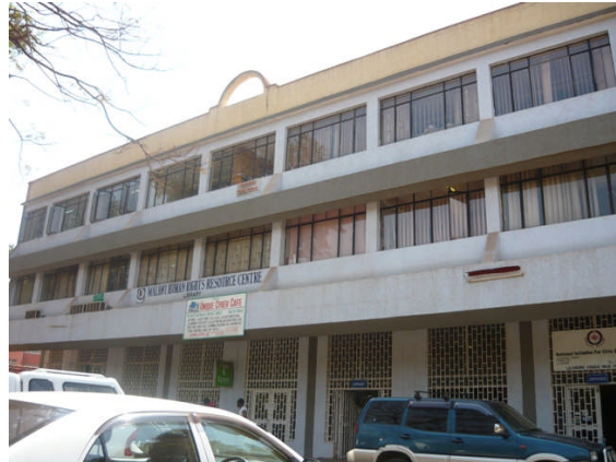
Figure 7-6. The building of Malawi Human Rights Resource Centre.
