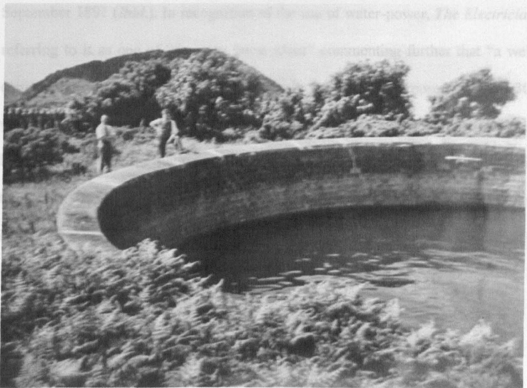
Figure 4.2.7d Reservoir on Summer House Hill which supplied the pumped storage scheme at Lynmouth, nd
