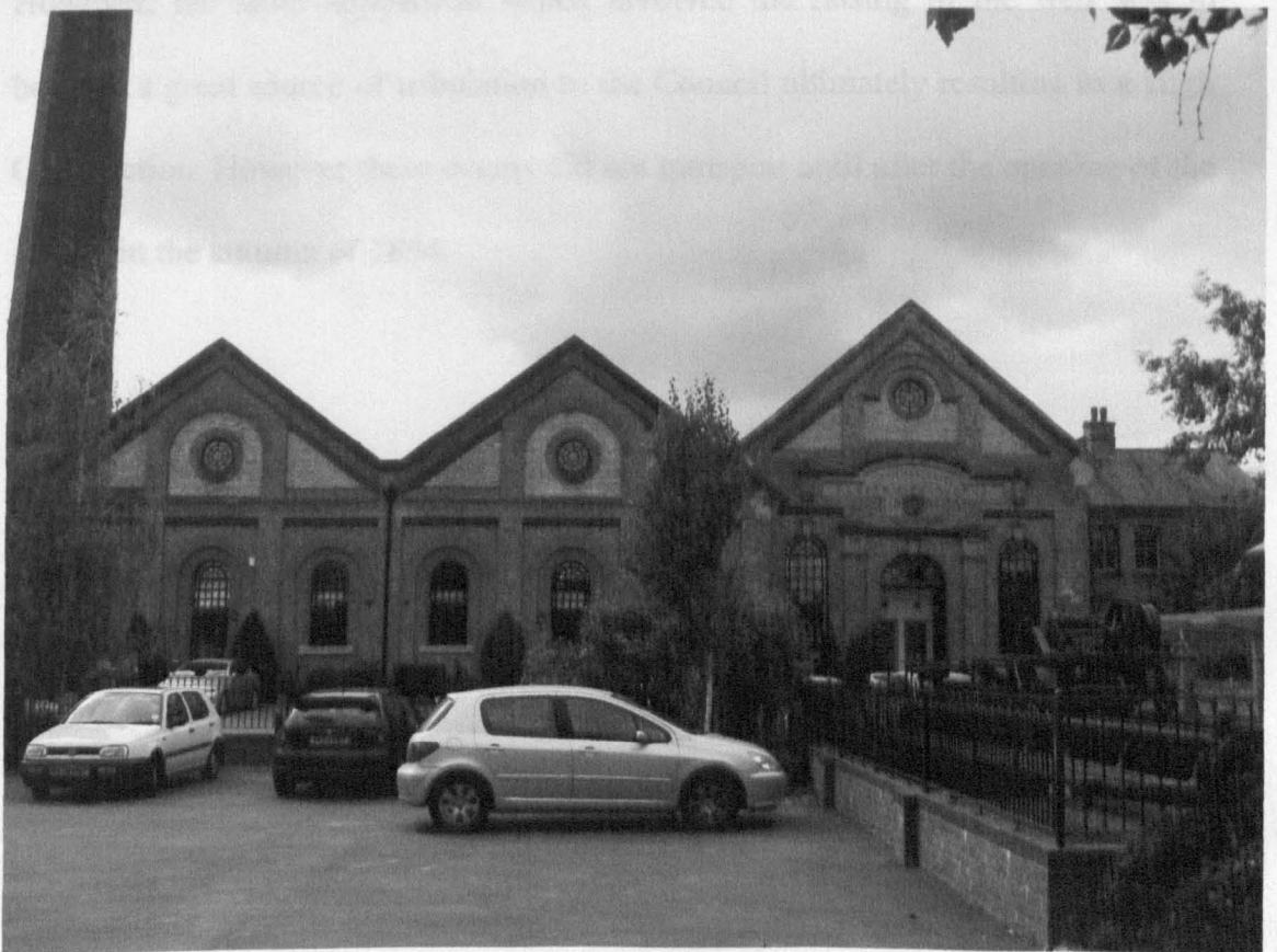
Figure 5.3.5 The front elevation of Powick Mills Source: Author's photograph
