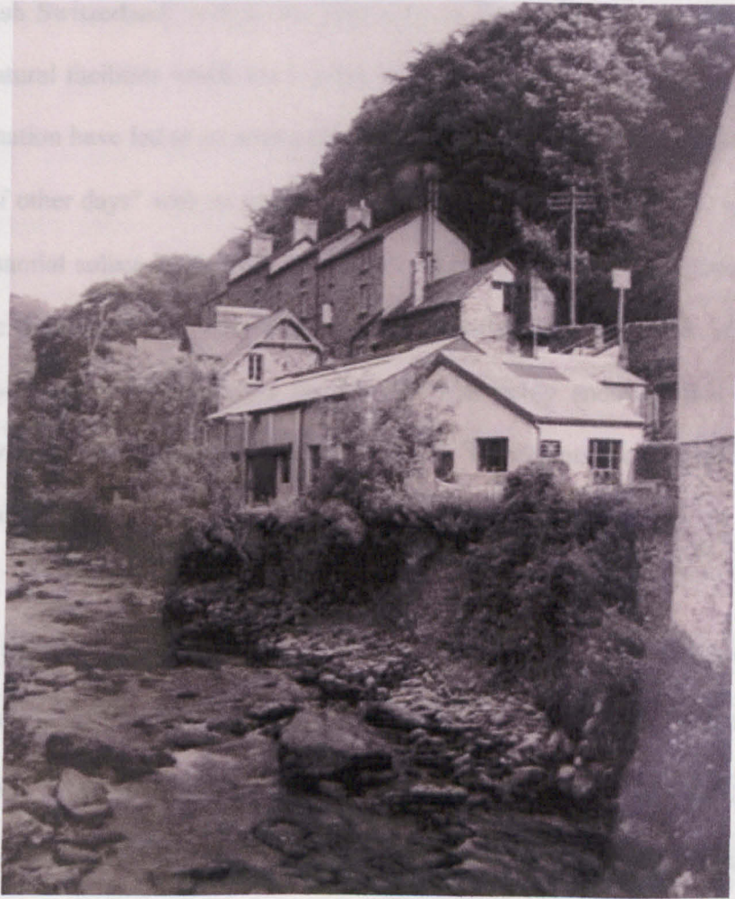
Figure 4.2.7b The hydro-electric generating station at Lynmouth, n.d.
