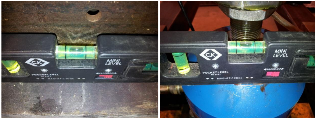
Figure 3.11 : Leveling work
