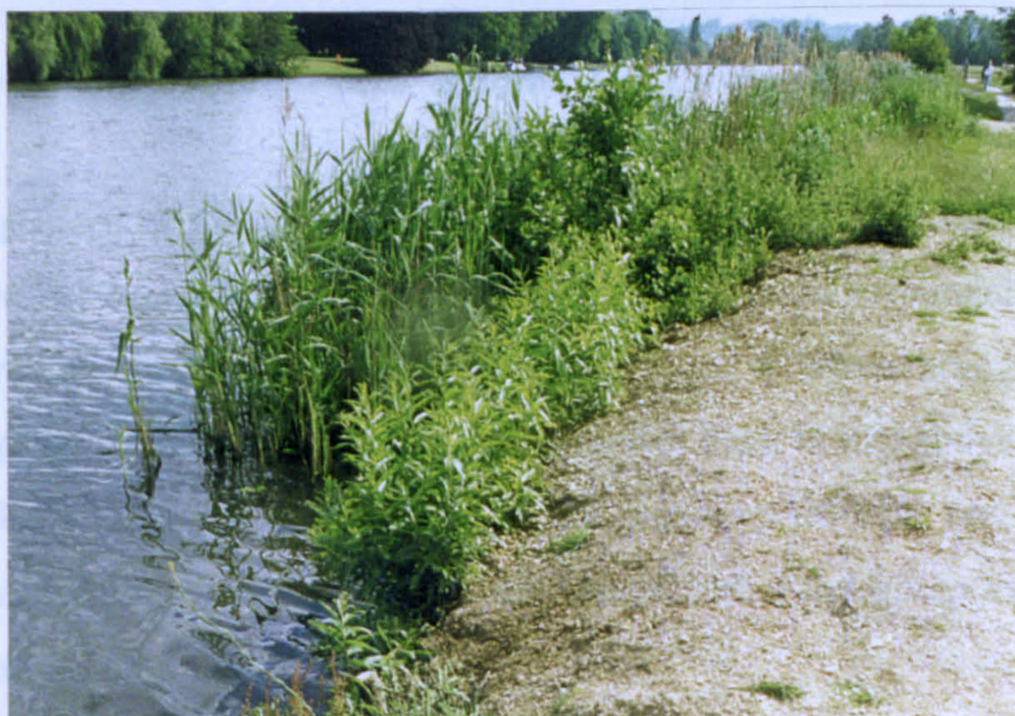
Plate 6.24 Case study no. 14: willow spiling bank protection along Marlow Reach.
