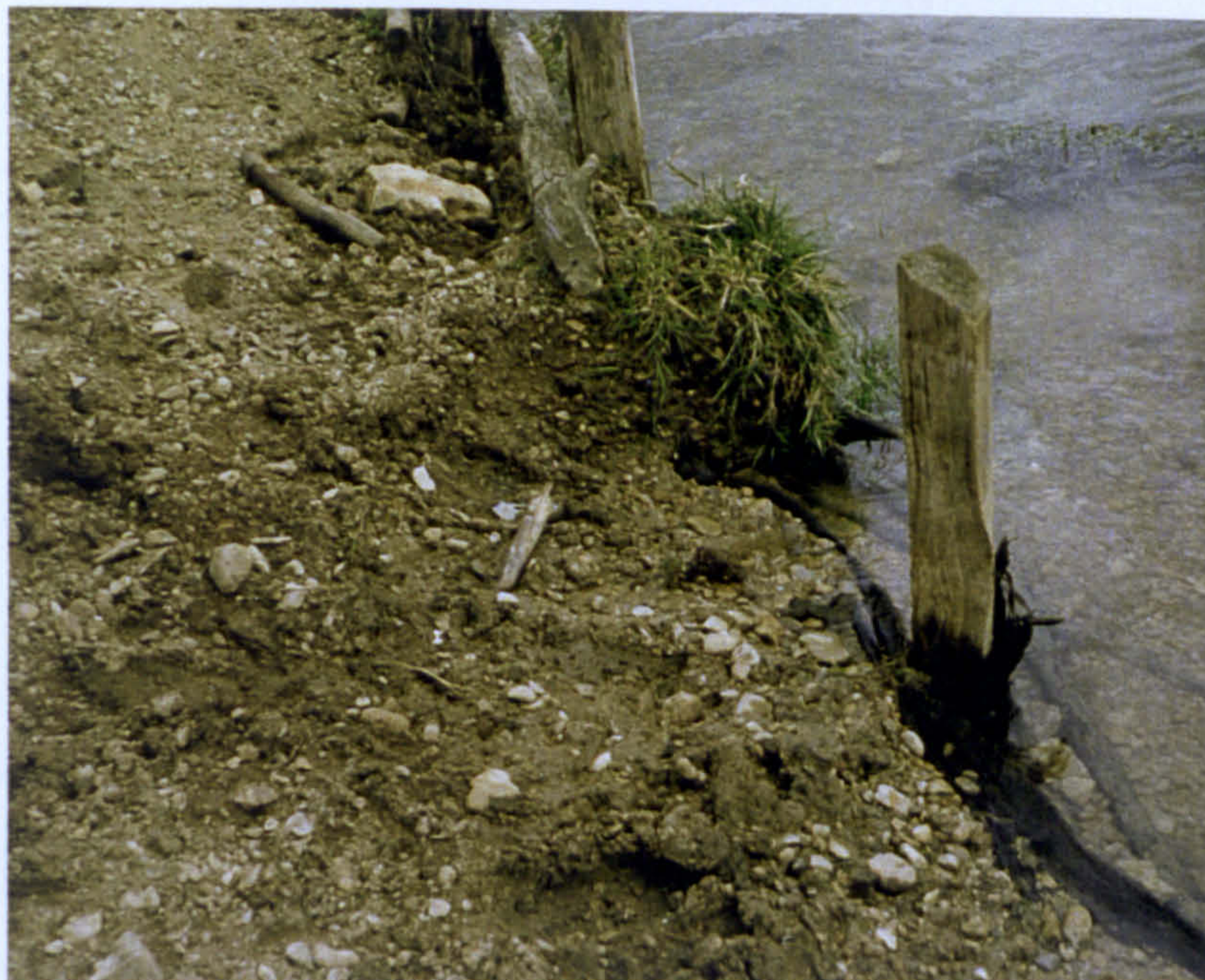
Plate 6.1 Case study no.1: Failed spiling and Nicospan geotextile along Godstow Reach
