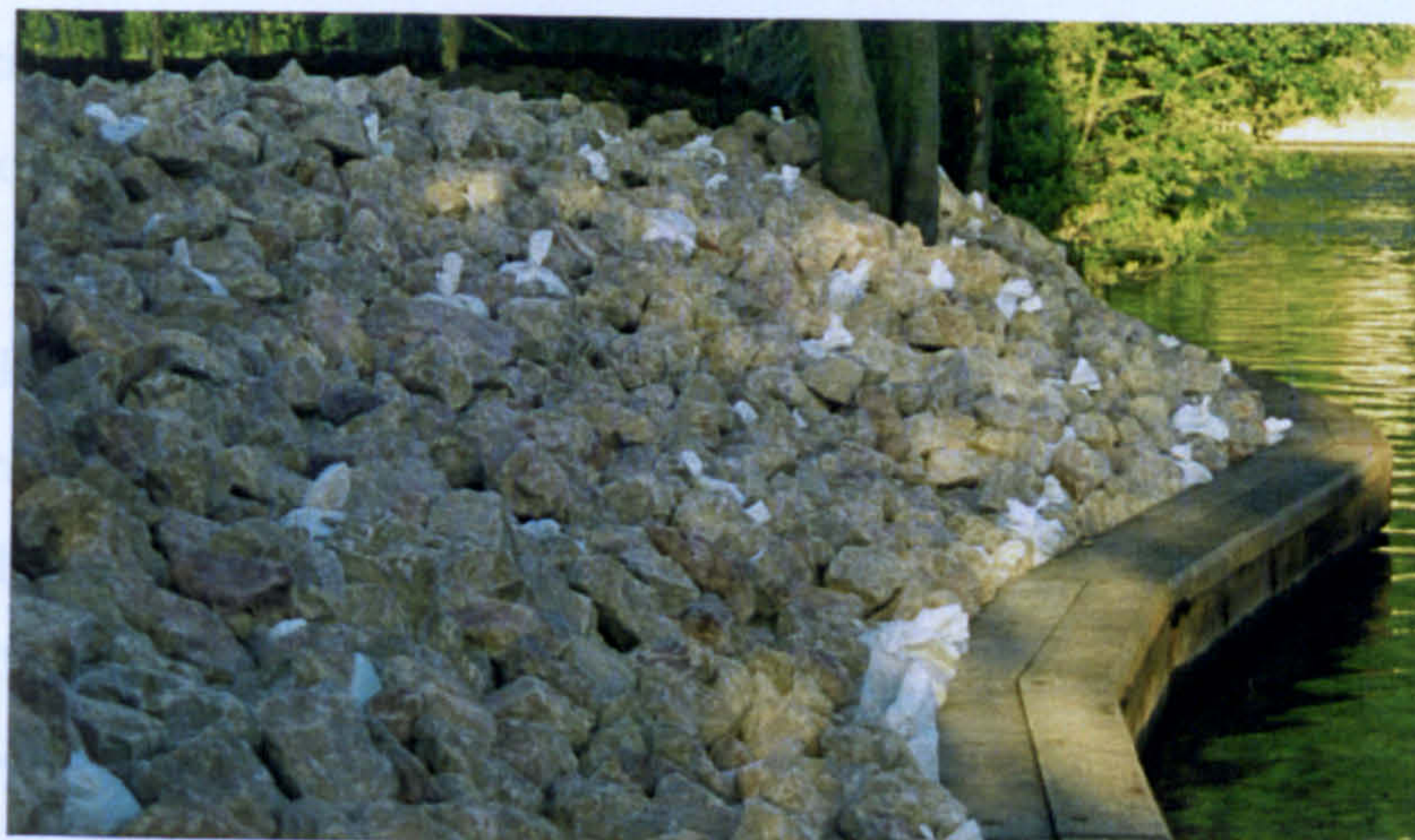
Plate 6.26 Case study no. 15: wood-capped sheet piling and riprap protection along Cookham Reach, after installation in spring 1995
