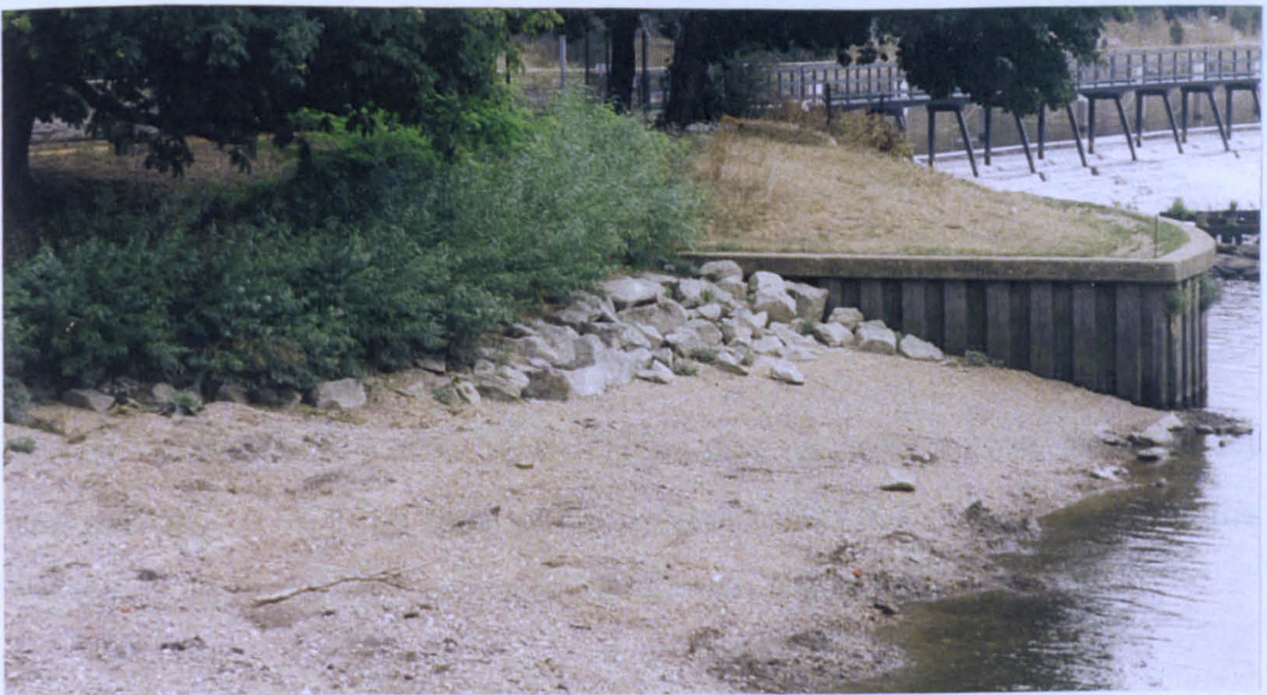
Plate 6.40 Case study no. 21: riprap installed to prevent scour downstream of sheet piling, with Teddington Weir in the background
