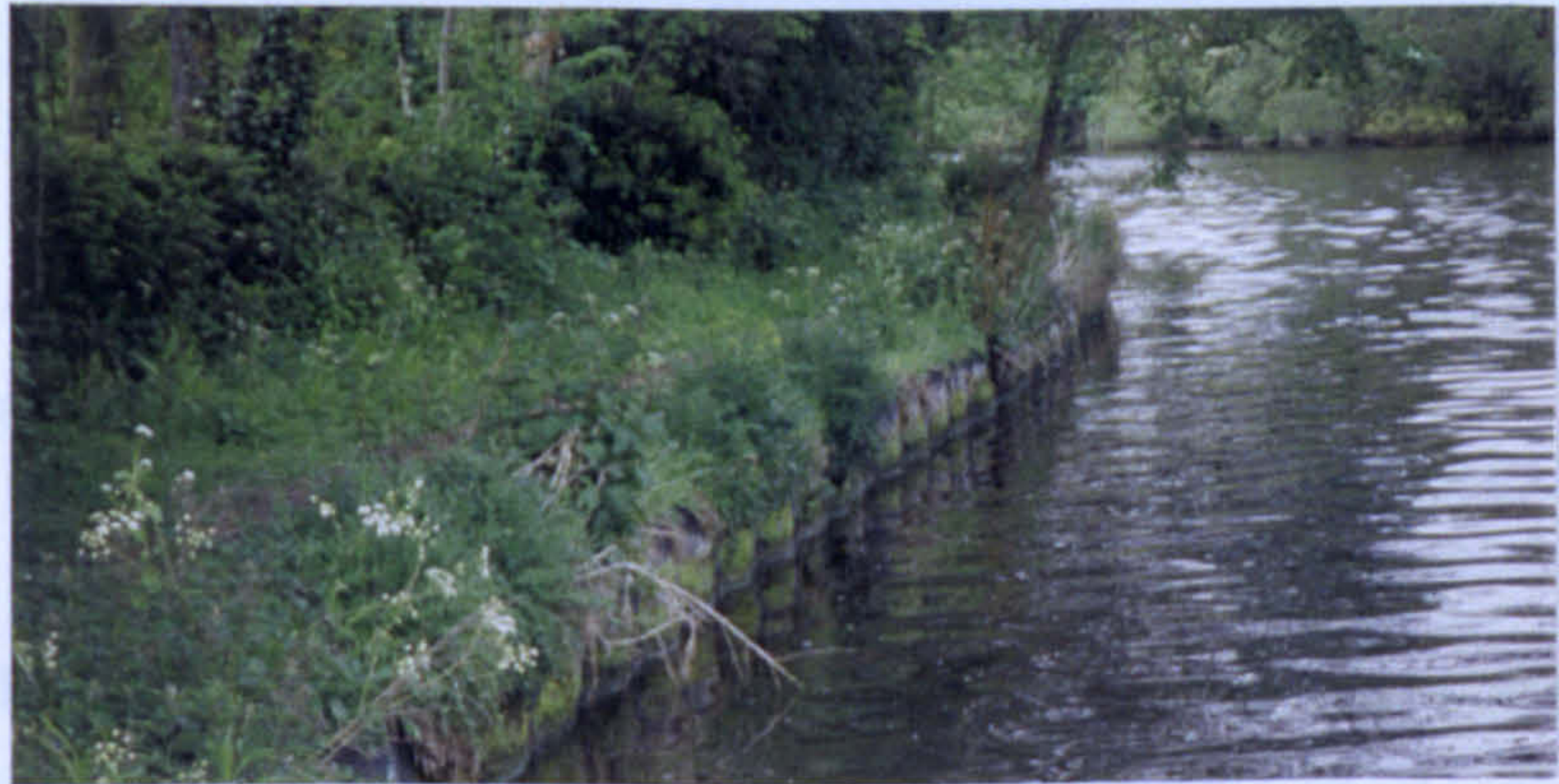
Plate 6.15 Case study no. 10: Nicospan geotextile along Goring Reach
