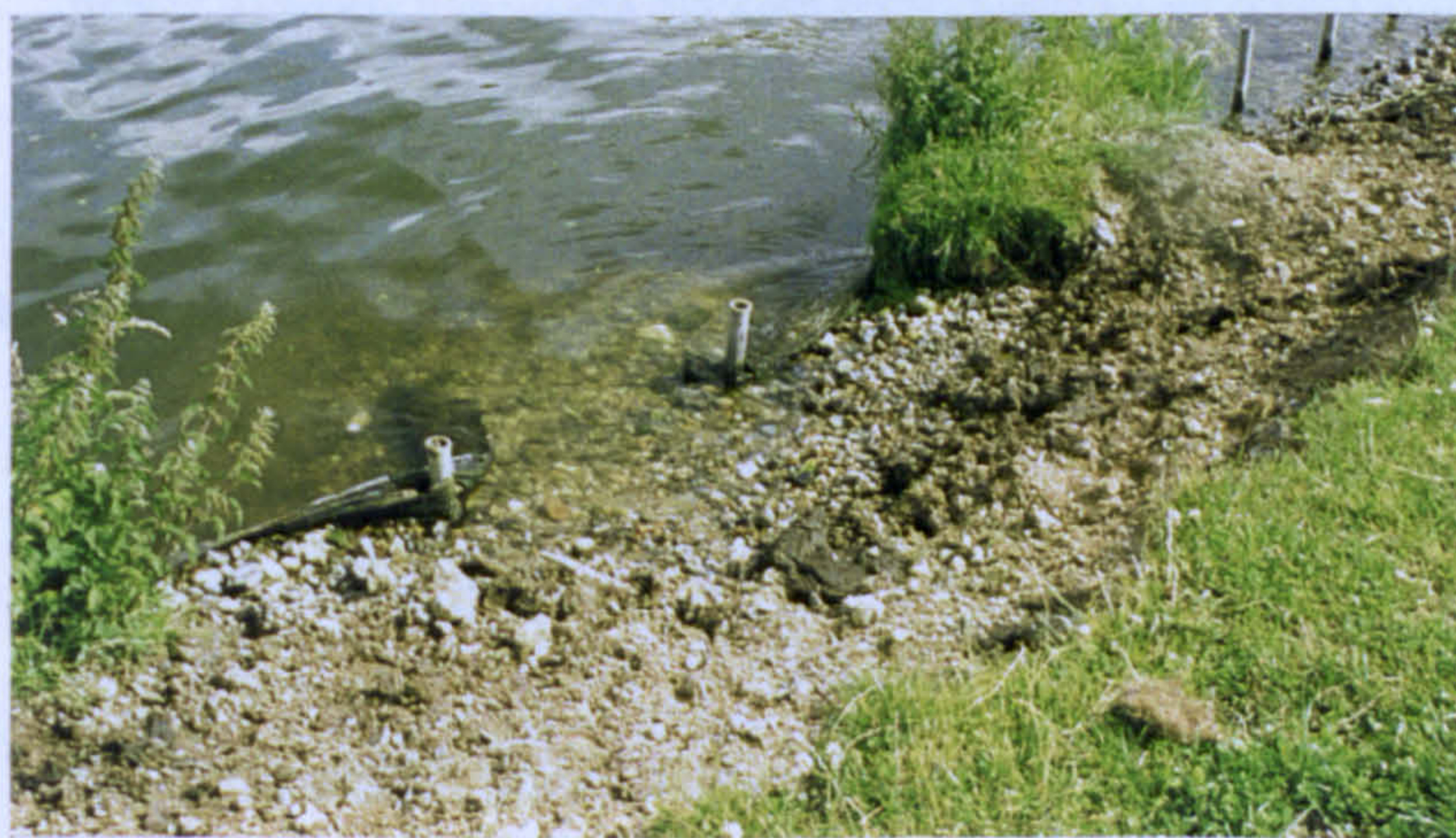
Plate 6.22 Case study no. 13: failed Nicospan geotextile along Marlow Reach
