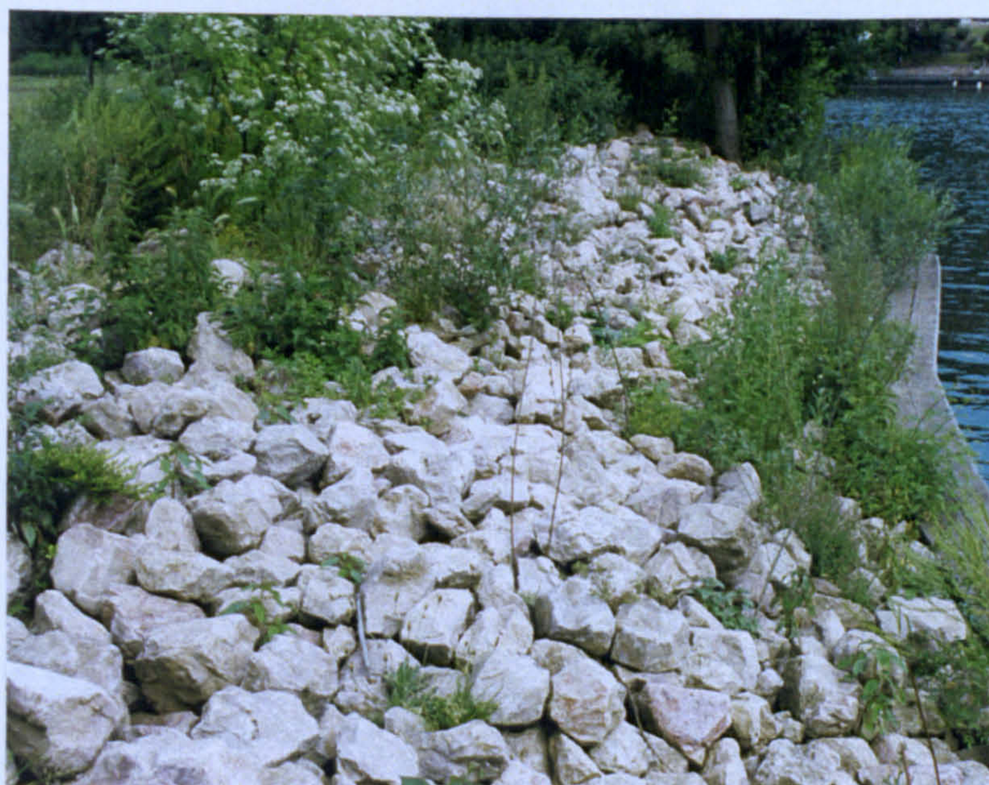
Plate 6.27 Case study no. 15: revegetation of riprap protection along Cookham Reach (June 1997)
