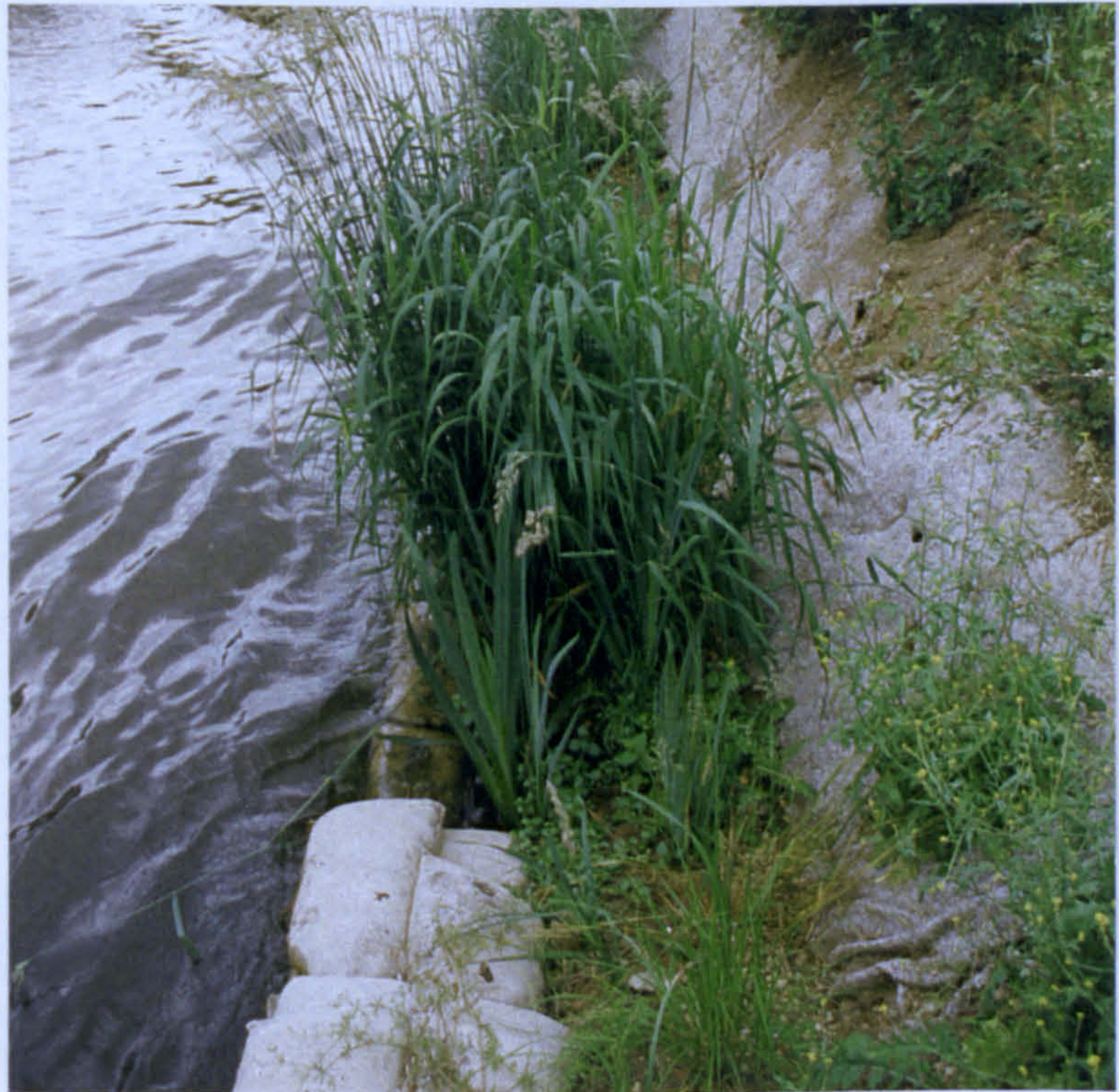
Plate 6.7 Case study no. 7: sheet piling and concrete bagwork along Clifton lock cut. Mitigation measures included reed planting in coir rolls on a low-level shelf.
