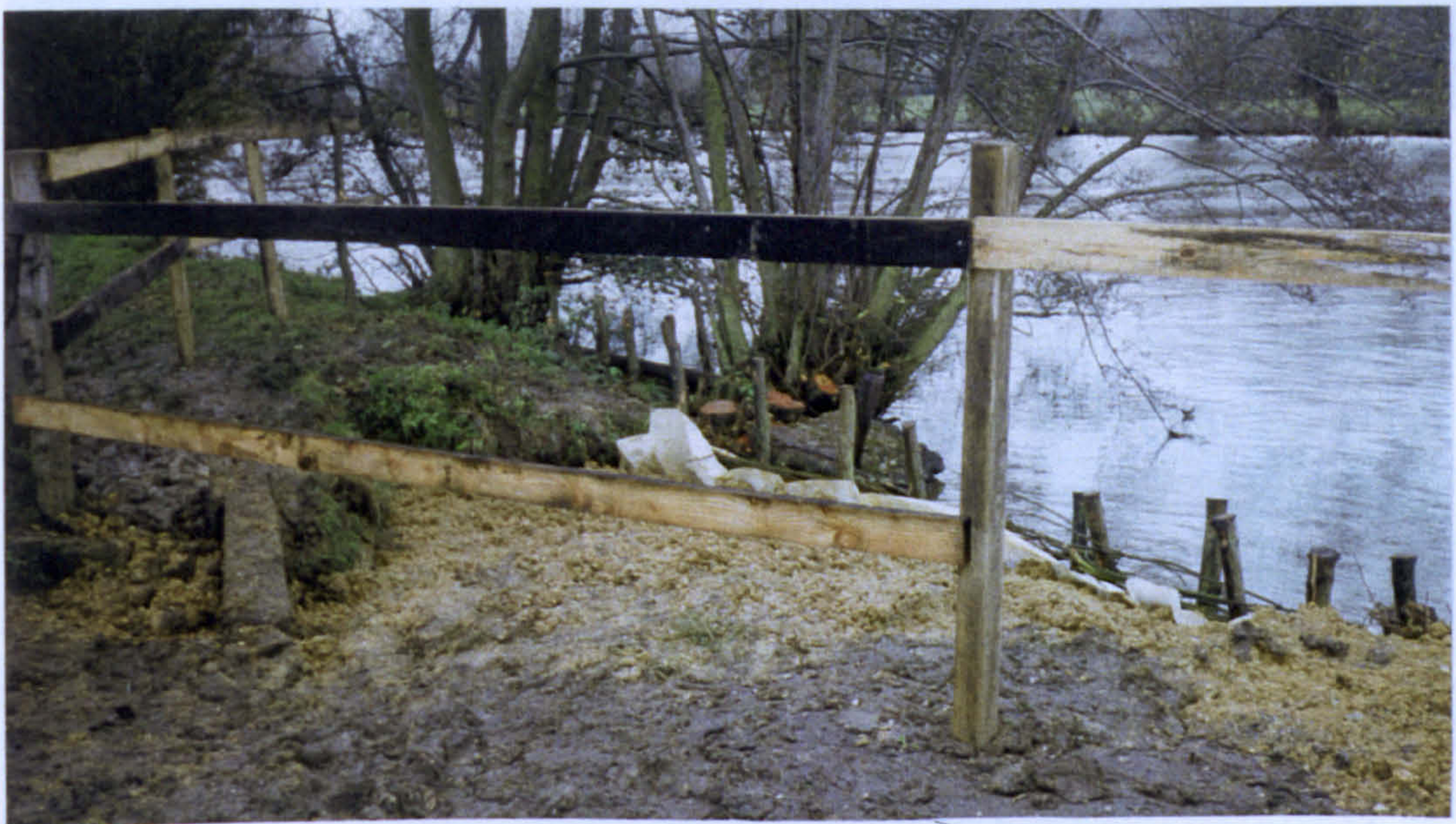
Plate 6.19 Case study no. 11: willow spiling along Mapledurham Reach, with fencing to prevent livestock access
