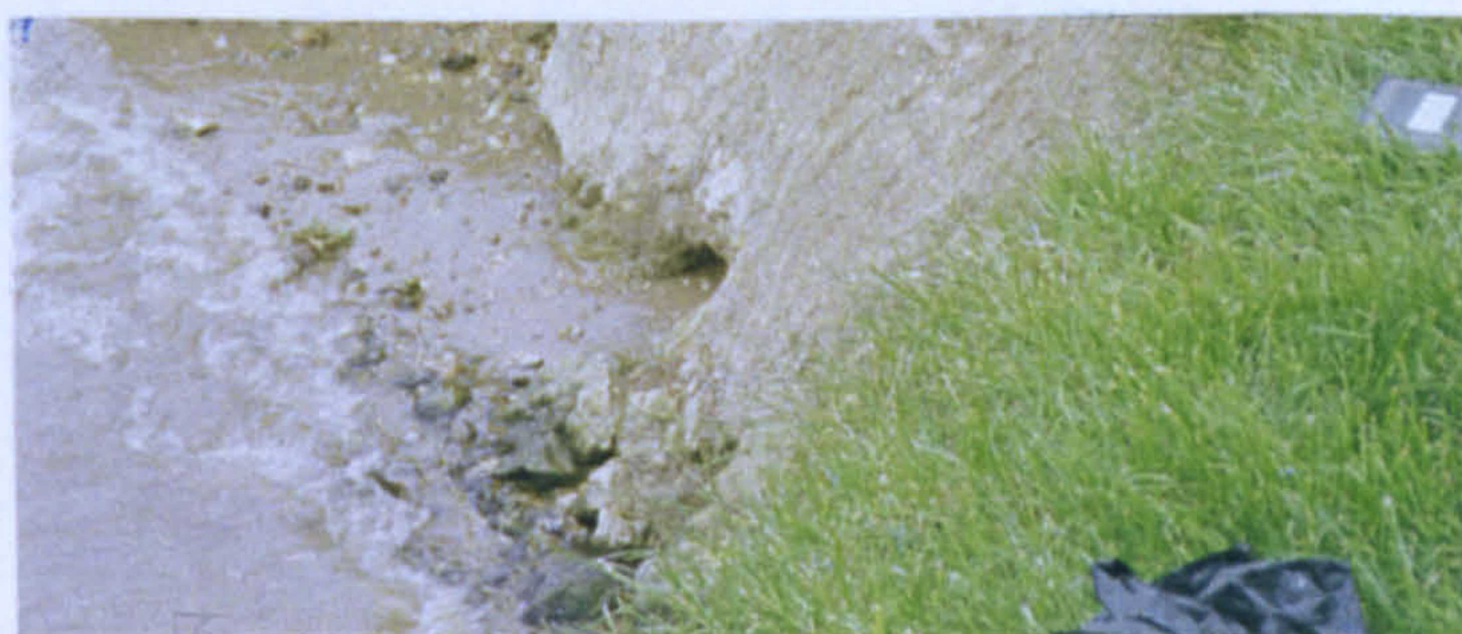
Plate 4.14 Erosion of the clay toe at Lower Wallingford.
