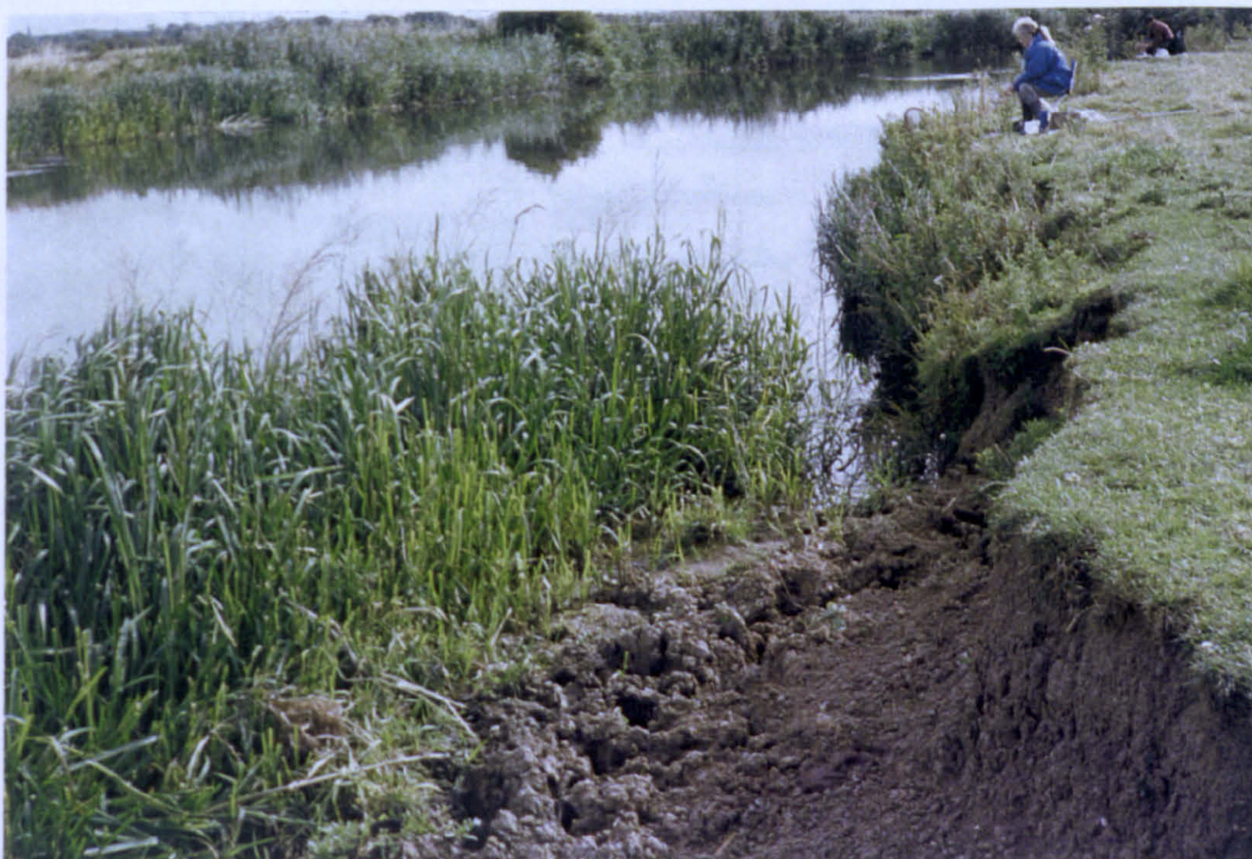
Plate 5.6 Poaching of the river bank downstream of Eynsham Lock (see Bank erosion site no. 36, Map 9, Volume III) .
