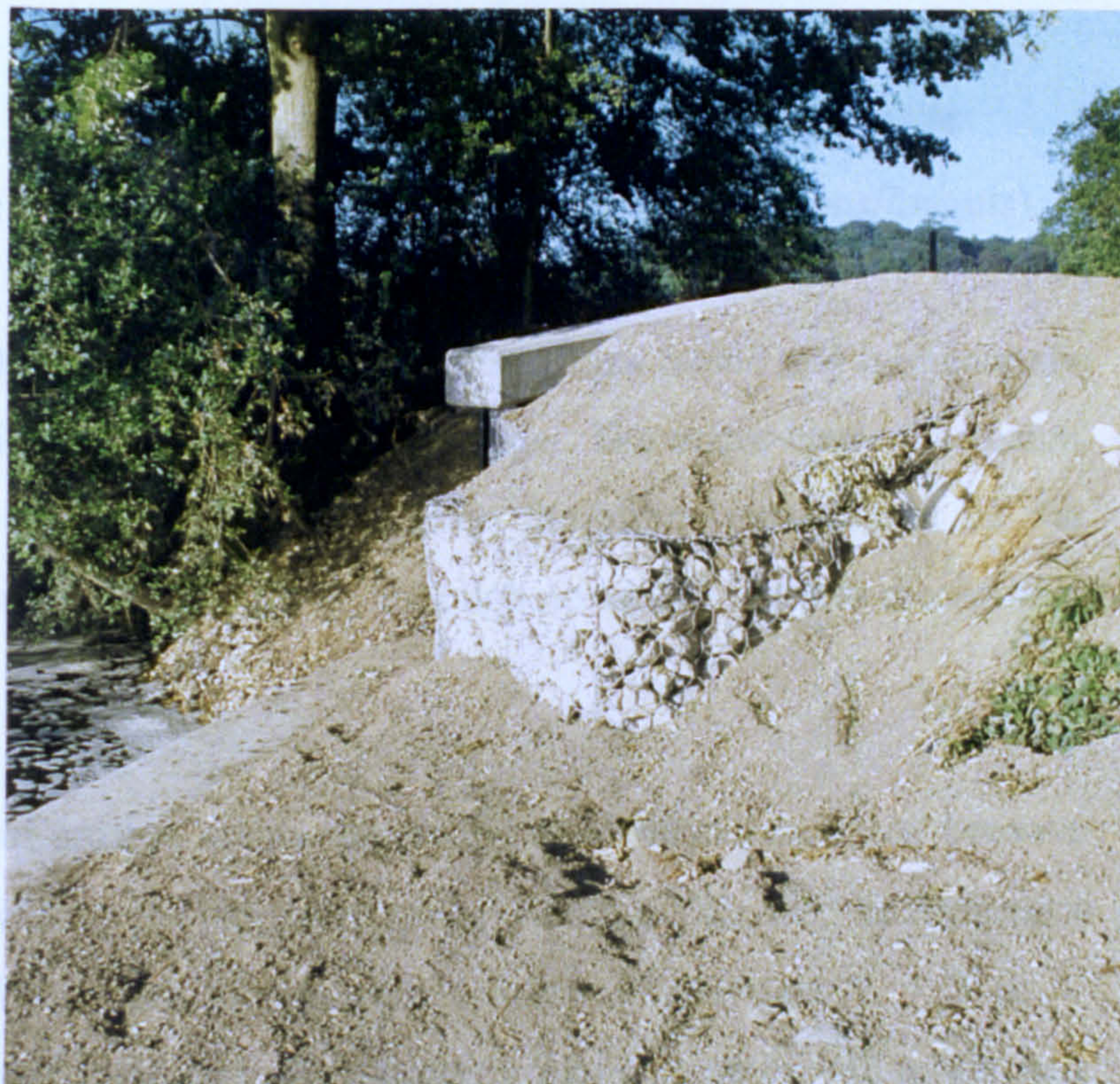
Plate 6.32 Case study no. 17: sheet piling and gabion baskets opposite Cookham Weir (June 1995, after construction)
