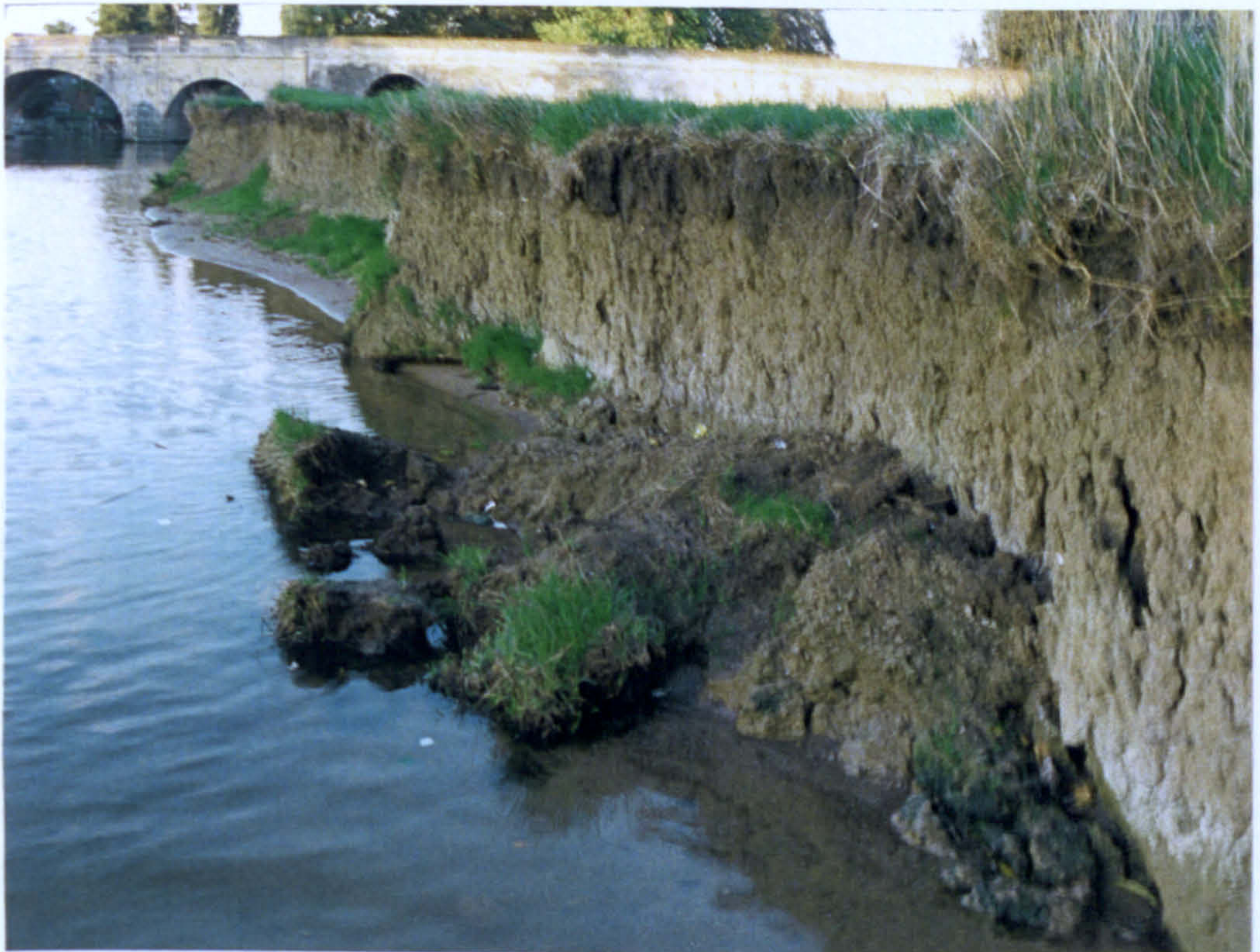
Plate 4.29 Bank failure at Lower Wallingford at the end of summer 1993.
