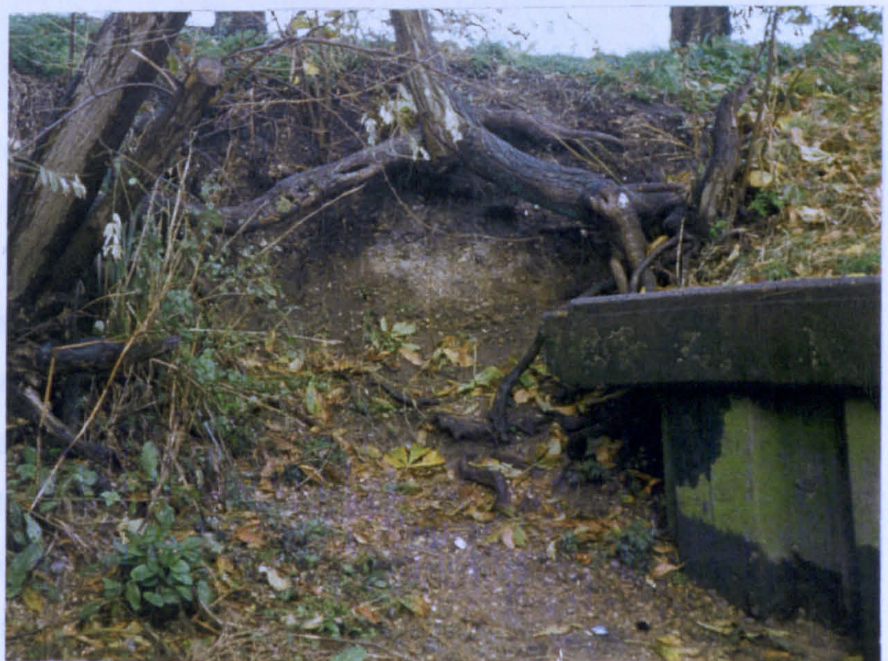
Plate 6.39 Case study no. 21: scour behind sheet piling downstream of Teddington Weir
