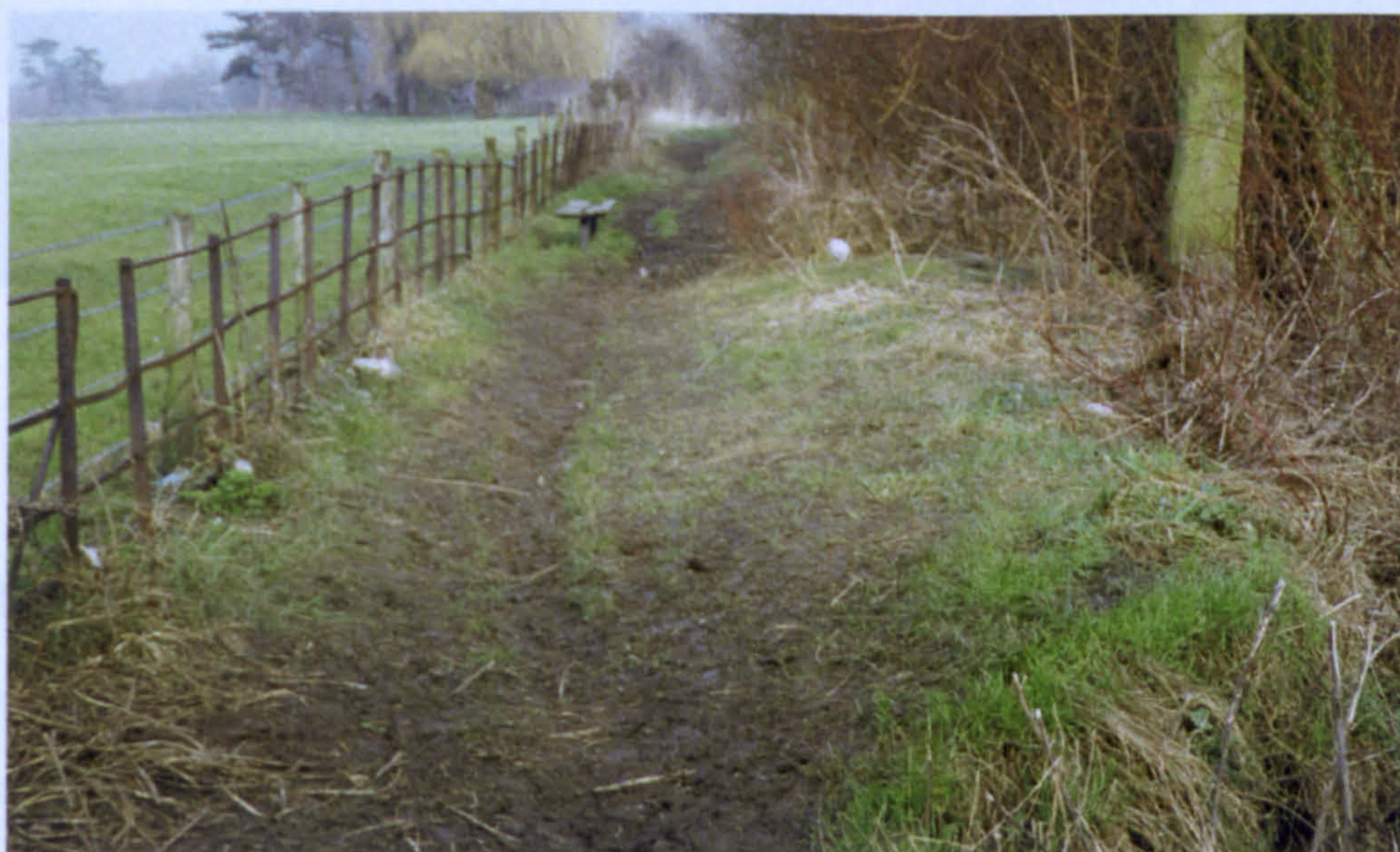
Plate 5.8 Erosion of the surface of the tow path due to pedestrian access, upstream of Wallingford Bridge.
