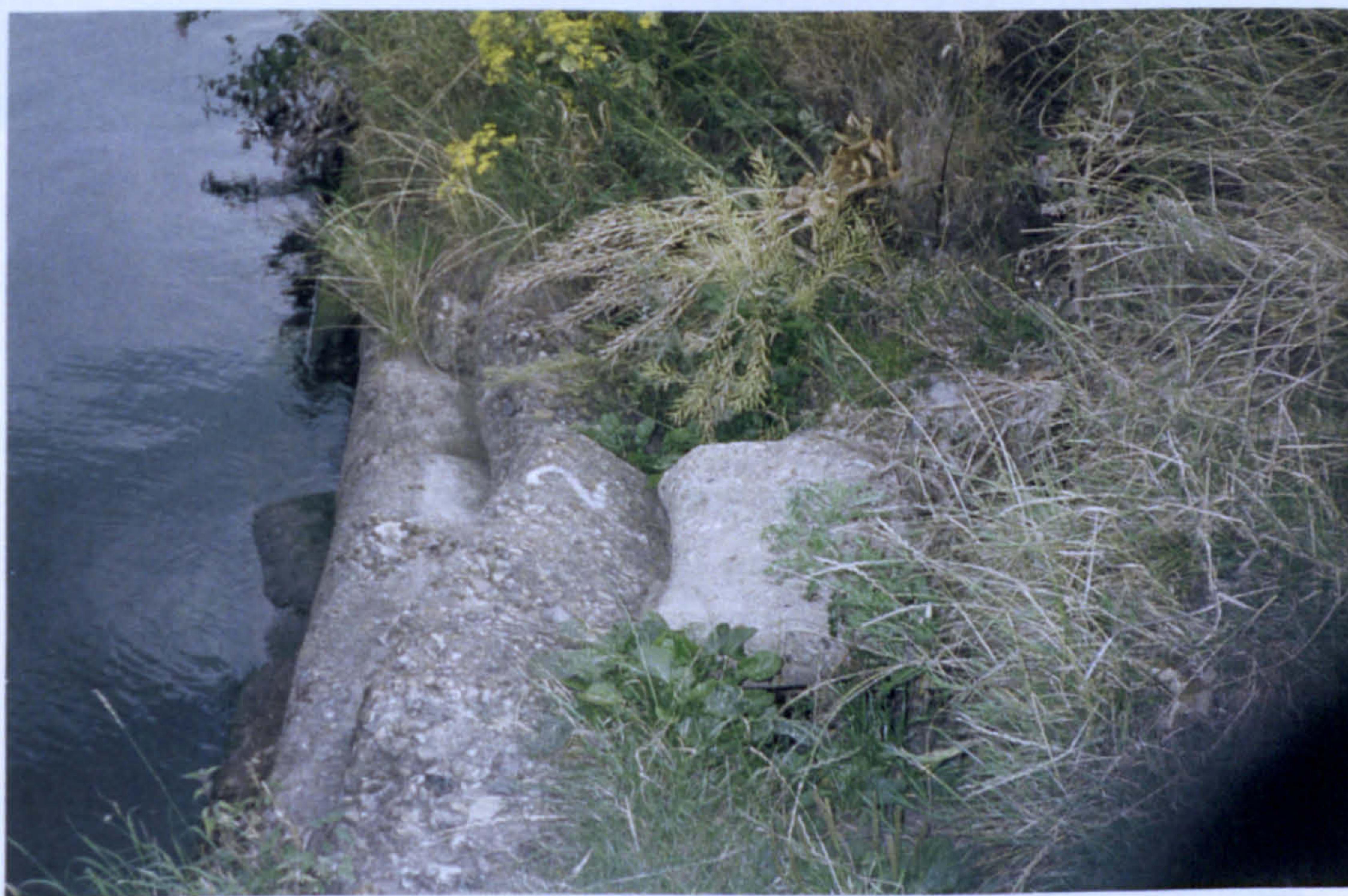
Plate 5.9 Displacement of concrete bagwork at angling swim along Old Windsor Reach (see Bank erosion site no. 127, Map 36, Volume III).
