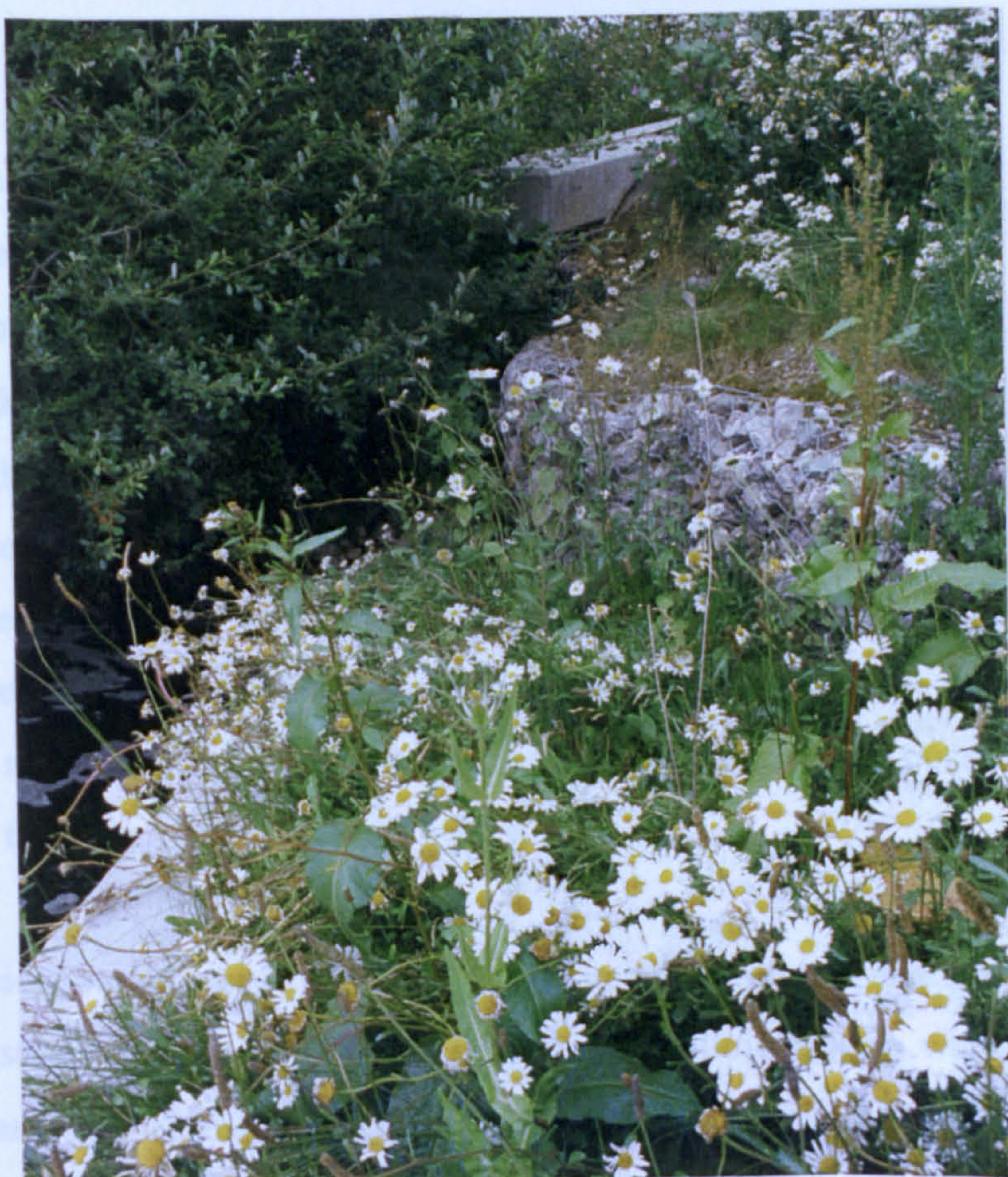
Plate 6.33 Case study no. 17: revegetation of gabion baskets 2 years after installation
