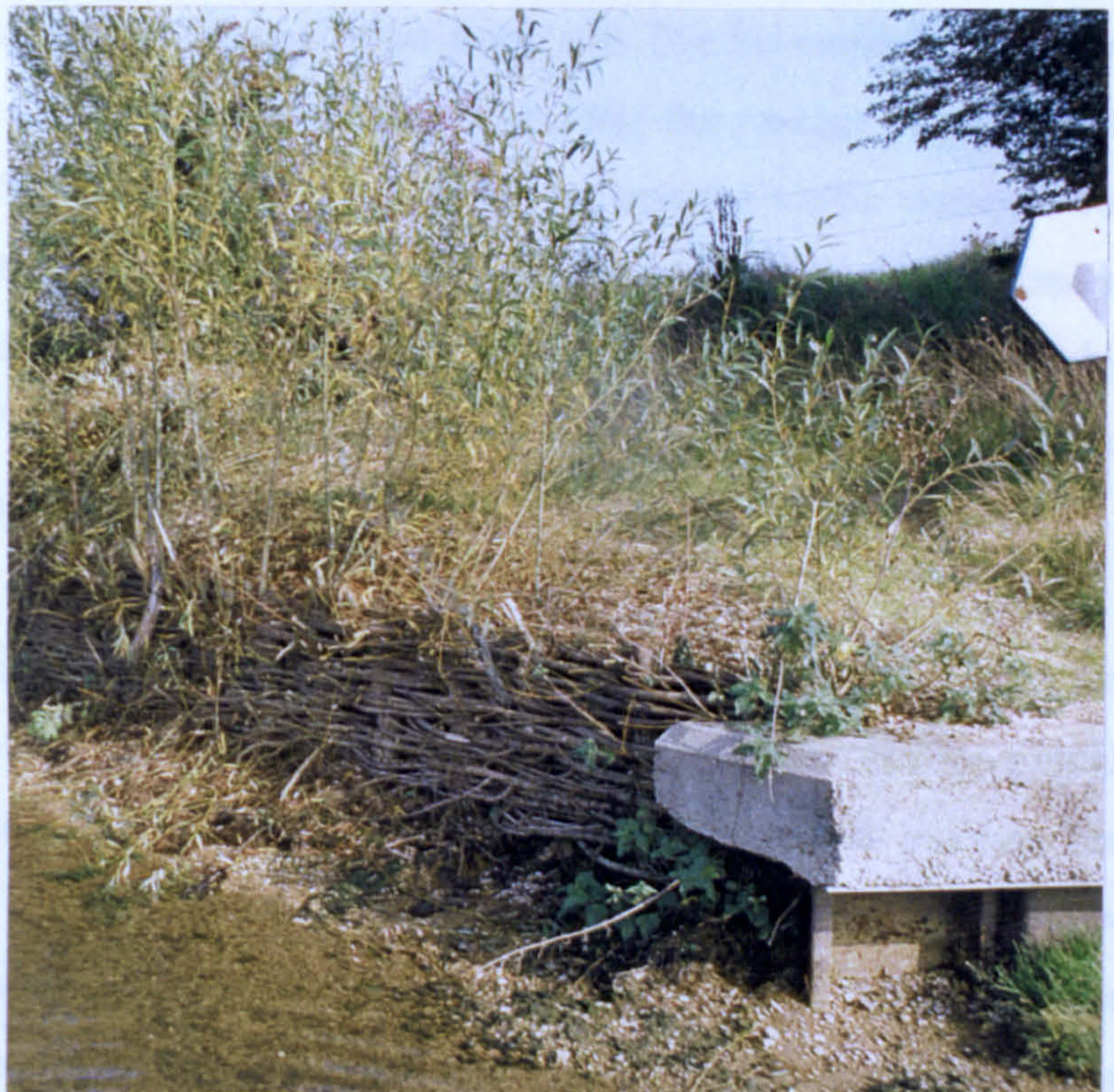
Plate 6.6 Case study no. 6: willow spiling at the entrance to Clifton Lock cut
