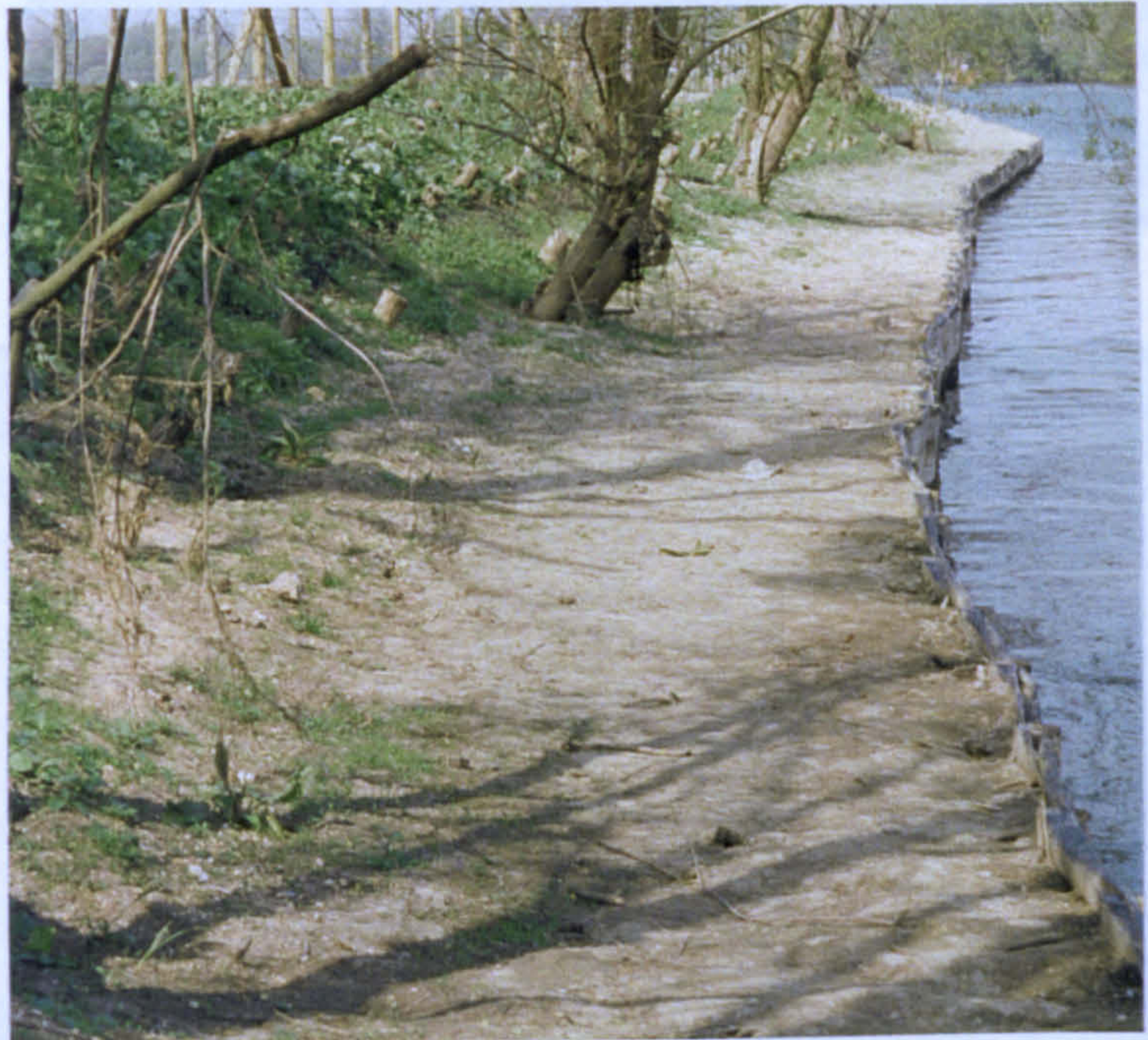
Plate 6.10 Case study no. 8: regraded bank with Nicospan geotextile protecting the lower shelf and willow stakes at the sloping upper bank (May 1995).
