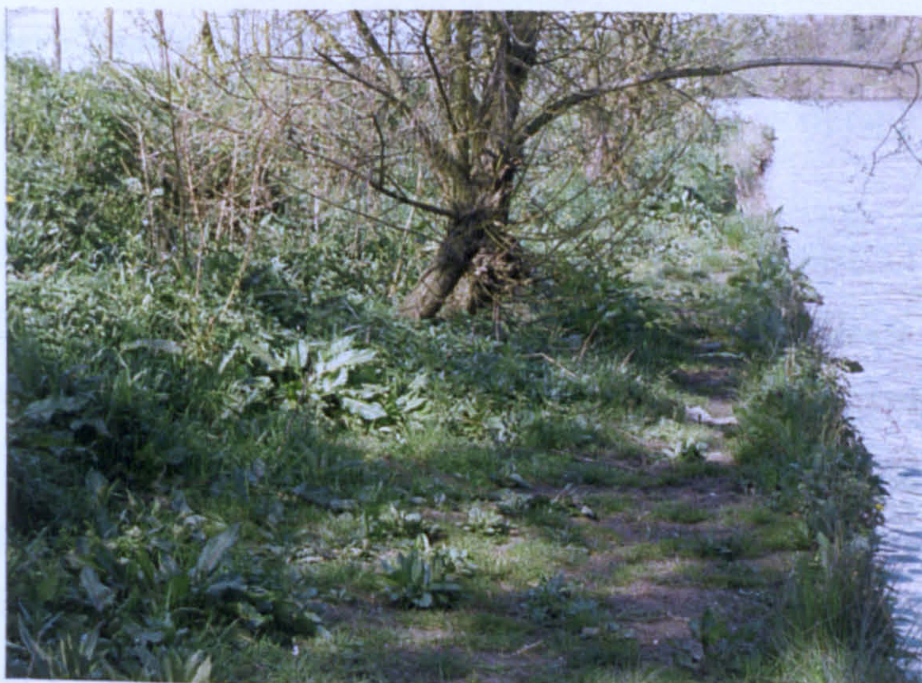
Plate 6.11 Case study no. 8: regraded bank with Nicospan geotextile protecting the lower shelf and willow stakes at the sloping upper bank (May 1996).
