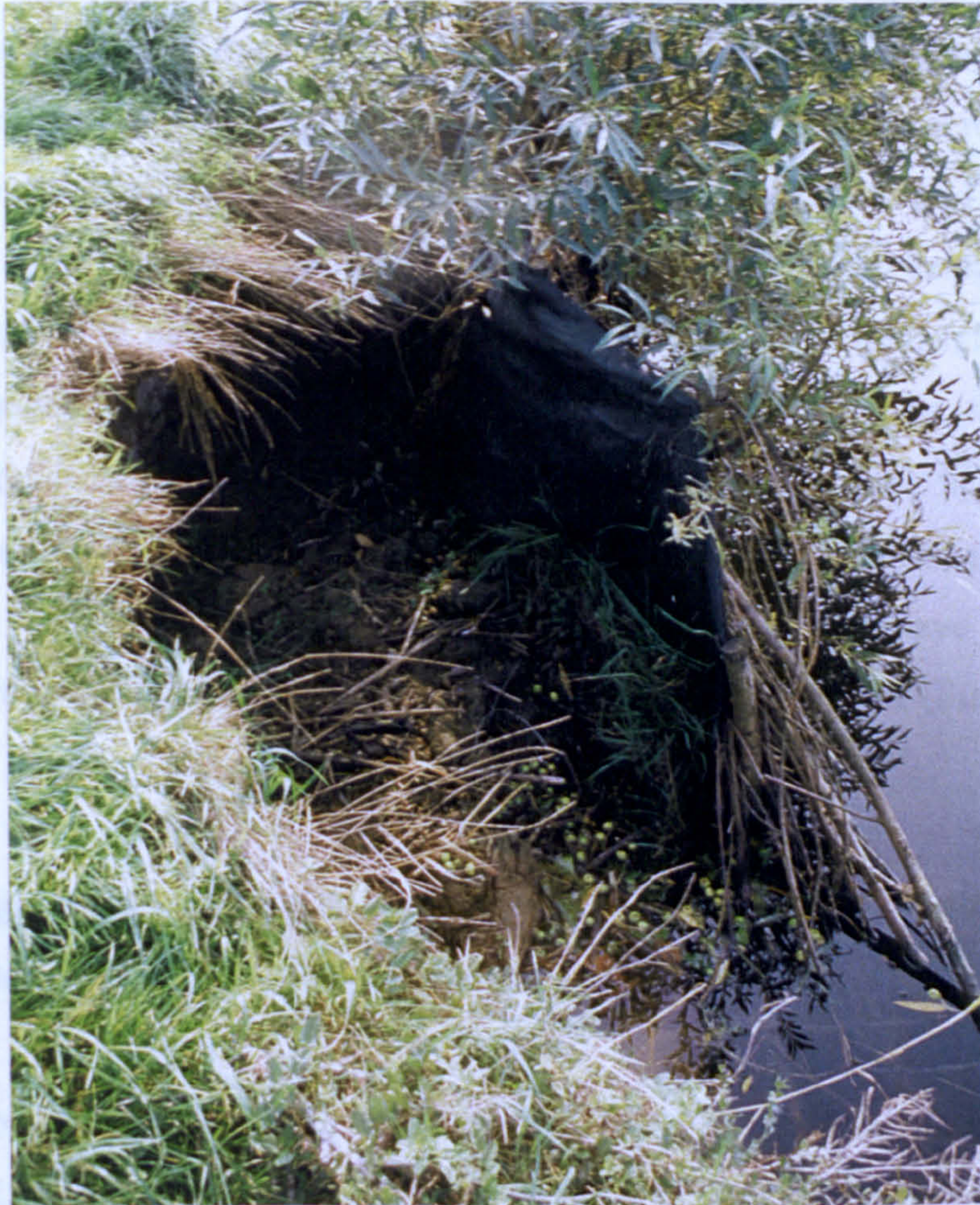
Plate 6.5 Case study no.5: Nicospan geotextile and willow spiling upstream of Clifton Weir
