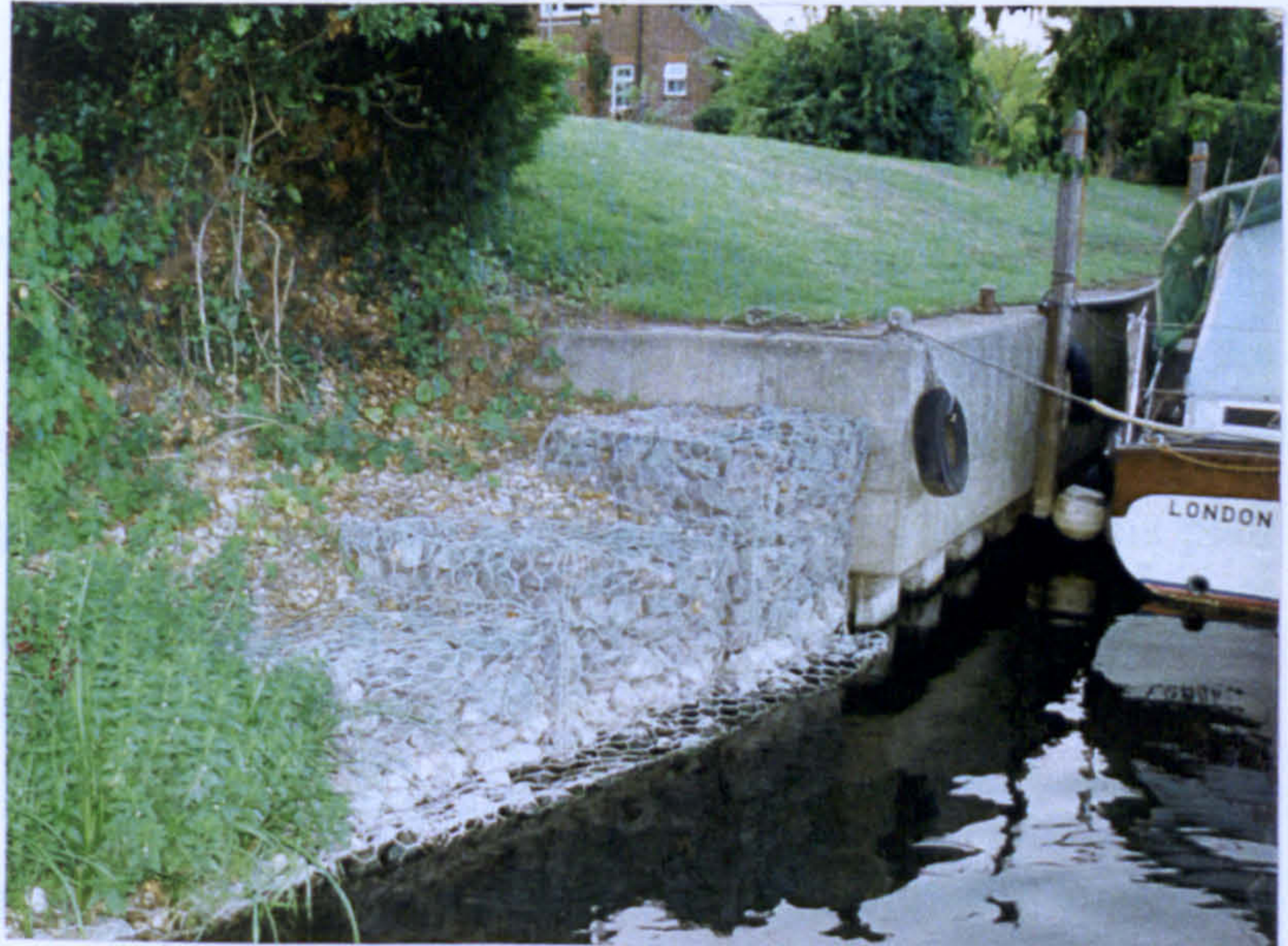
Plate 6.34 Case study no. 18: gabion baskets installed along Egham Reach
