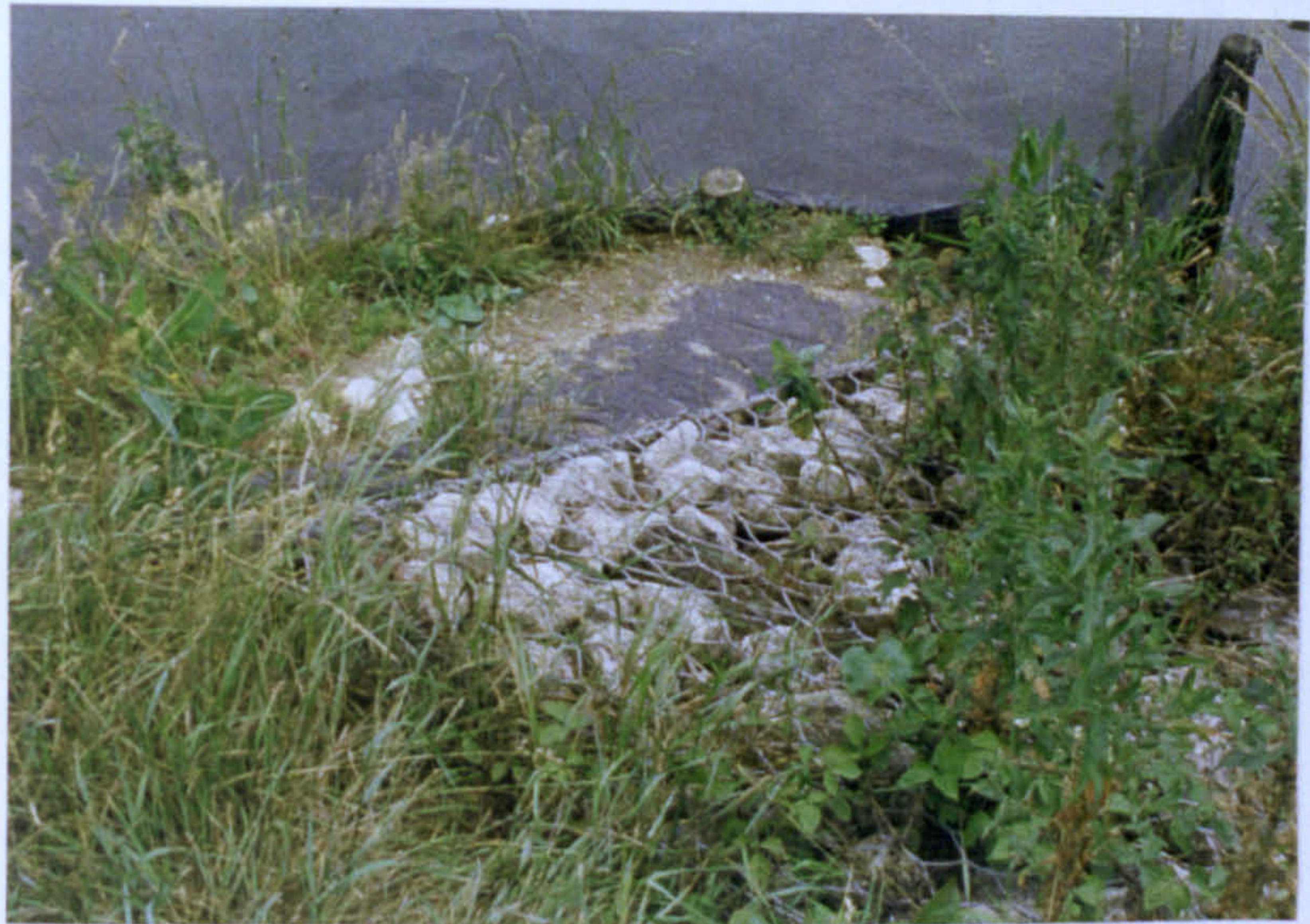
Plate 6.14 Case study no. 9: exposed geotextile underlay where riprap had been placed (June 1997)
