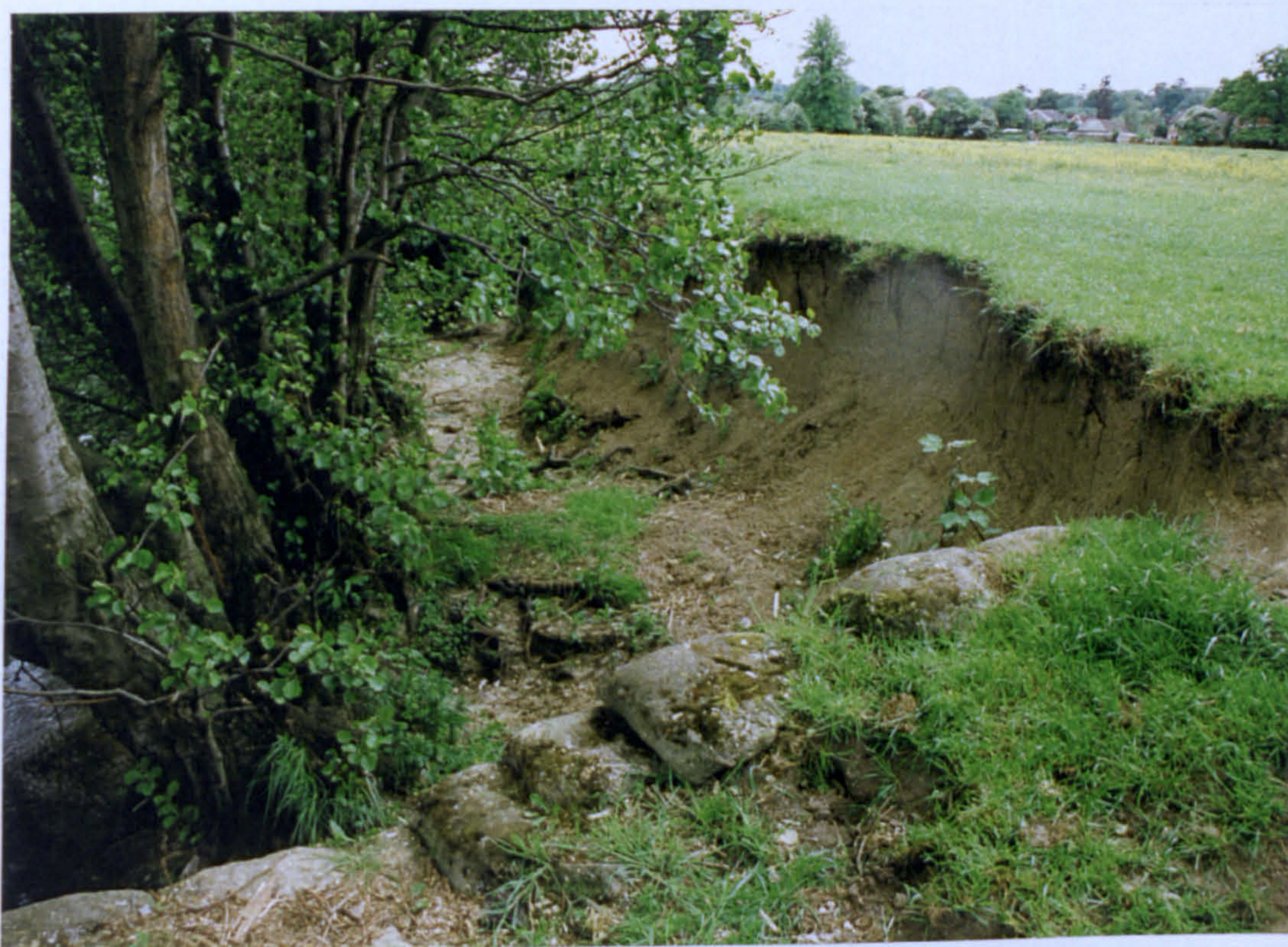
Plate 6.20 Case study no. 12: erosion downstream of Mapledurham Lock prior to bank protection
