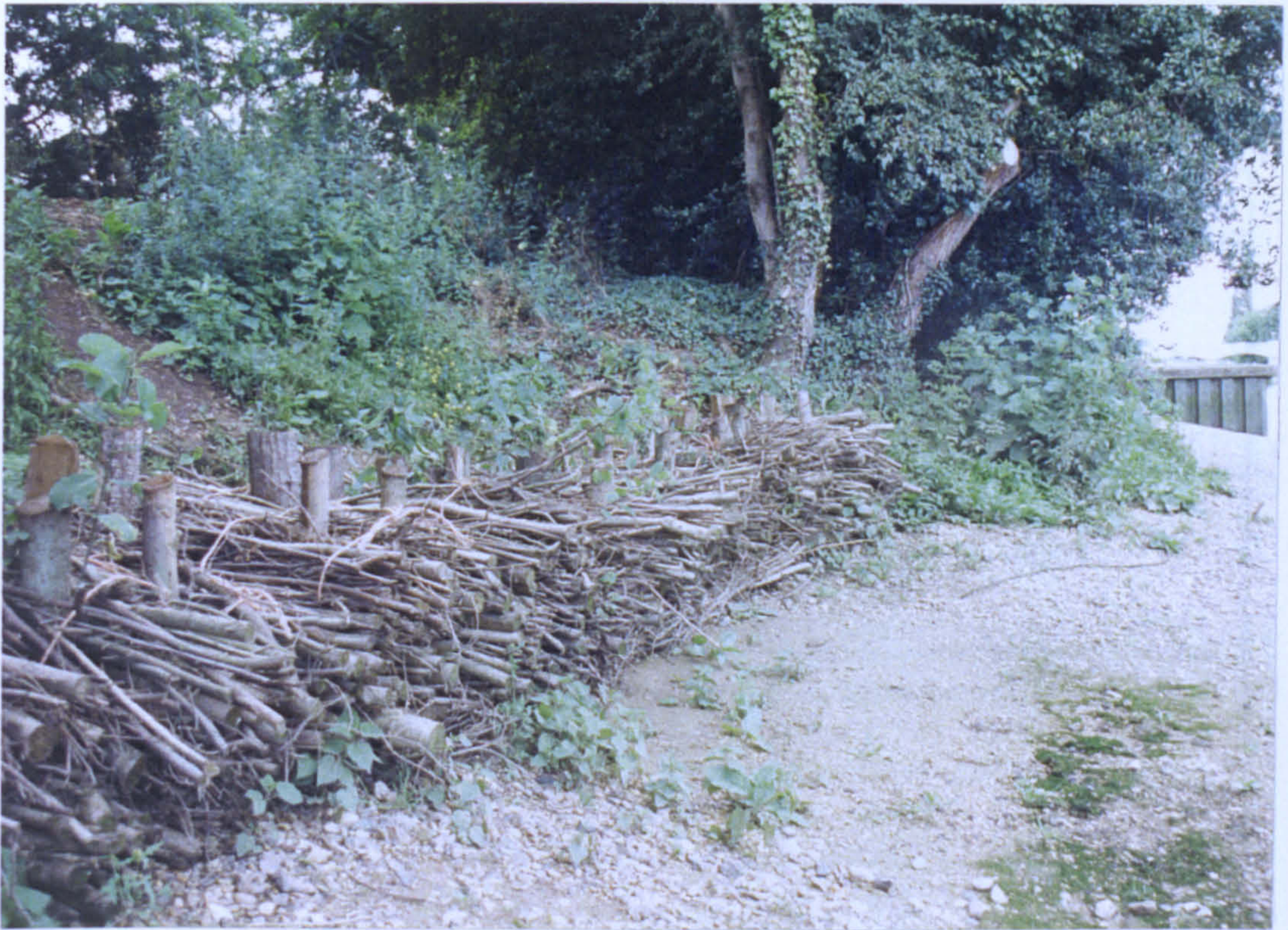
Plate 6.41 Case study no. 21: faggots installed downstream of Teddington Weir
