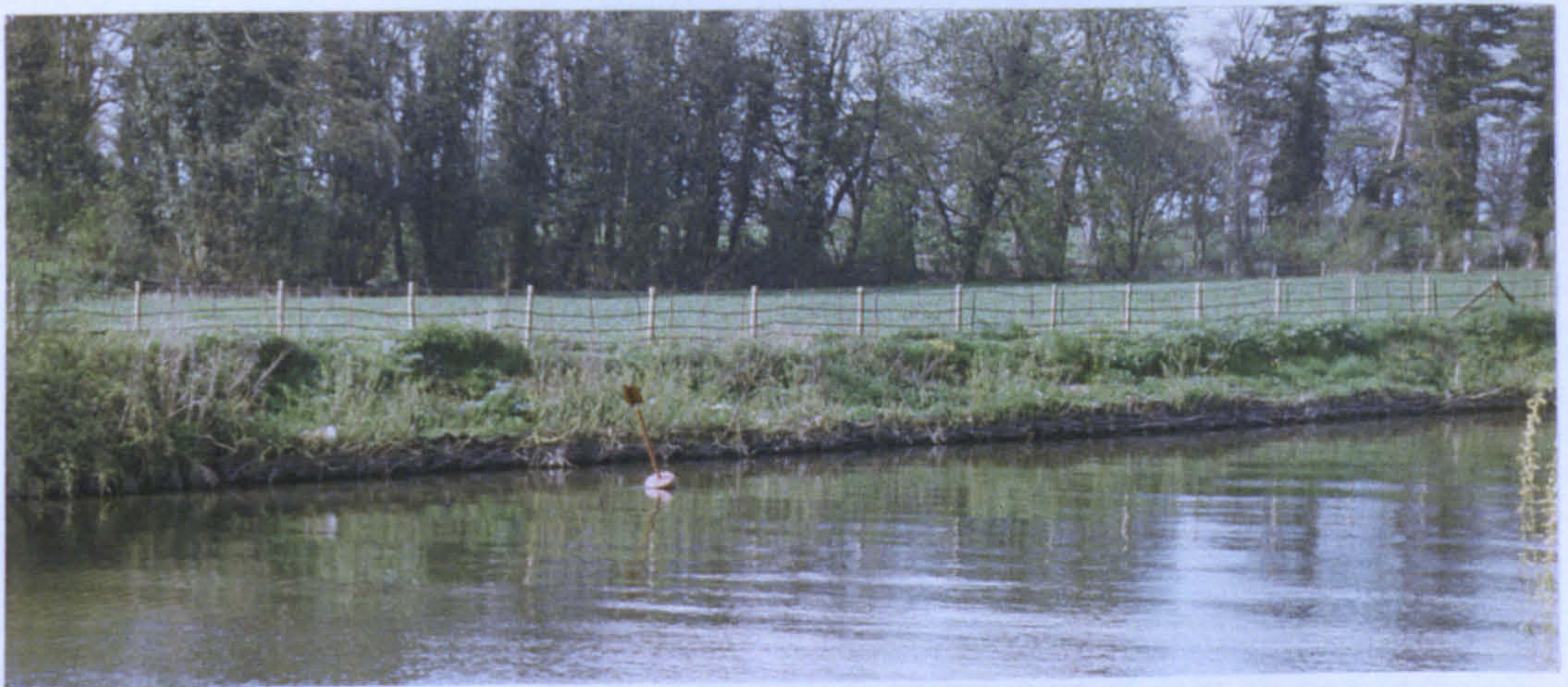
Plate 6.9 Case study no. 8: willow spiling protection along regraded bank, May 1996
