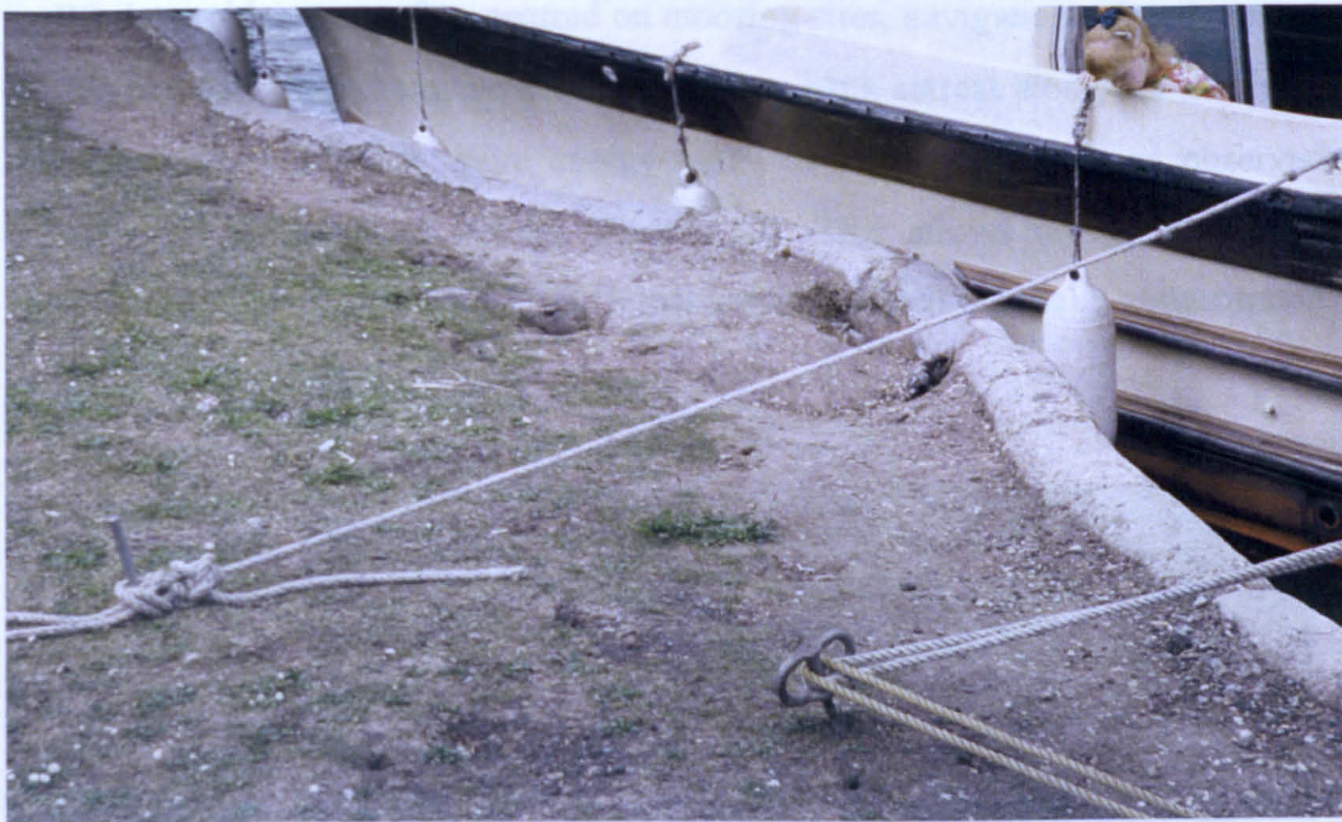
Plate 5.10 Damage of the river bank resulting from the use of mooring pegs at Deadwater Ait, Romney Reach (see Bank erosion site no. 124, Map 35, Volume III)
