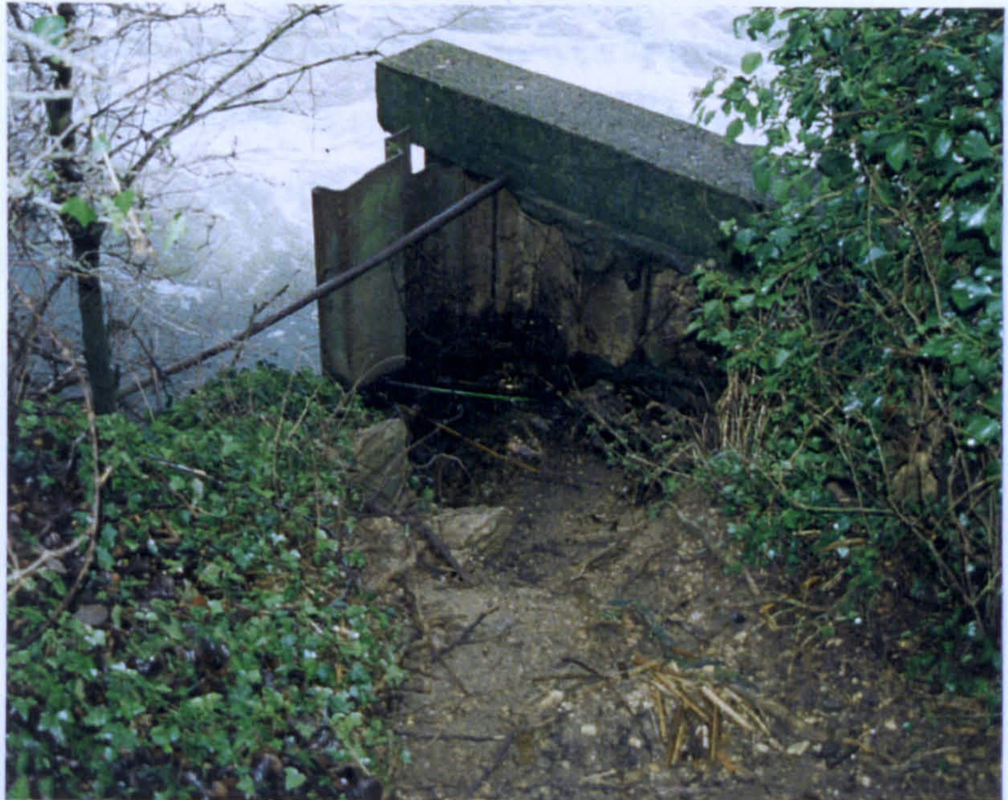
Plate 6.4 Case study no. 4: erosion of the upper bank downstream of Culham Weir
