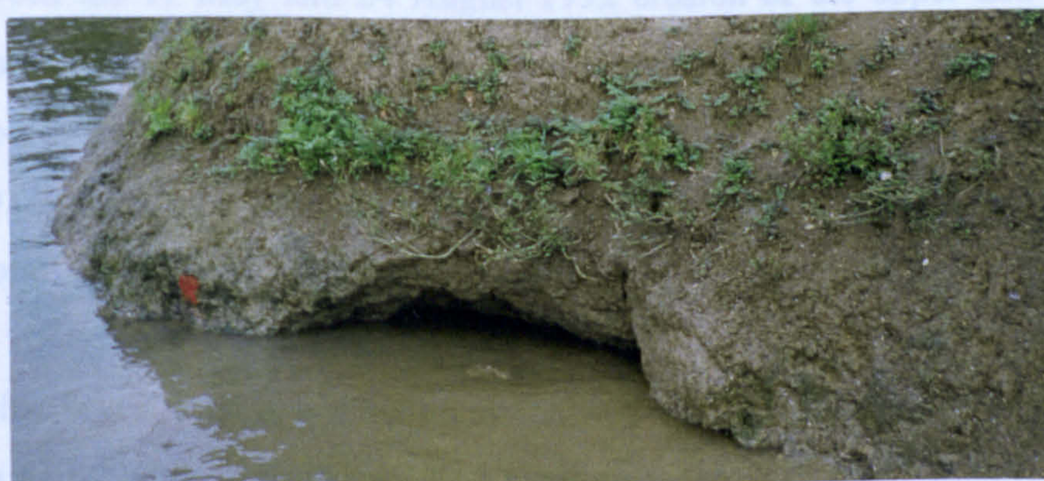
Plate 4.12 Undercutting at the toe of the bank at profile four.
