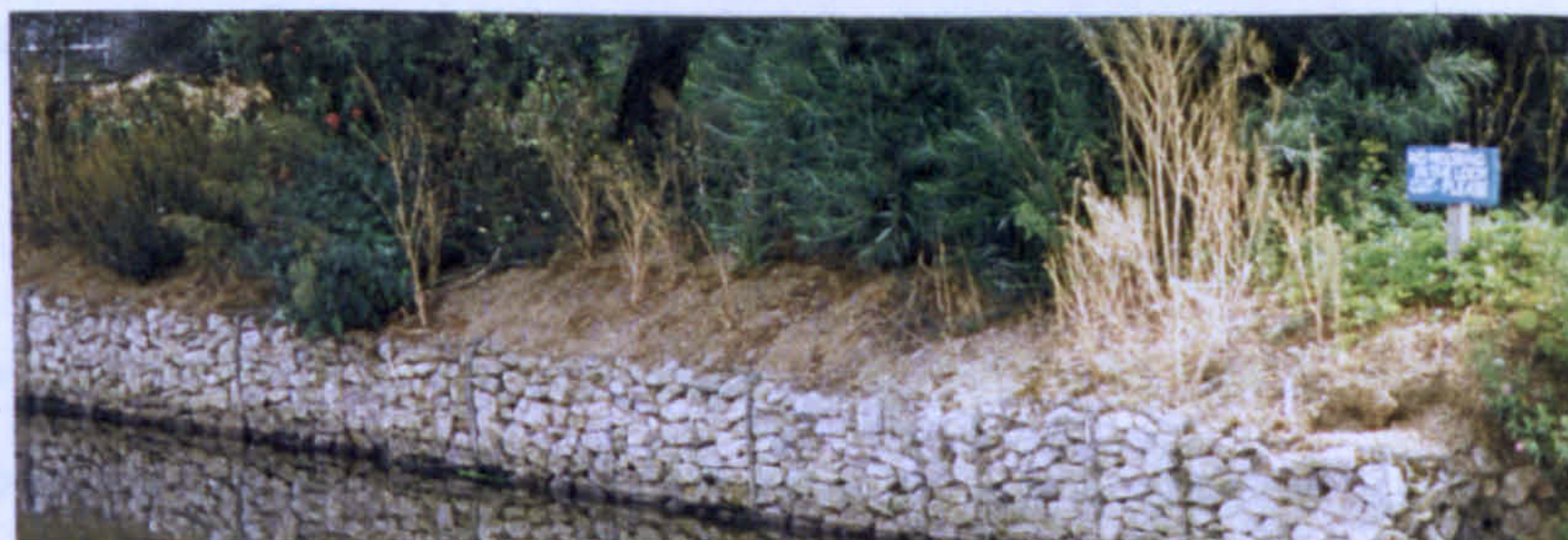
Plate 6.2 Case study no. 2: gabion baskets at Godstow lock island
