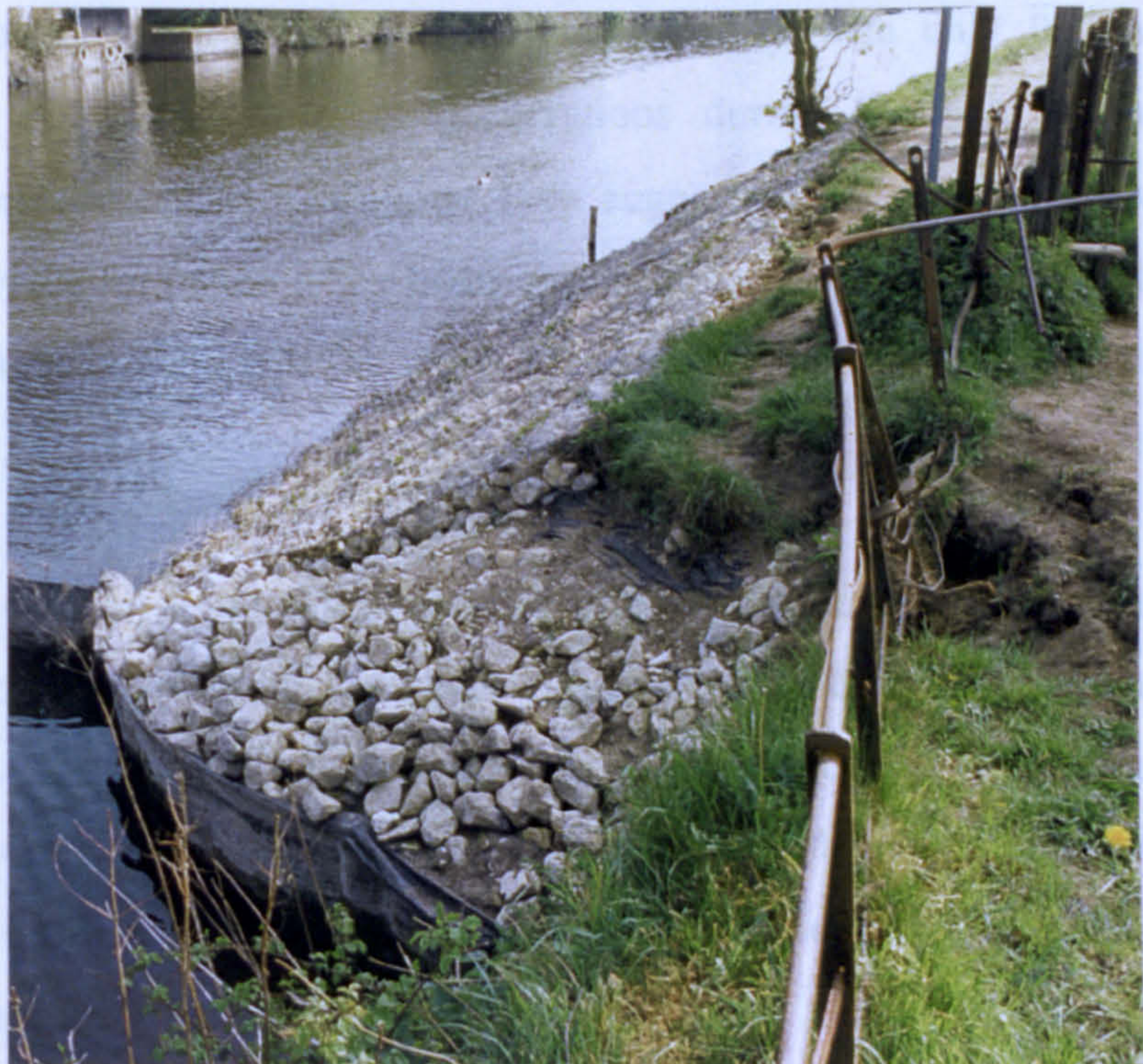
Plate 6.13 Case study no. 9: gabion mattress and riprap protection upstream of Wallingford Bridge (taken May 1995)
