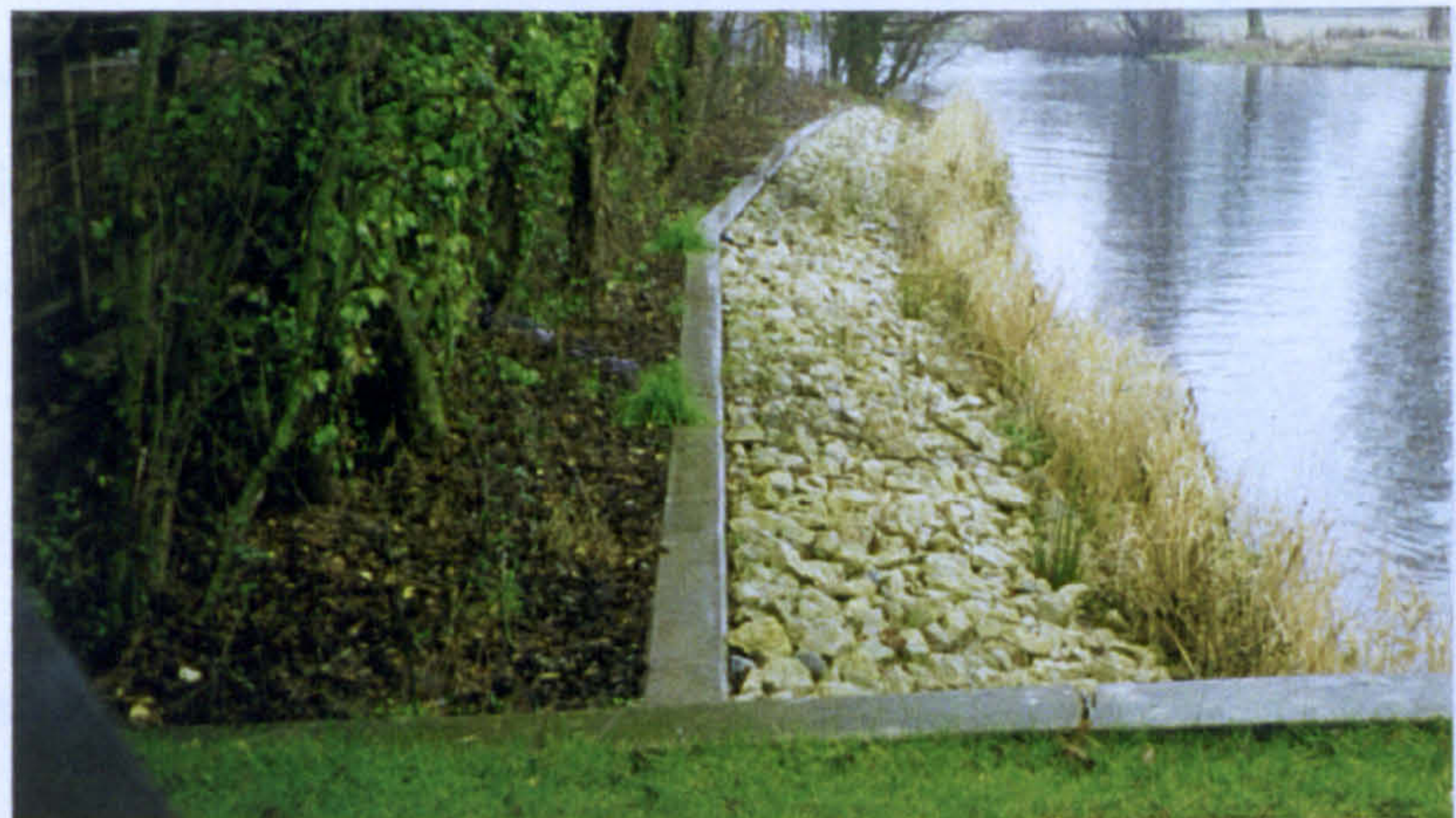
Plate 6.3 Case study no. 3: sheet piling below water level with riprap and reed planting (taken December 1996)
