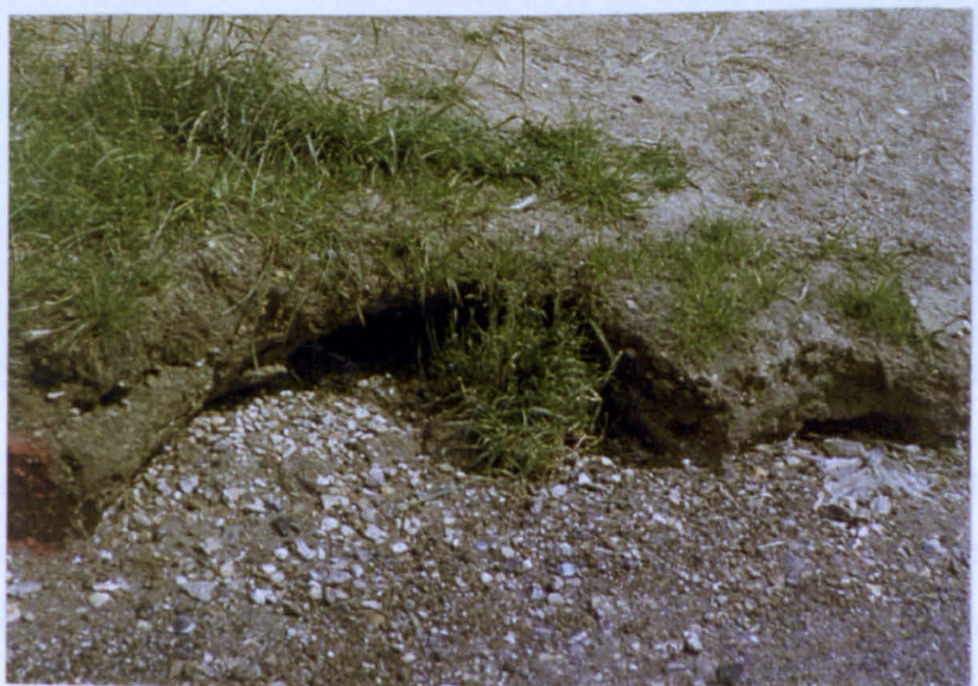
Plate 4.11 Undercutting at the toe of the bank at profile three.
