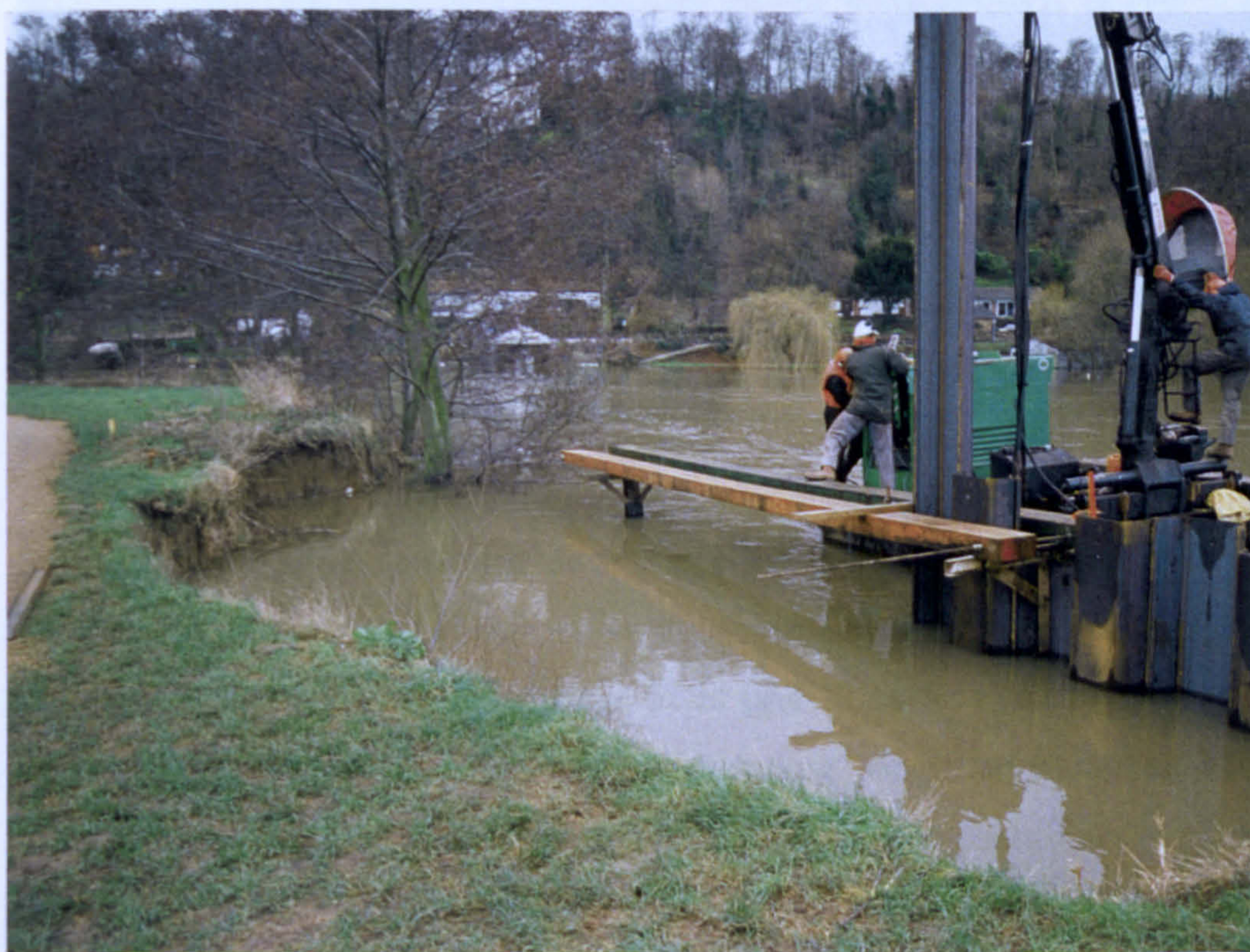
Plate 5.3 Installation of sheet piling to protect the eroding cliff face at Marlow (see also Erosion control case study no. 15: Plate 6.15, Map 31, Volume III)
