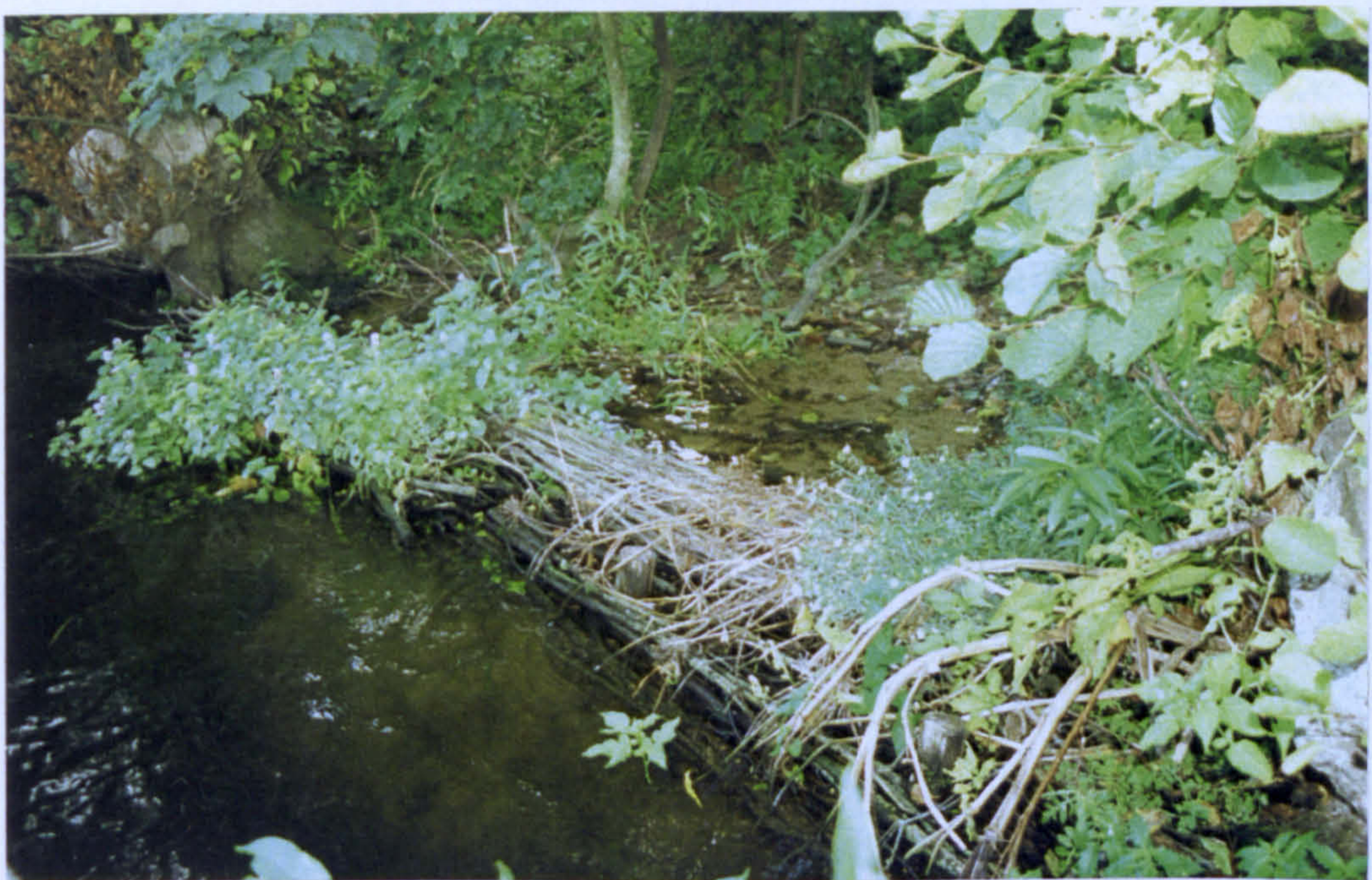
Plate 6.21 Case study no. 12: faggot bank protection downstream of Mapledurham Lock
