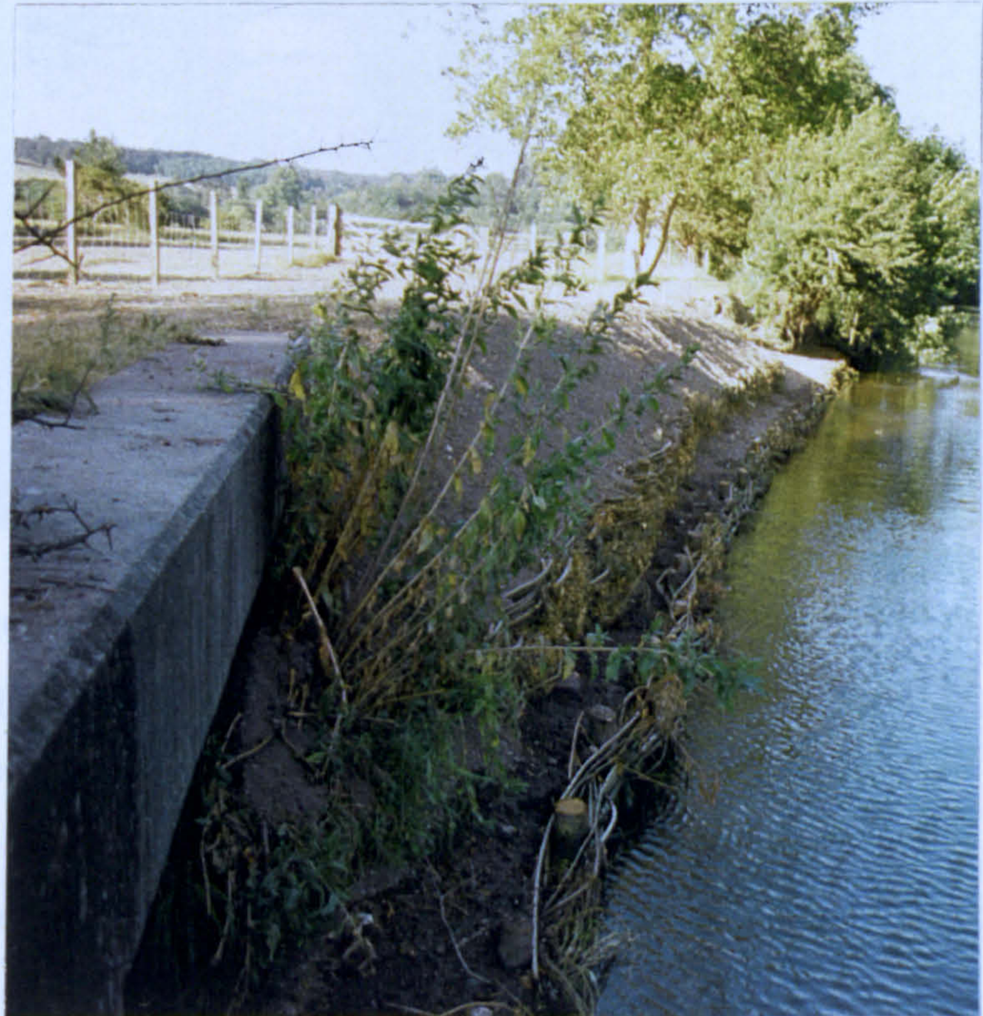
Plate 6.30 Case study no. 16: willow spiling along Cookham Lock Cut
