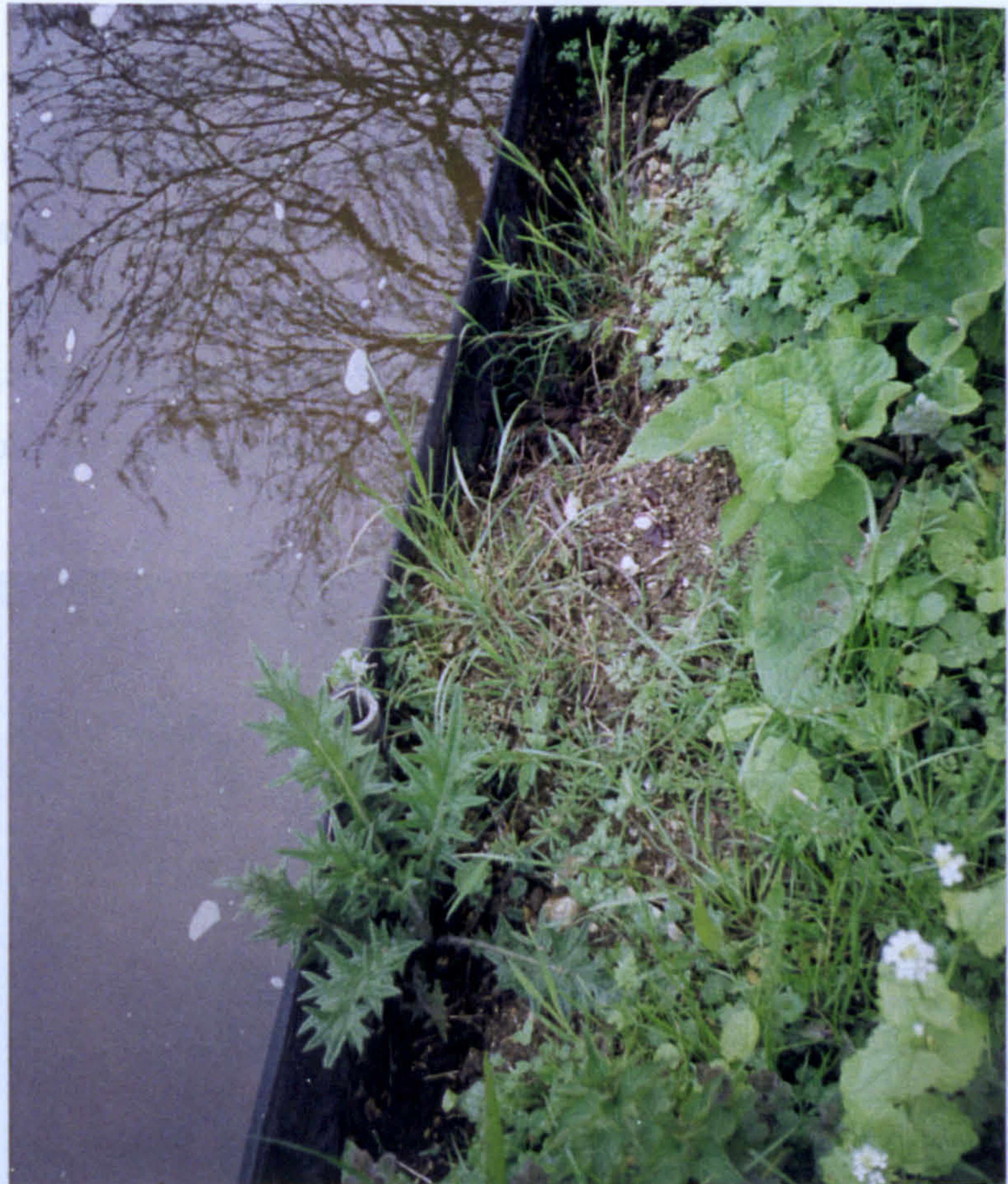
Plate 6.17 Case study no. 10: wash out of backfill behind Nicospan geotextile along Goring Reach
