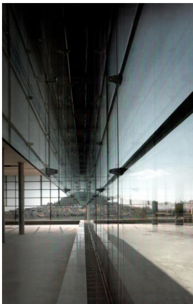
Figure 5.50 Detail of double-glass façade (Source: Tschumi, B. New Acropolis Museum , 2009, p. 117.)
