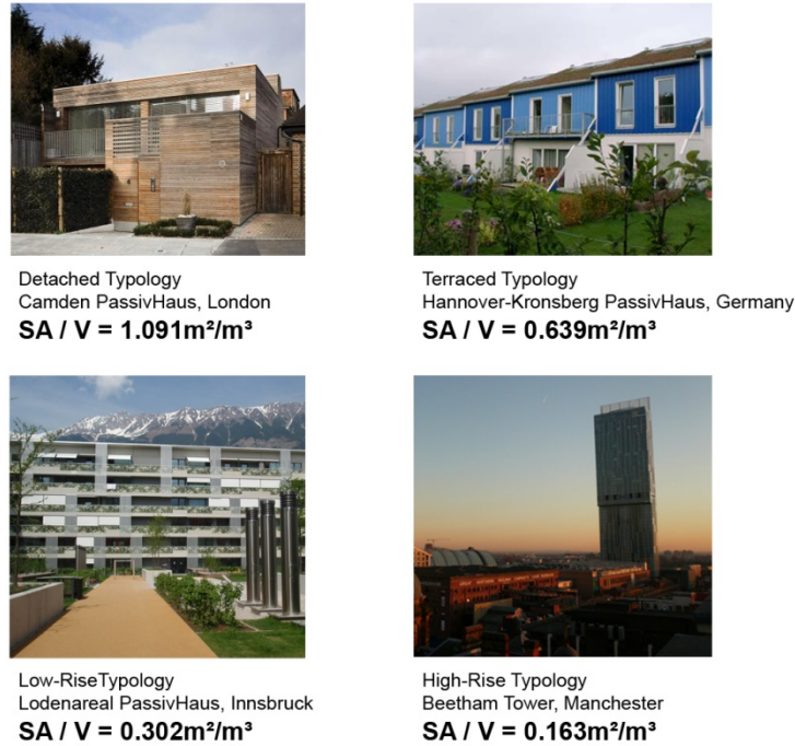
Figure 5: Surface area to volume ratios of the four different typologies (Source: author)
