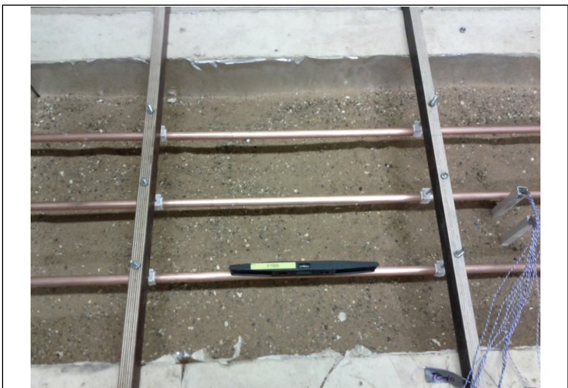
Figure 5-7 Supporting and levelling the collector pipes
