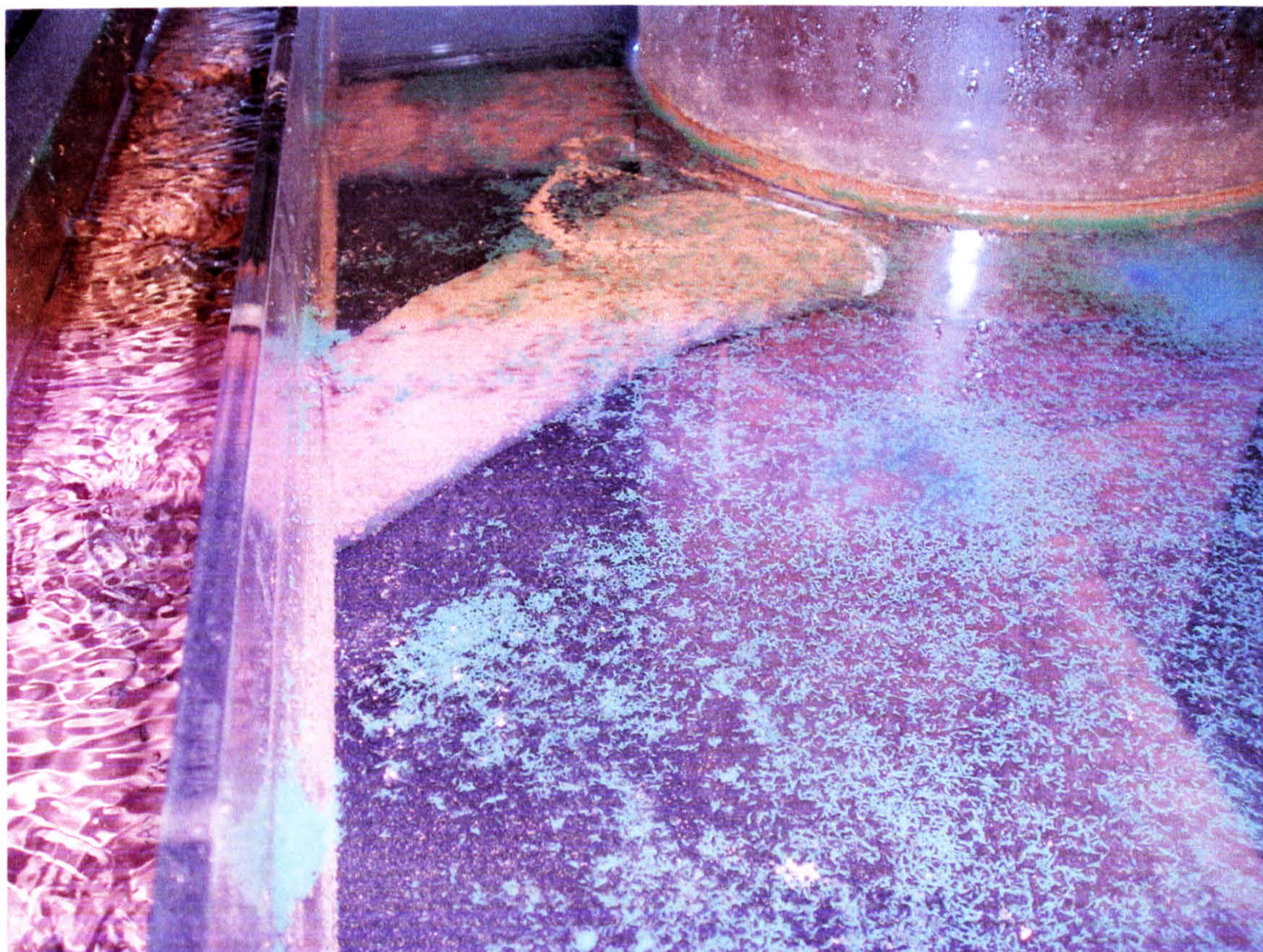
Fig 8.6 Algae growth in the MIEX settling tank
