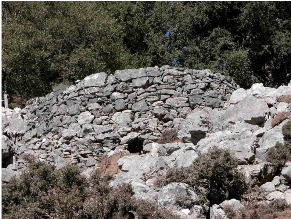
Figure 8.11: Stone construction for cheese maturation. The small entrance (no more than a metre high) is characteristic and keeps temperature stable for cheese storage.
