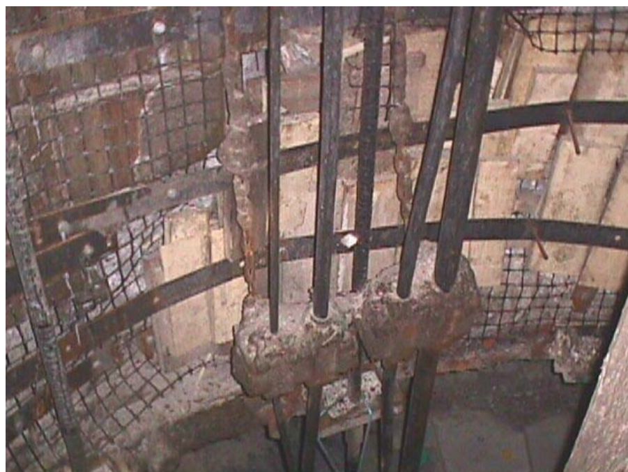
Figure 2.13 Damaged manshaft before the second relining (Williams and Auld 2002)
