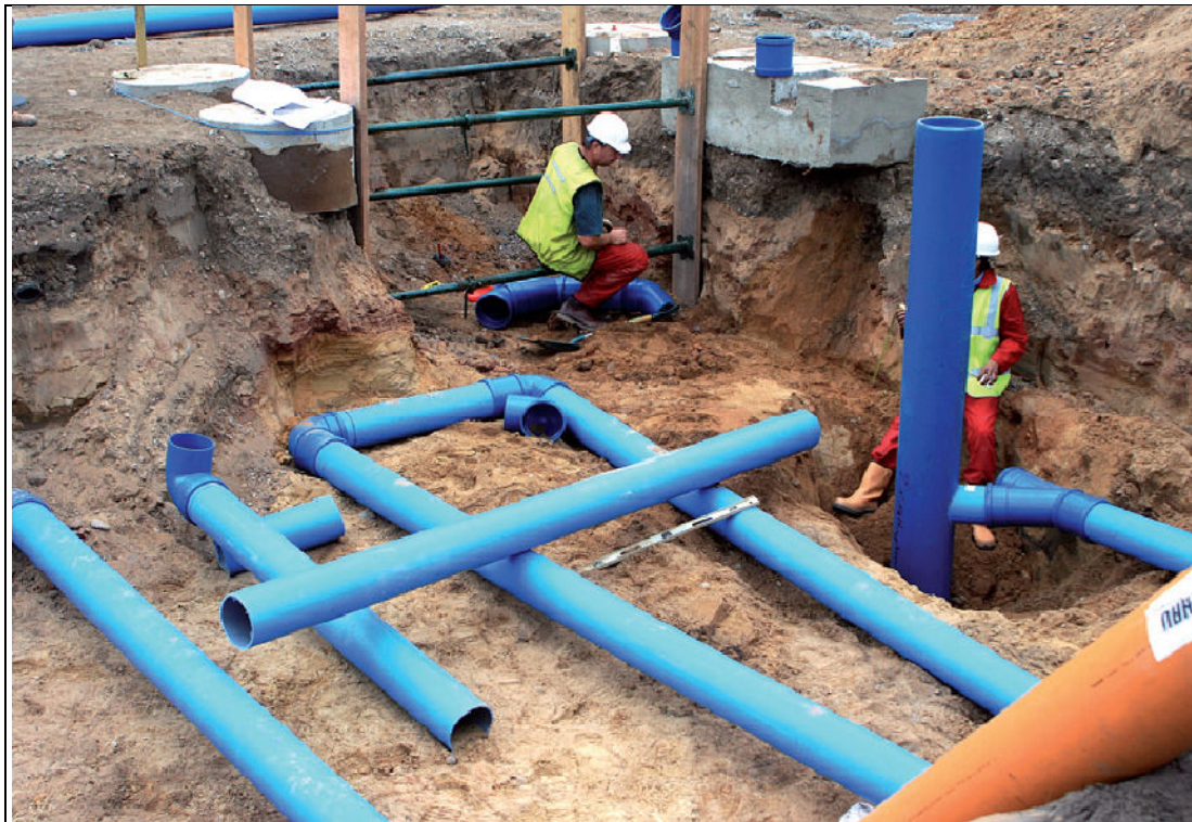
Figure 7-16: The installation of the Awadukt EAHE in the BASF house plot
