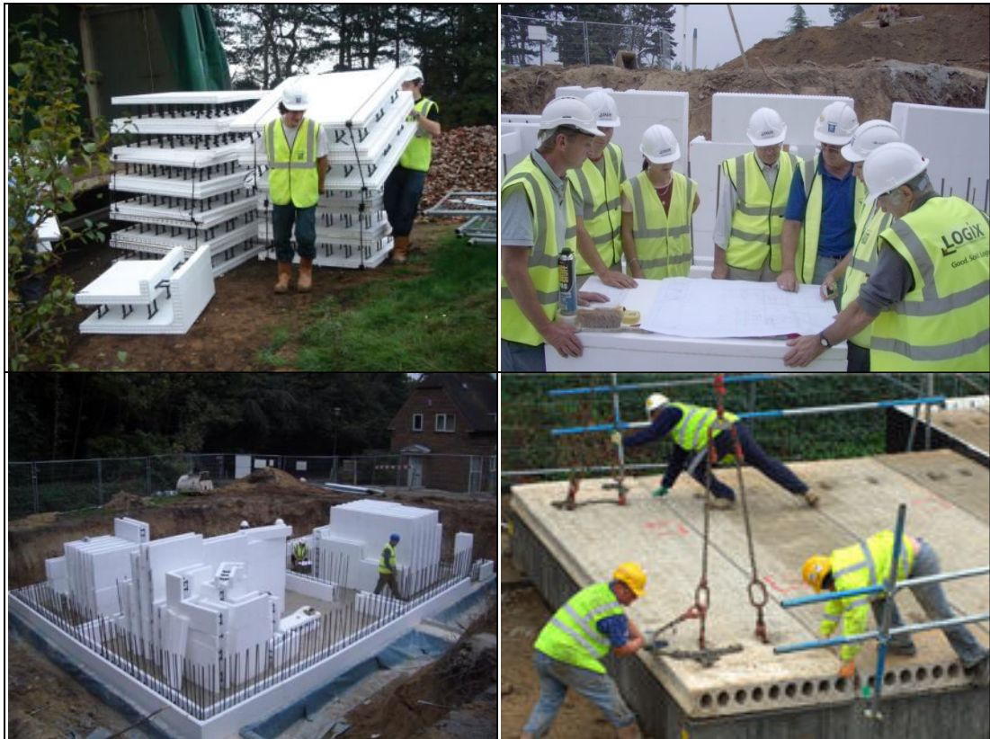
Figure 6-5: The construction of the Stoneguard house basement with help of undergraduate students of architecture (pictures by the author and by the photographer Robert Paulden)
