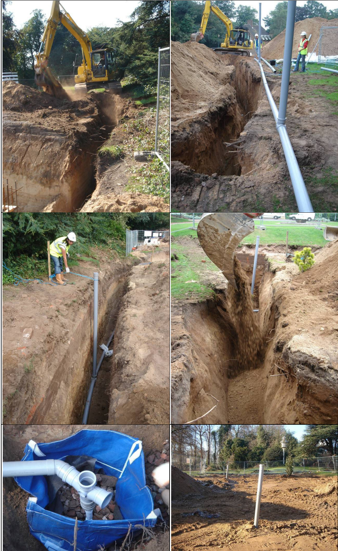
Figure 6-18: The construction of the Stoneguard House EAHE
