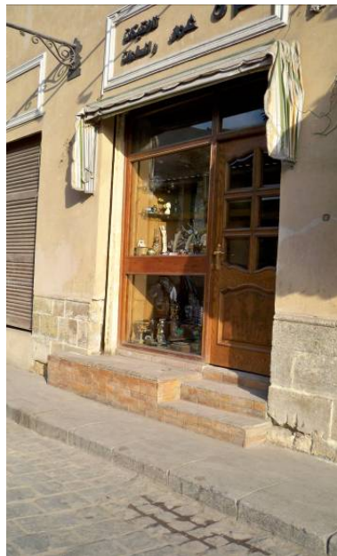
FIGURE 6.19: THE STREET LOWERING CAUSED A HEIGHT DIFFERENCE BETWEEN THE SHOPS AND STREET LEVEL.
