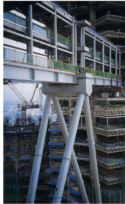
1996. Petronas Towers Skybridge , Kuala Lumpur; (a) View of towers showing skybridge connecting at 41 st & 42 nd floor (source: author), (b) Lift zoning sketch diagram, showing 'skylobby' elevator change-over at 41 st & 42 nd floor levels (source: Pelli & Crosbie, 2001, p.114), (c) Double deck nature of skybridge (source: Pelli & Crosbie, 2001, p.54)
