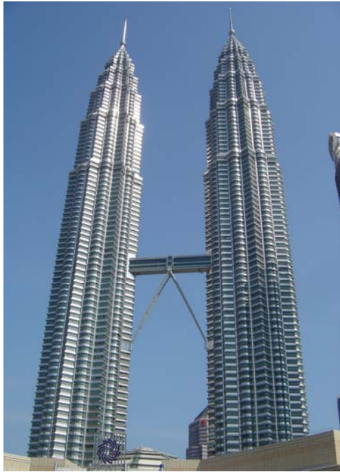
1996. Petronas Towers Skybridge , Kuala Lumpur; (a) View of towers showing skybridge connecting at 41 st & 42 nd floor (source: author), (b) Lift zoning sketch diagram, showing 'skylobby' elevator change-over at 41 st & 42 nd floor levels (source: Pelli & Crosbie, 2001, p.114), (c) Double deck nature of skybridge (source: Pelli & Crosbie, 2001, p.54)
