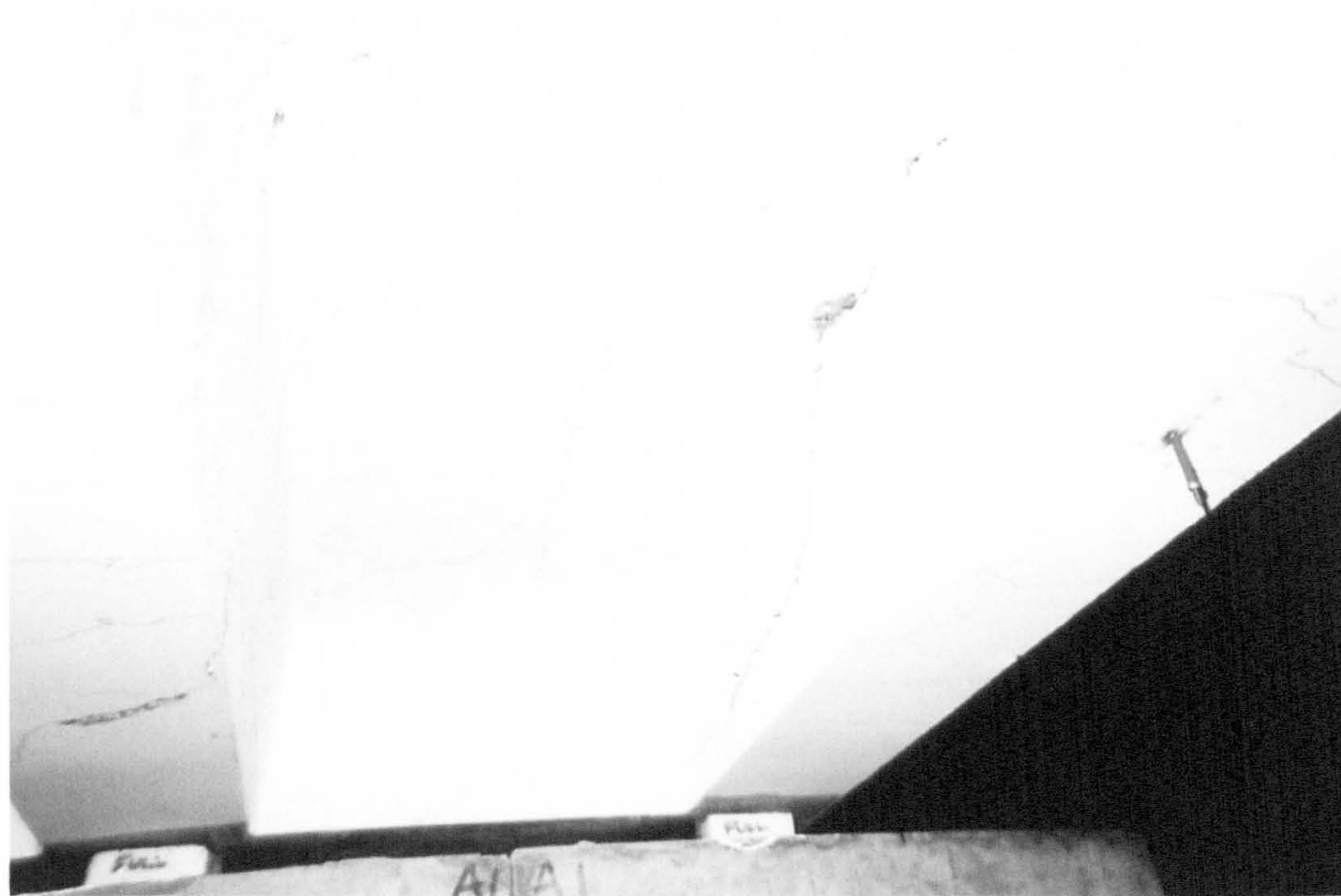
Plate 4-15: Deck 5 loading and cracking
